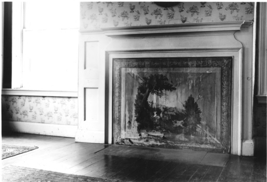
Wooden mantel in left side front room on second floor of the mansion house at "Lindenwald." Photo taken 8-3-36.
