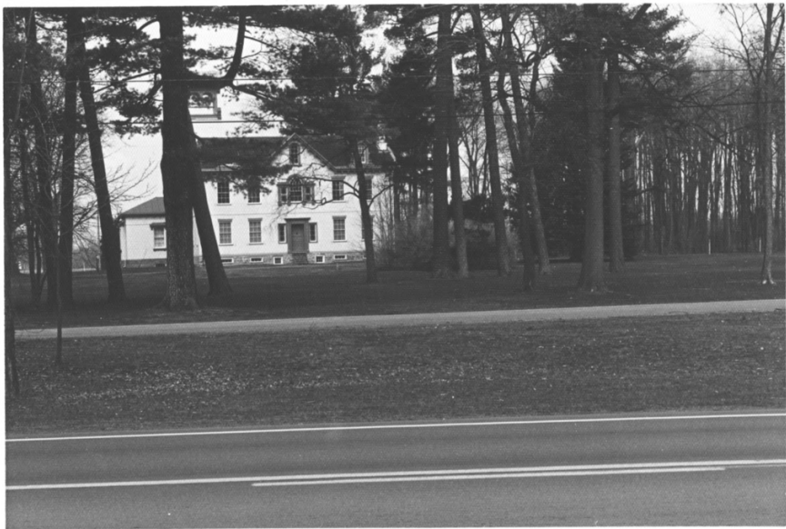
Lindenwald mansion with Route 9H in foreground and Old Post Road in center. Looking west.
