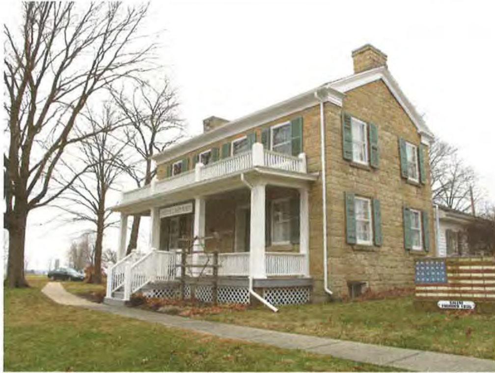
Figure 9. Henderson Lewelling House, 401 S. Main, Salem, Salem Township, circa 1842, coursed ashlar sandstone construction, listed on NRHP (McCarley, December 2014).
