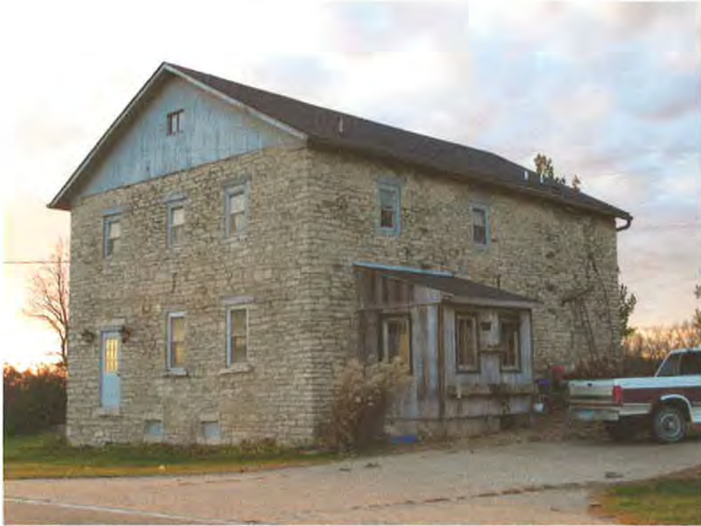
Figure 11. Dennis Melcher Pottery, Agency Road, on line of Section 36, Baltimore Township (Henry Co) and Des Moines County, circa 1851, coursed rubble limestone construction, listed on NRHP (McCarley, October 2014).
