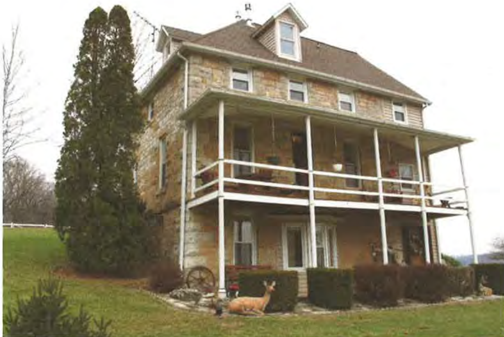
Figure 12. Leonard Farr House, on 286 th St off of Agency Road, Section 5, Salem Township, construction date unknown, coursed ashlar sandstone construction (McCarley, December 2014).
