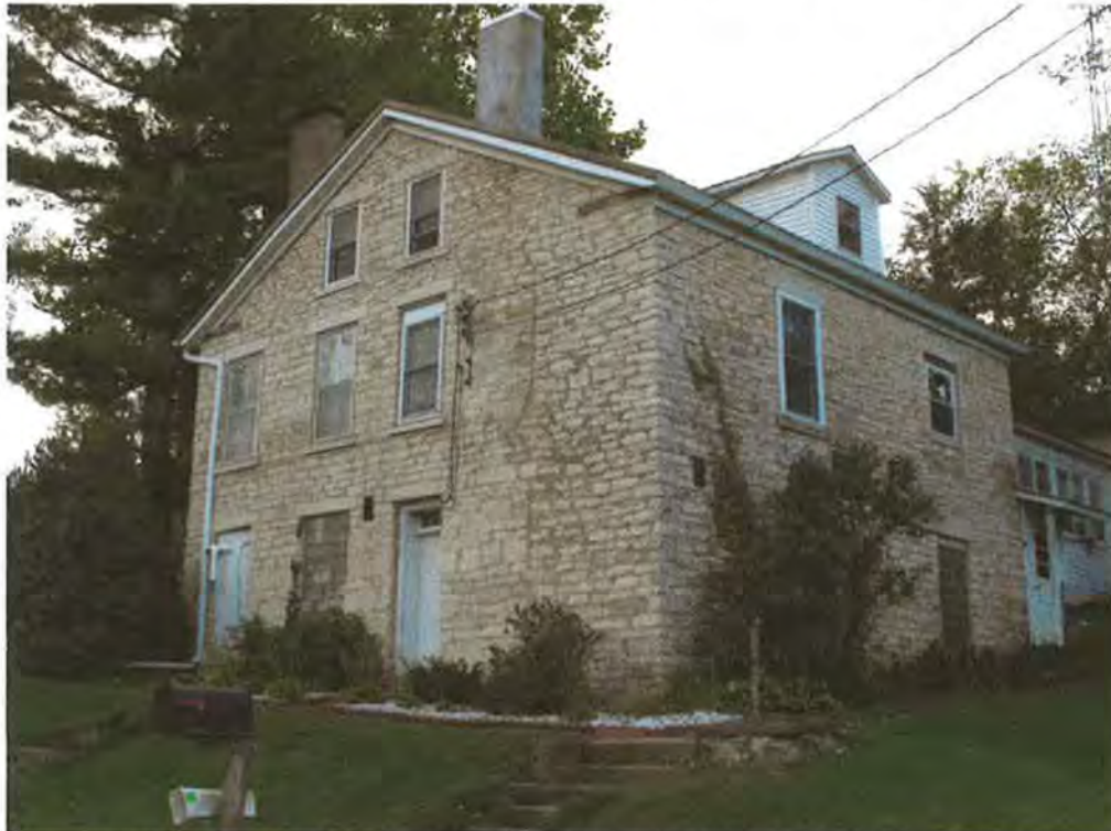
Figure 10. Hugh and Matilda Boyle House, Salem Road, Section 25, Jackson Township, circa 1850, coursed rubble limestone construction, currently nominated to NRHP (McCarley, December 2014).
