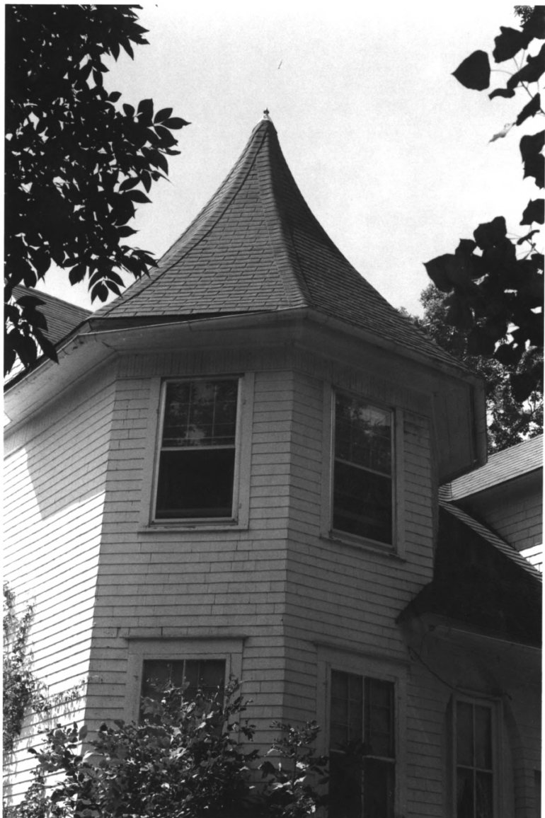
Amy A. Davis House, Codrington Co., S.A., No. 3
