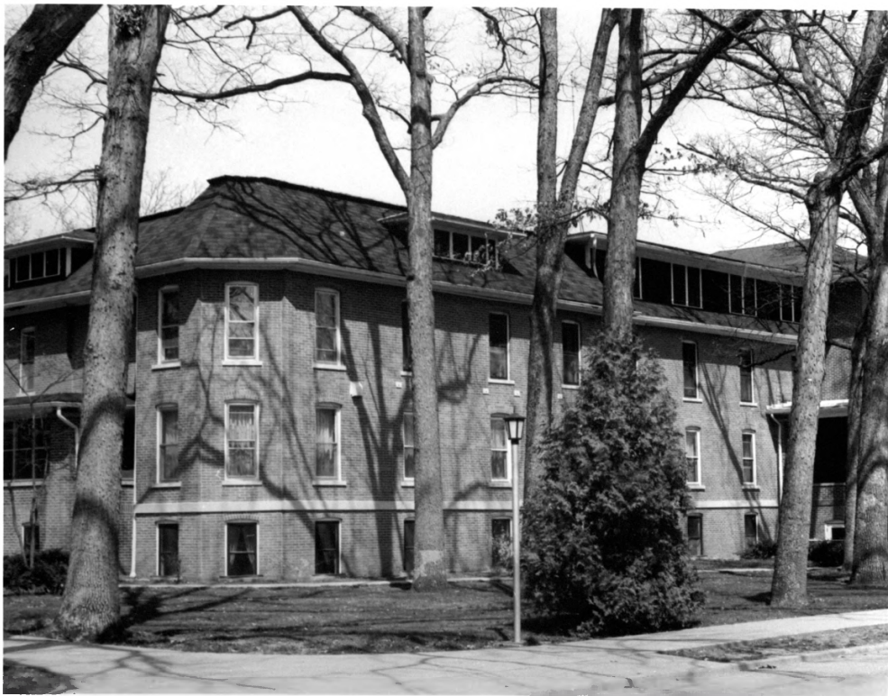
#10 Manchester College Historic District Wabash County Indiana
