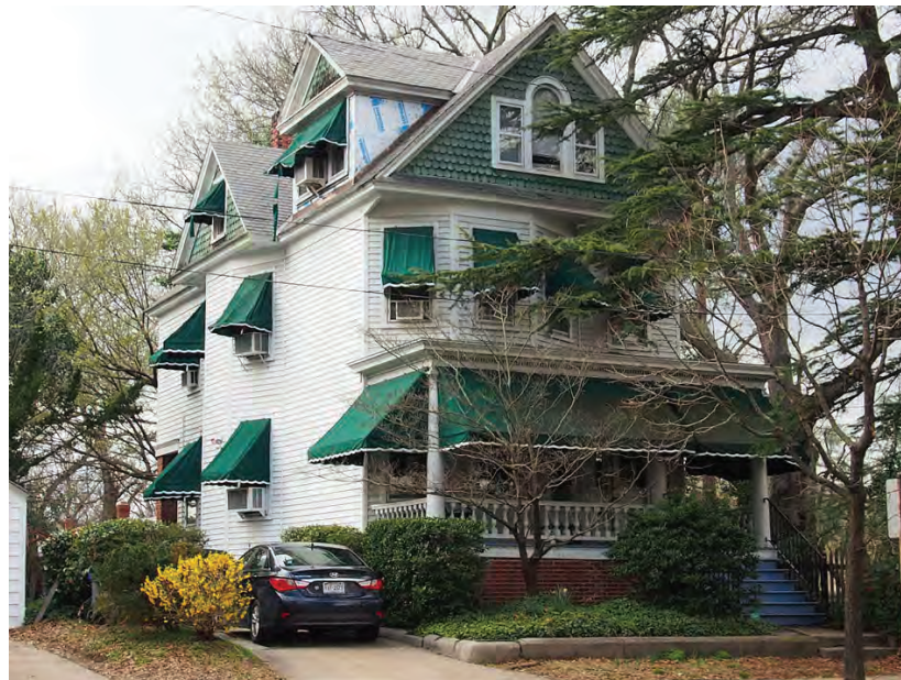
Figure 3. House at 3709 Llewellyn Avenue, Looking Northwest
