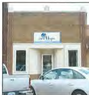
Prior to rehabilitation in 2013.
