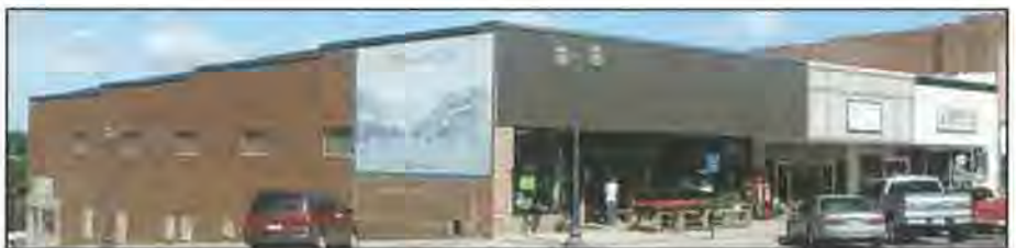
Prior to rehabilitation in 2013.
