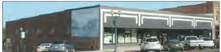
Following rehabilitation in 2014.
