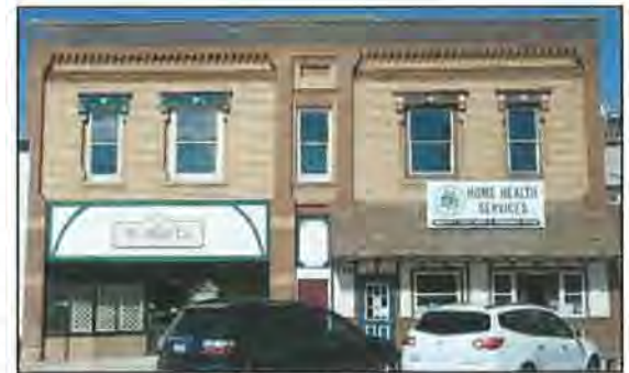
Prior to rehabilitation in 2013.
