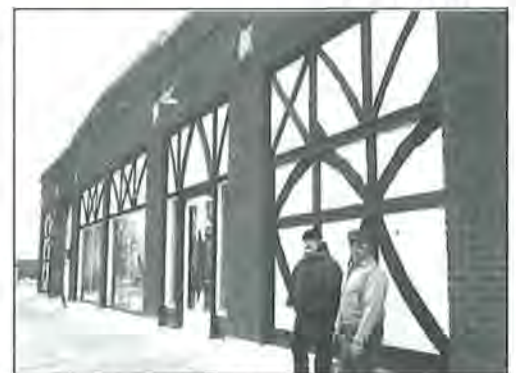
Façade of 303 Center Street late 1970s-1980s. Copy provided by Manning HPC, 2012.
