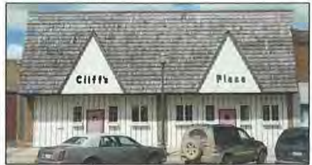
Prior to rehabilitation in 2013.
