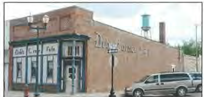
Prior to rehabilitation in 2013.
