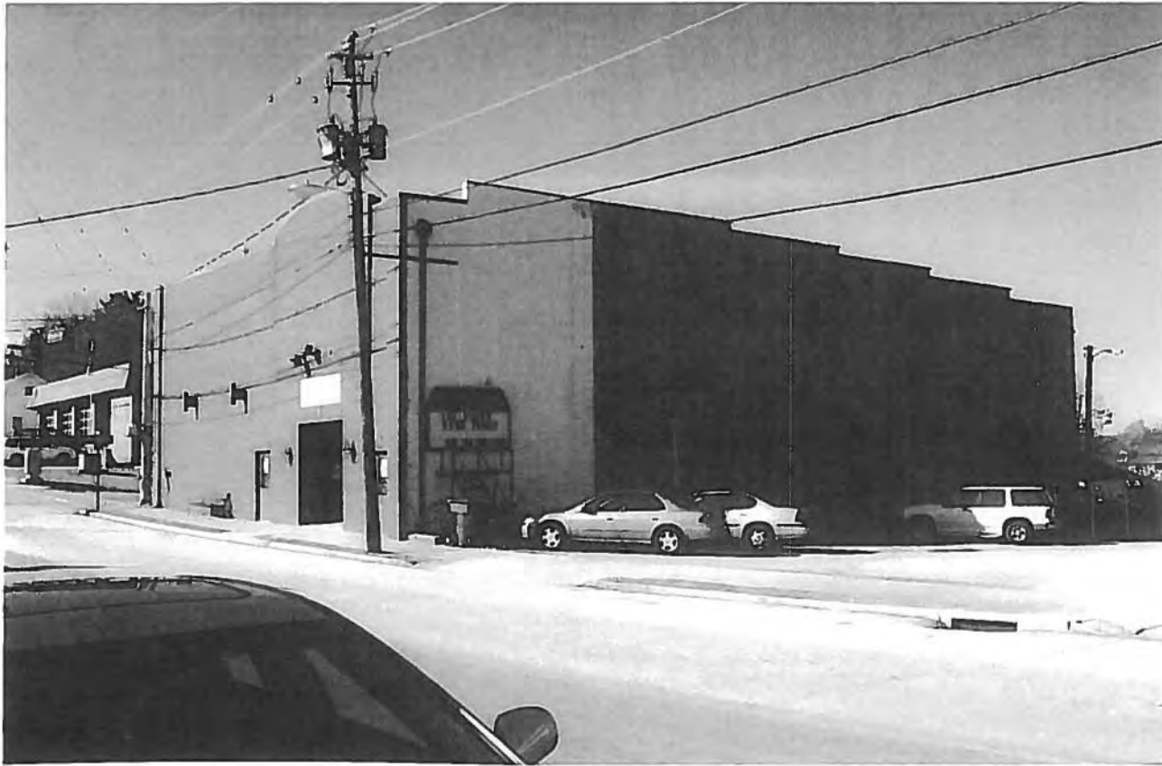
Ritz Theater 2012 Prior to removal of brick façade
