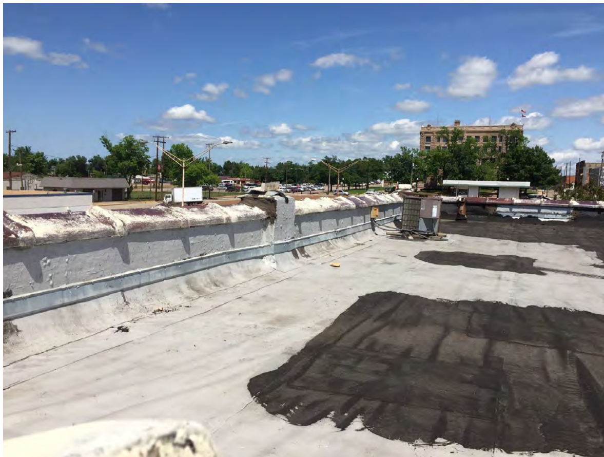
Photo 4 View of roof Camera facing East
