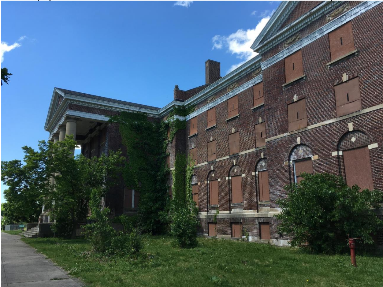
Main Administration Building, main (east) façade, 2017
