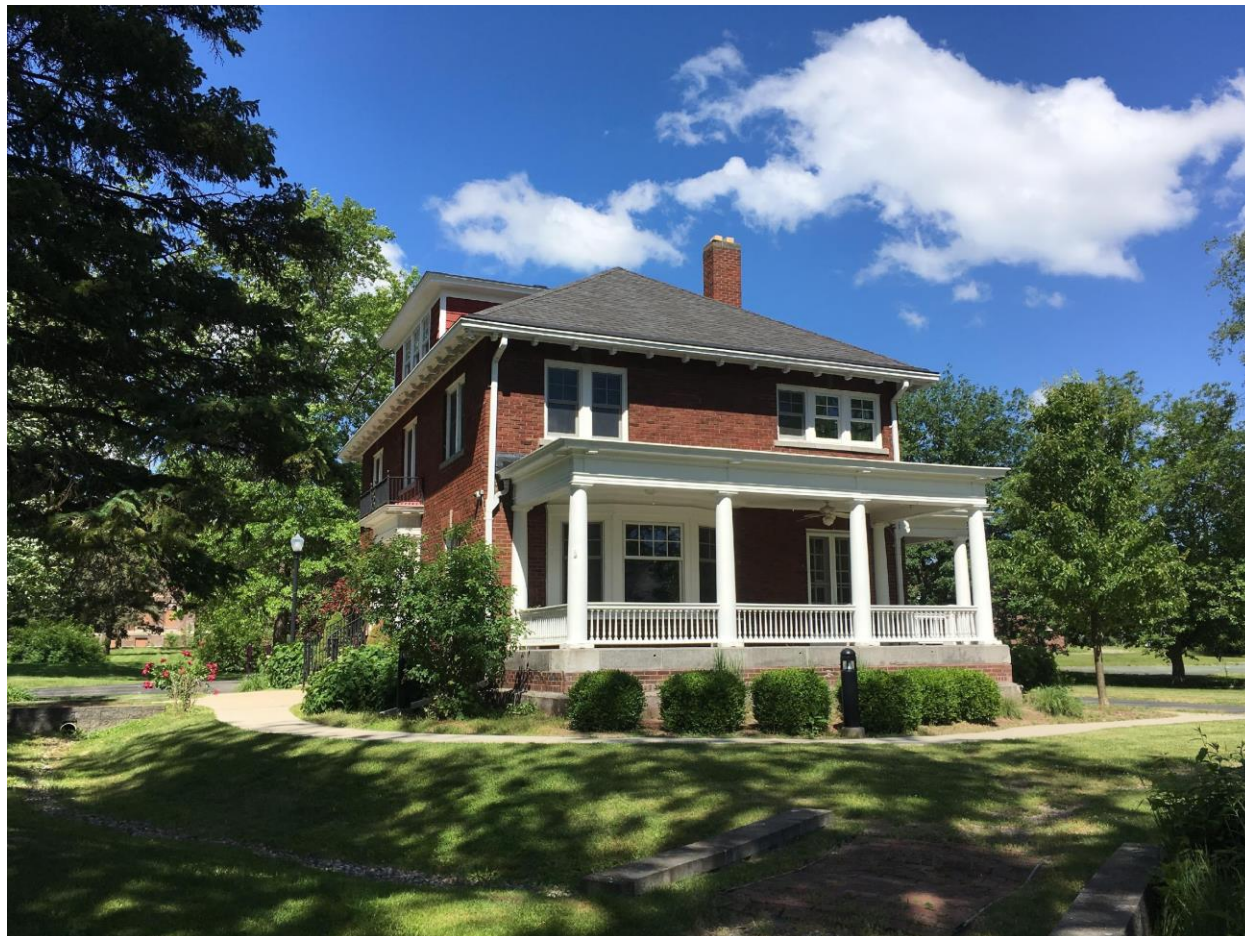
Superintendent's House, south and east facades, 2017
