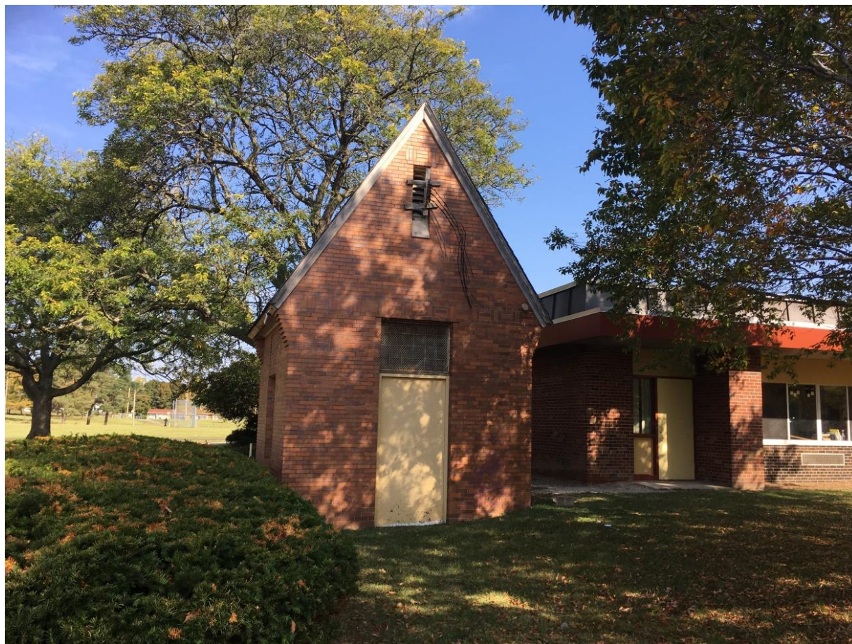
Pump House, located by the Elementary School, at the south side of the campus, 2017
