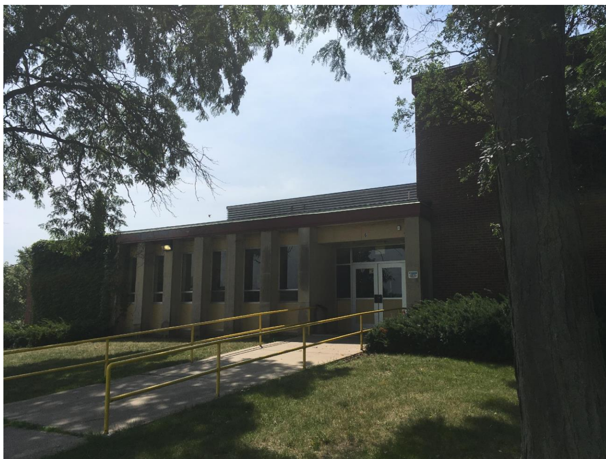
Gymnasium/Pool, entry at north façade, 2017
