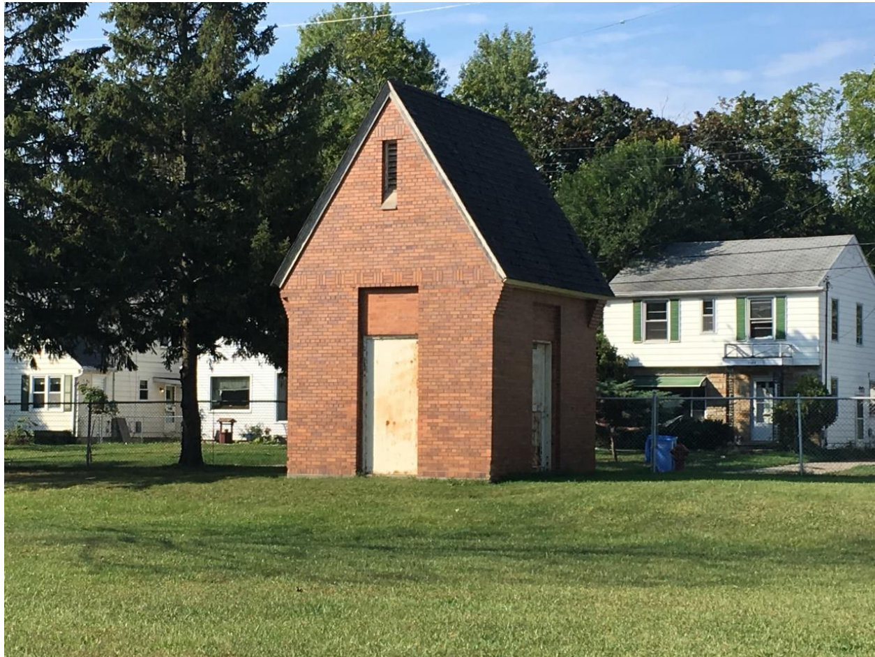
Pump House, located at the west end of the campus, 2017
