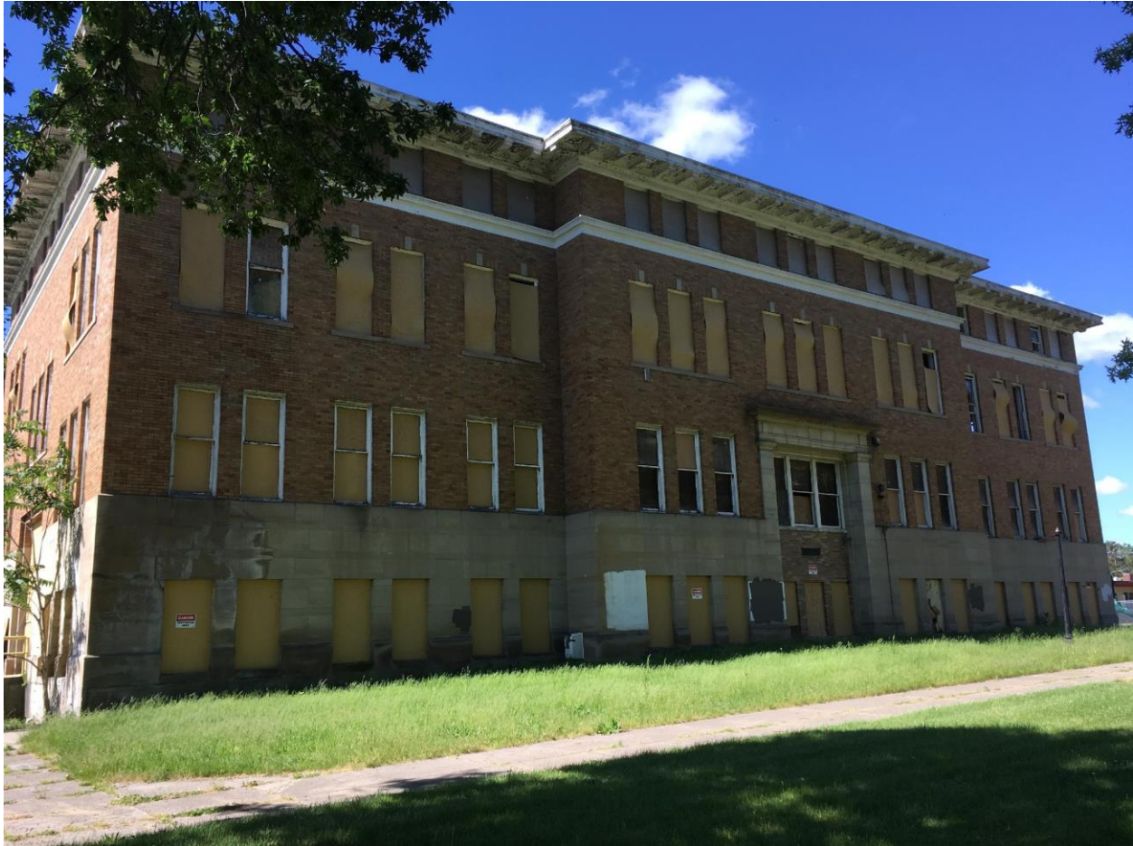
High School Building, main (north) façade, 2017
