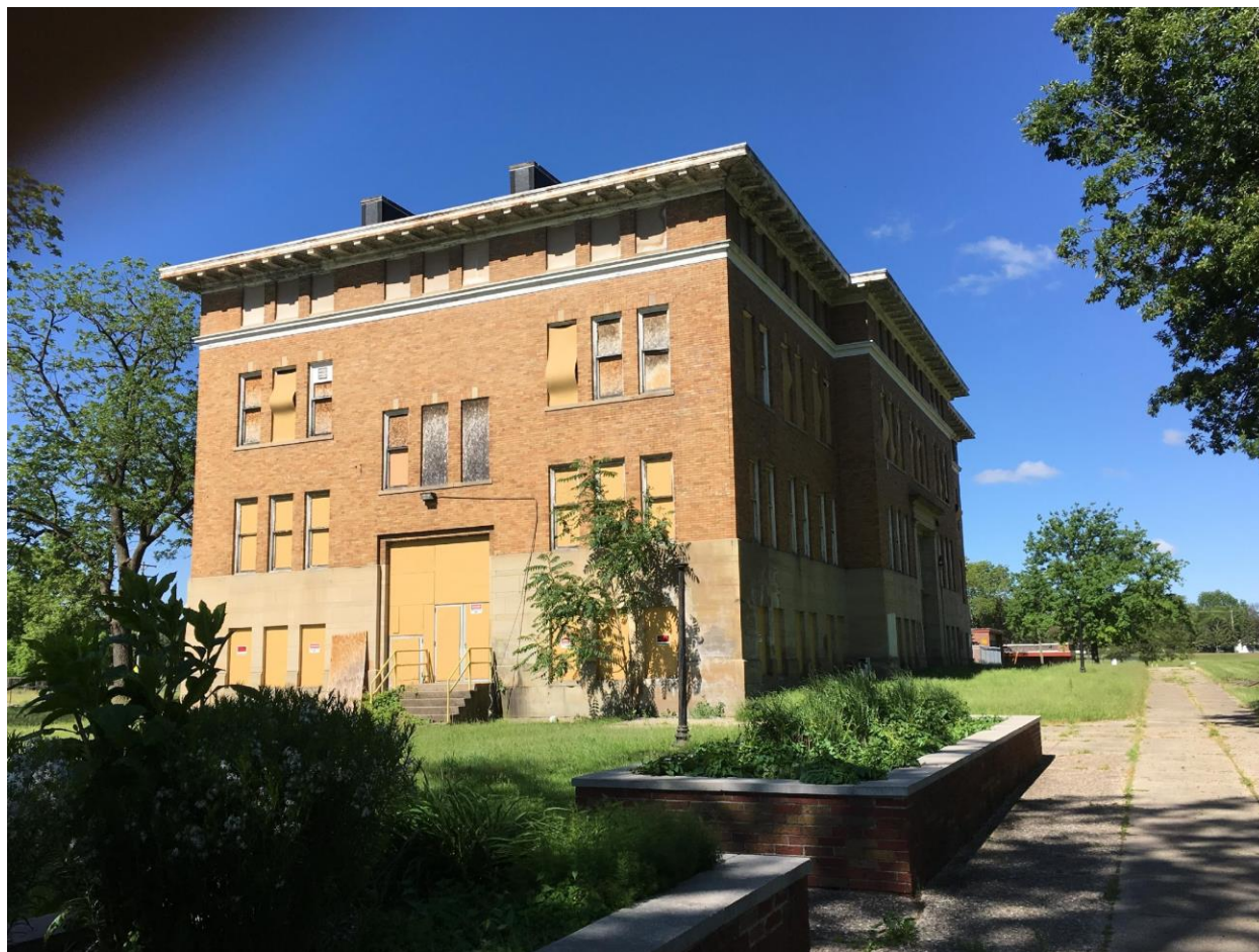
High School Building, east and north (front) facades, 2017
