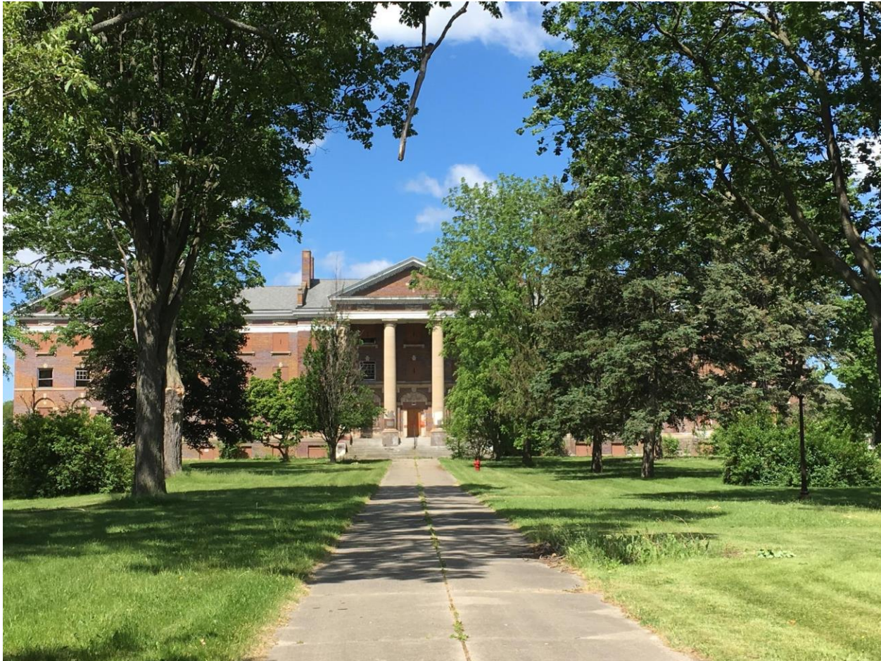
Main Administration Building, main (east) façade, 2017
