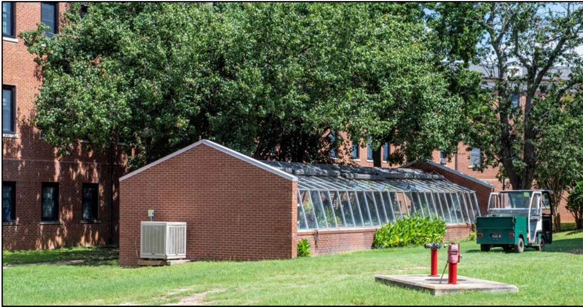
Figure 38. Perspective view of the greenhouse with Building No. 16 in the background, 2018 (VA).
