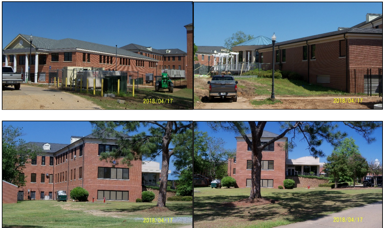
Figure 25. Views of Building No. 10 (top) and Building No. 12 (bottom) in 2018 (VA).
