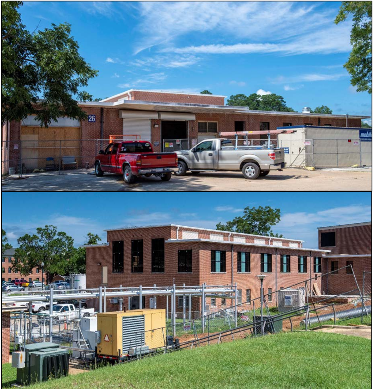
Figure 28. Views of the laundry (Building No. 26) in 2018 (VA).
