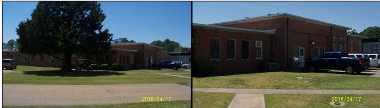
Figure 32. Contemporary views of Building No. 29 – (top, left) view looking north into the maintenance quadrangle with the L-shaped building on the right of the photograph; (top, right) view looking southeast to Building No. 29 with Building No. 81 in the background; (middle, left) view looking northwest into the maintenance quadrangle, note the latticed parking area in the center and Building No. 66 in the background; (middle, right) oblique view looking west with building No. 66 in the background; (bottom, left) perspective view looking southwest at the north elevation, note the annex in the background; (bottom, right) closer view (VA).
