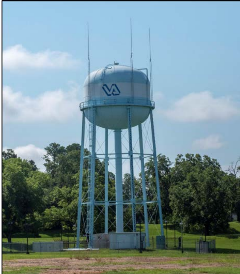
Figure 12. General view looking to the water tower.
