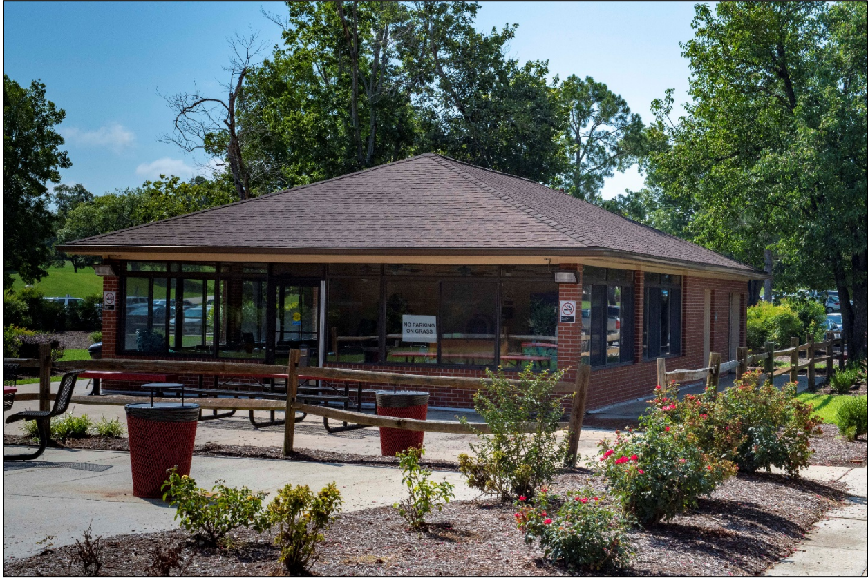
Figure 37. General view of Building No. 63 in 2018 (VA).
