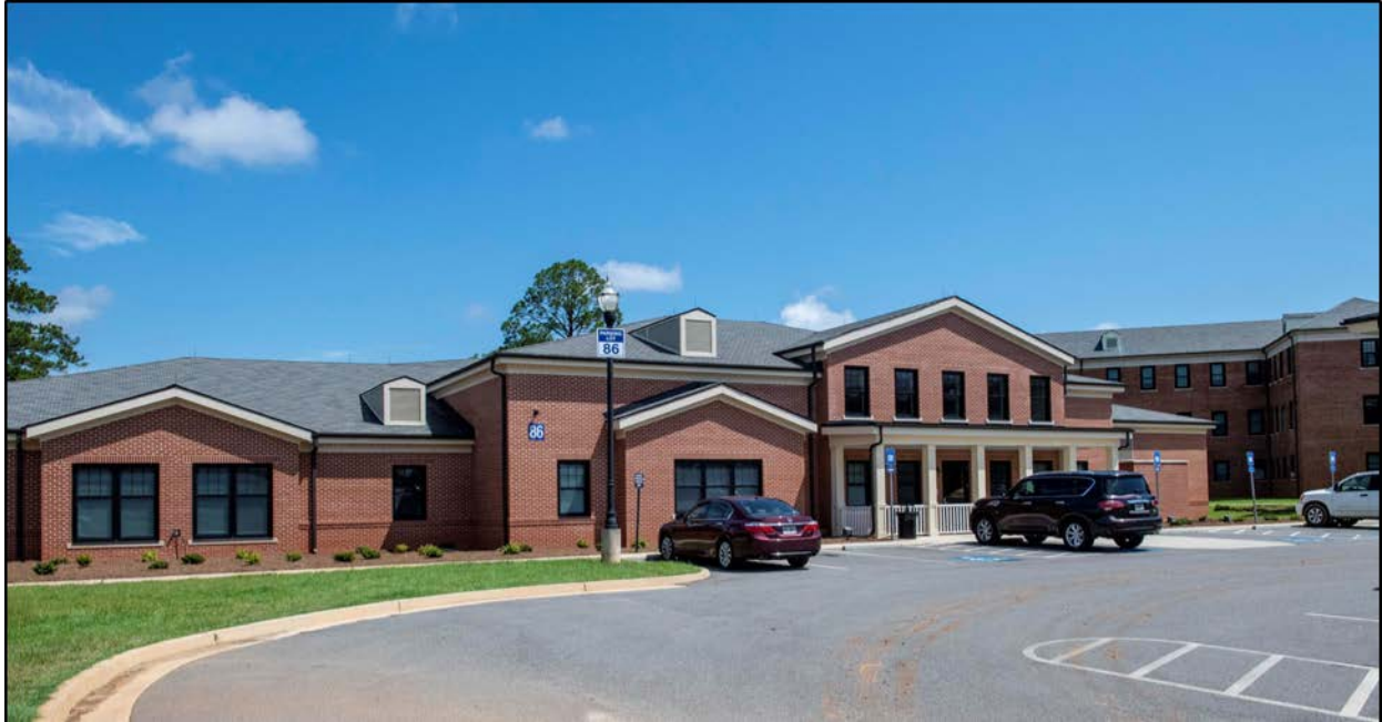
Figure 40. Views of Building No. 86 in 2018 (VA).
