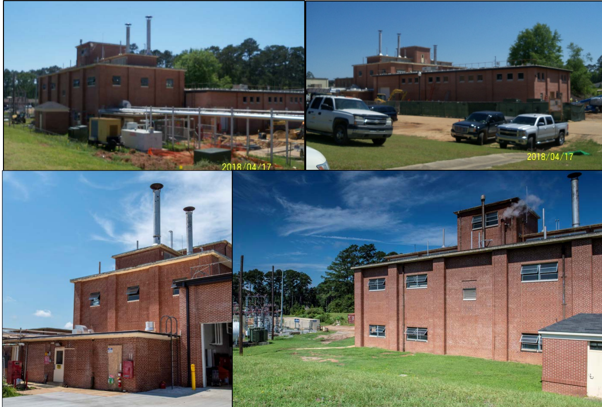
Figure 30. Views of the boiler plant that include Building No. 72 in front and the chiller plant to the rear, 2018 (VA).
