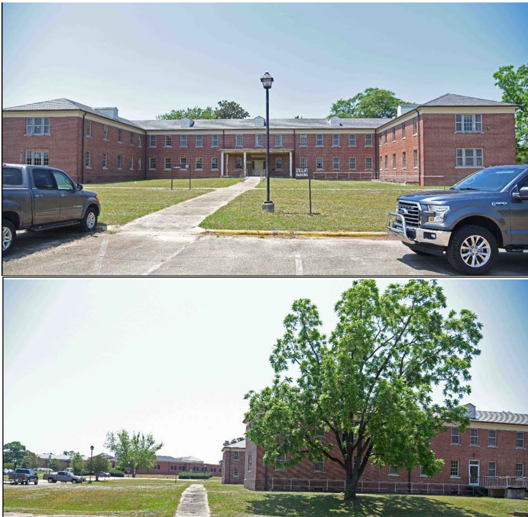
Figure 34. Front and side elevations of Building No. 34 in 2018 (VA).
