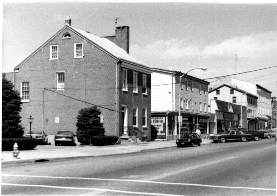
#10: 400 block of High Street, west side, looking northwest
