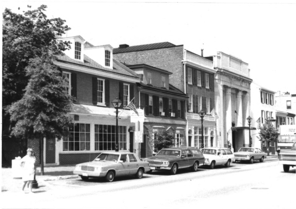
#6: 300 block of High Street, west side, looking northwest
