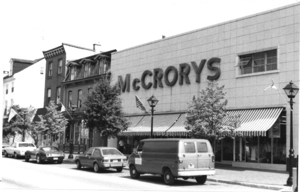
#7: 300 block of High Street, east side, looking north.
