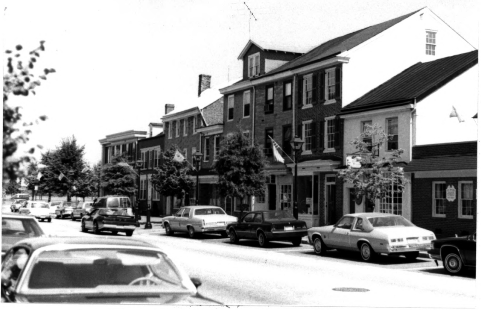
#1: 200 block of High Street, east side, looking north.
