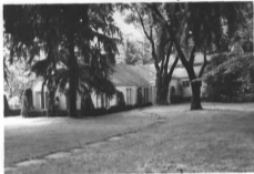
View looking SE showing early 20th c. rear wing of the Carlock House. neg. file # 19848-23
