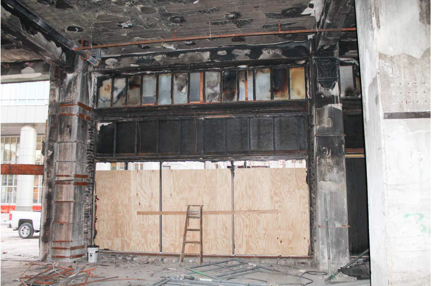
Photo 6 of 11: INTERIOR: First floor – South elevation storefront, looking south
