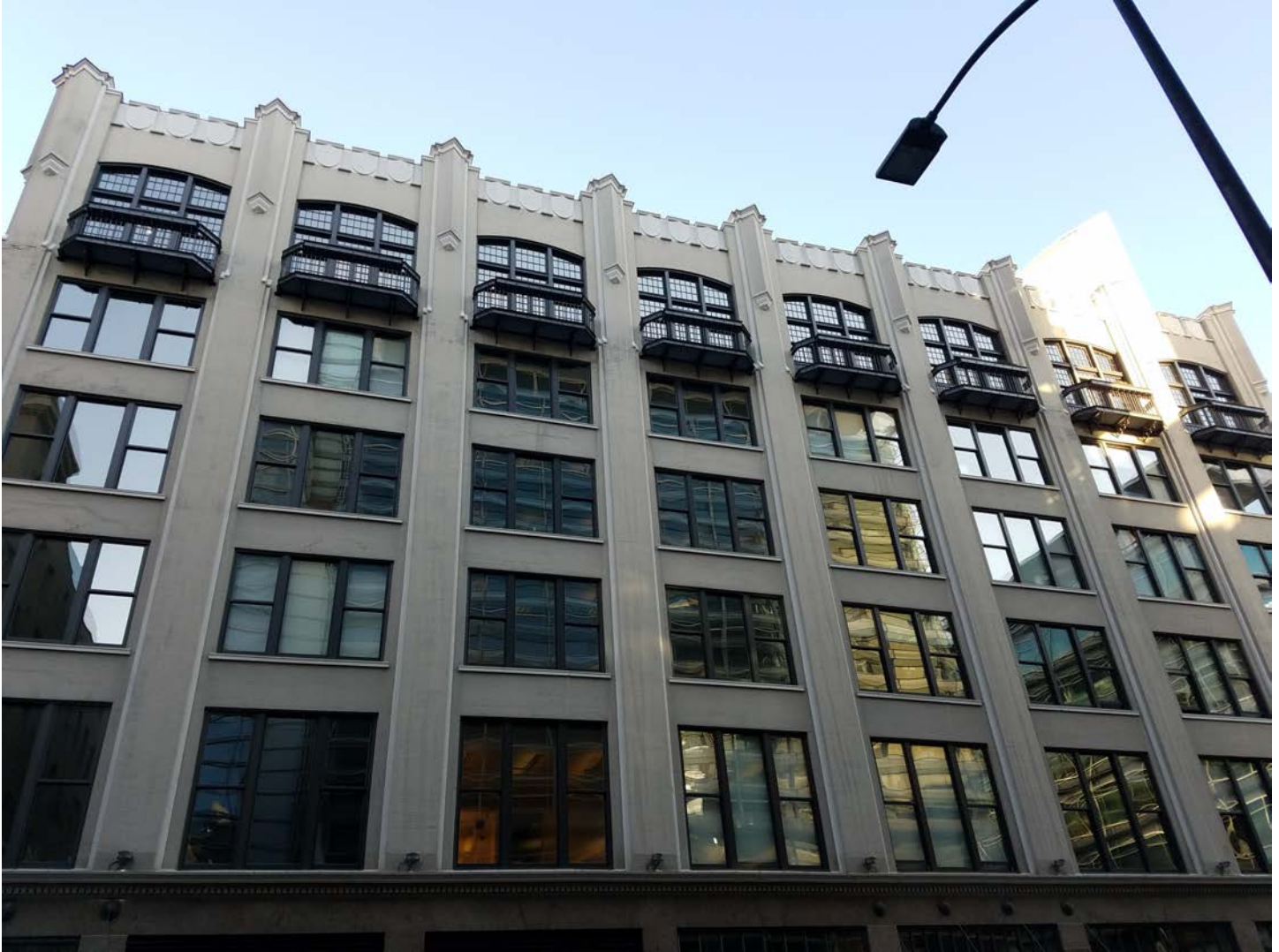
Photo 2 of _18_: EXTERIOR: South elevation - fenestration
