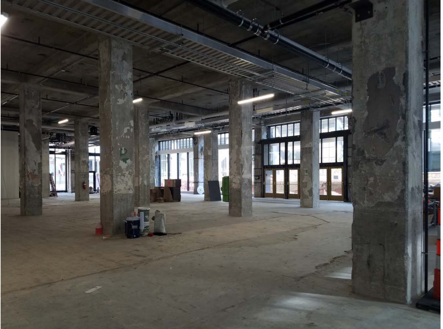
Photo 7 of _18_: INTERIOR: View of the first floor, looking SE
