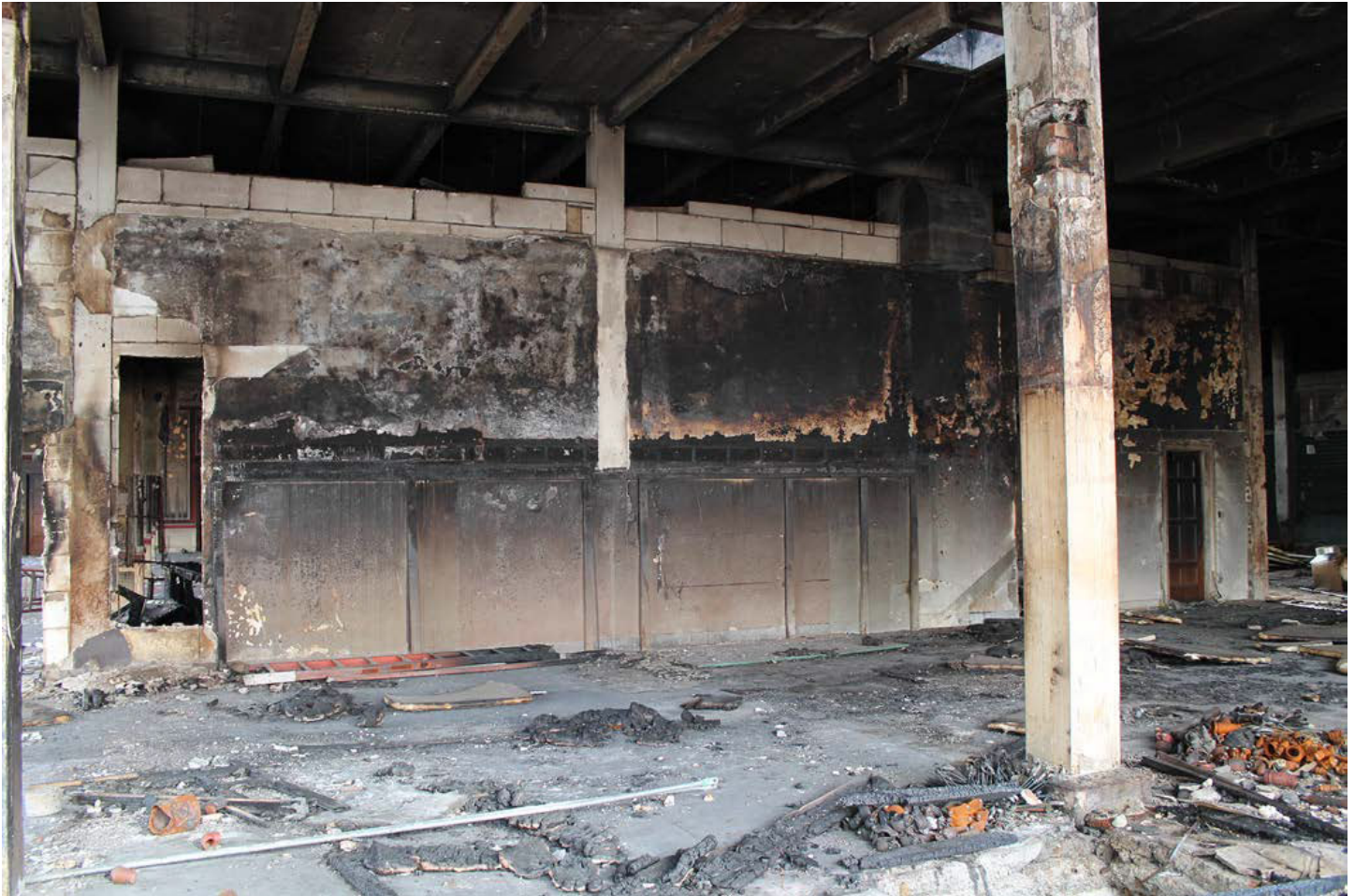
Photo 11 of 11: INTERIOR: Sixth floor, looking west
