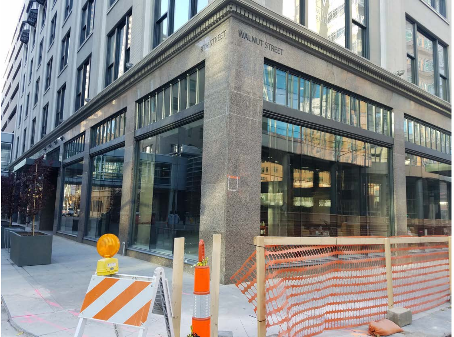
Photo 5 of _18_: EXTERIOR: Detail of storefronts – SW corner of the building
