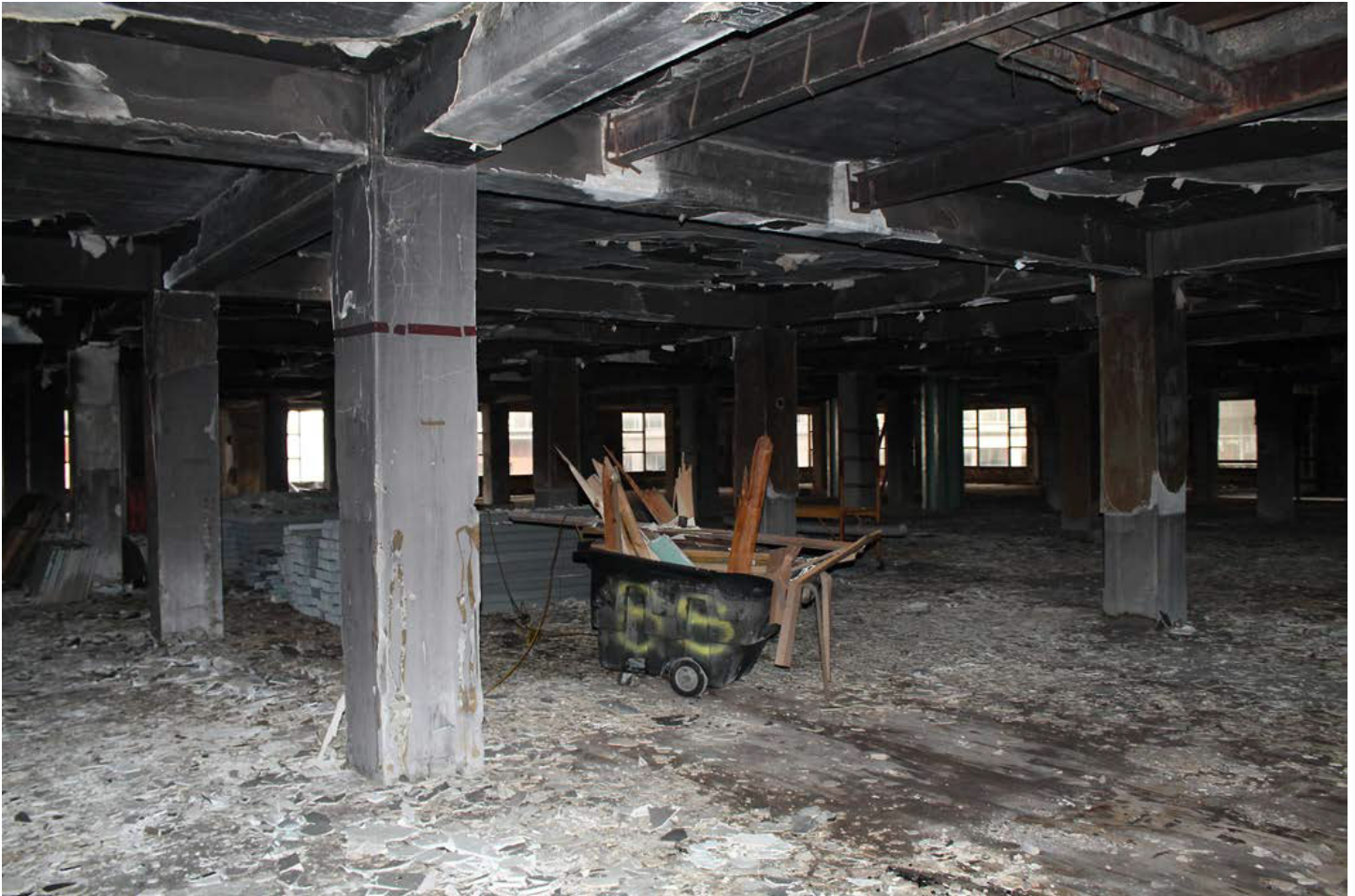
Photo 8 of 11: INTERIOR: Third floor, looking SW
