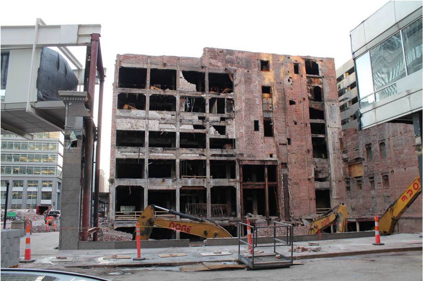
Photo 3 of 11: EXTERIOR: East elevation, looking west
