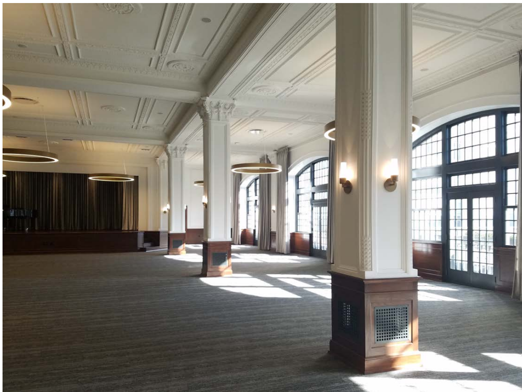
(Image courtesy of Neumann Monson, Architects – November 2017)
