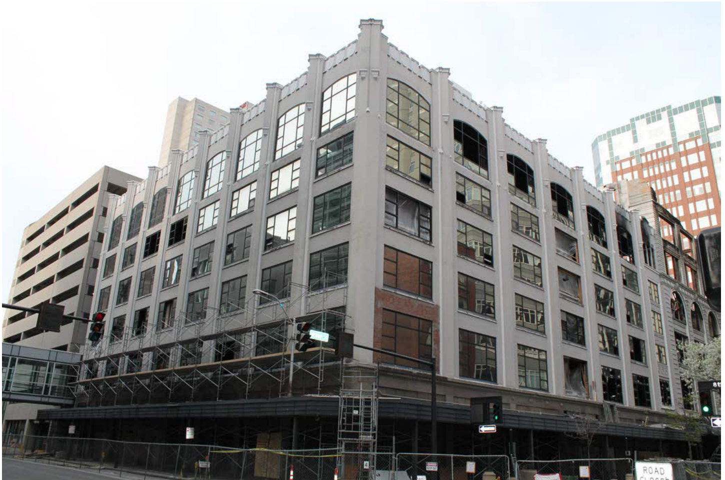
Photo 1 of 11: EXTERIOR: West and south elevations, looking NE
