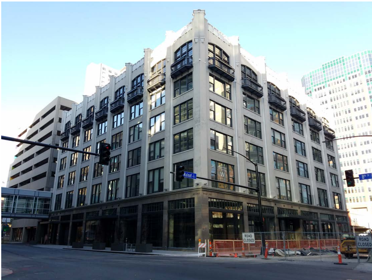
(Image courtesy of Neumann Monson, Architects – November 2017)
