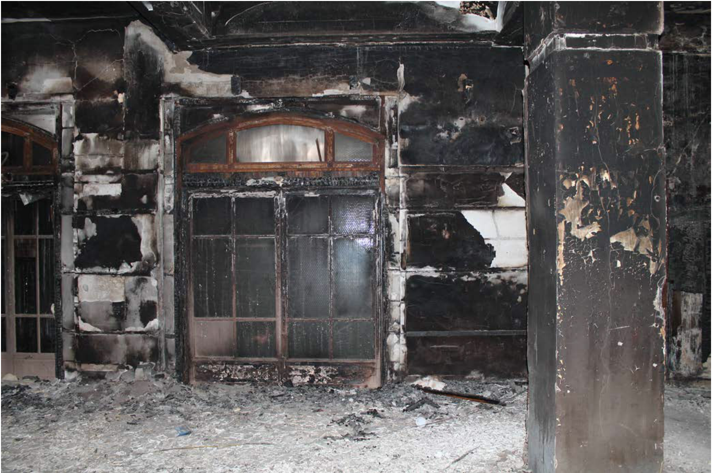
Photo 7 of 11: INTERIOR: Second floor elevators looking north
