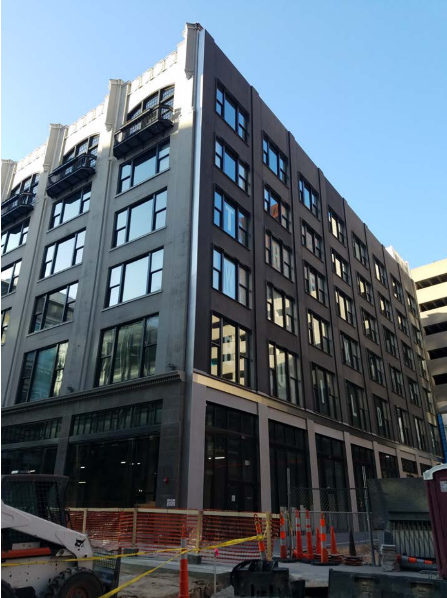
Photo 3 of _18_: EXTERIOR: South and east elevations, looking NW across Walnut Street
