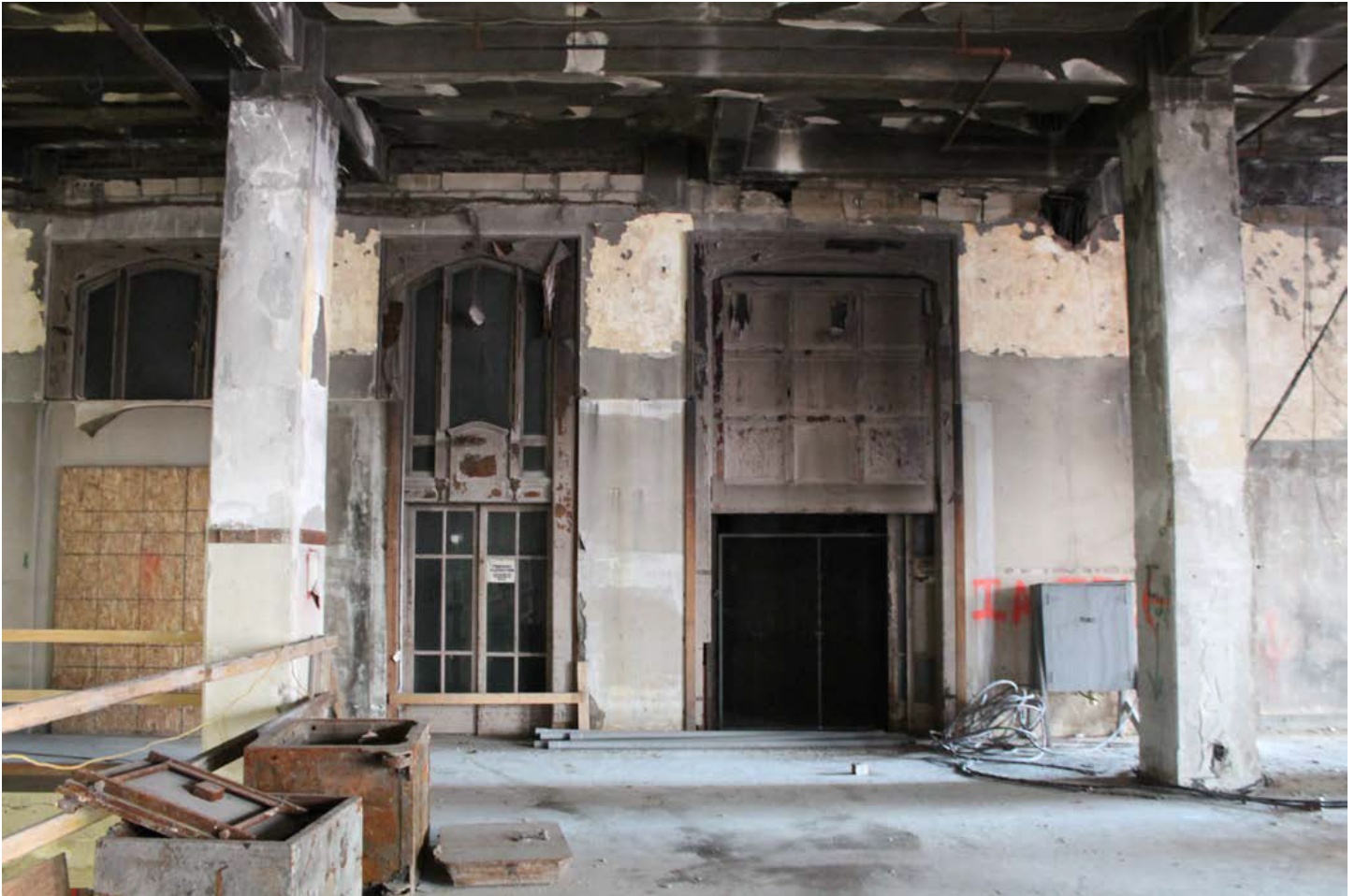
Photo 5 of 11: INTERIOR: First floor elevator doors, looking north
