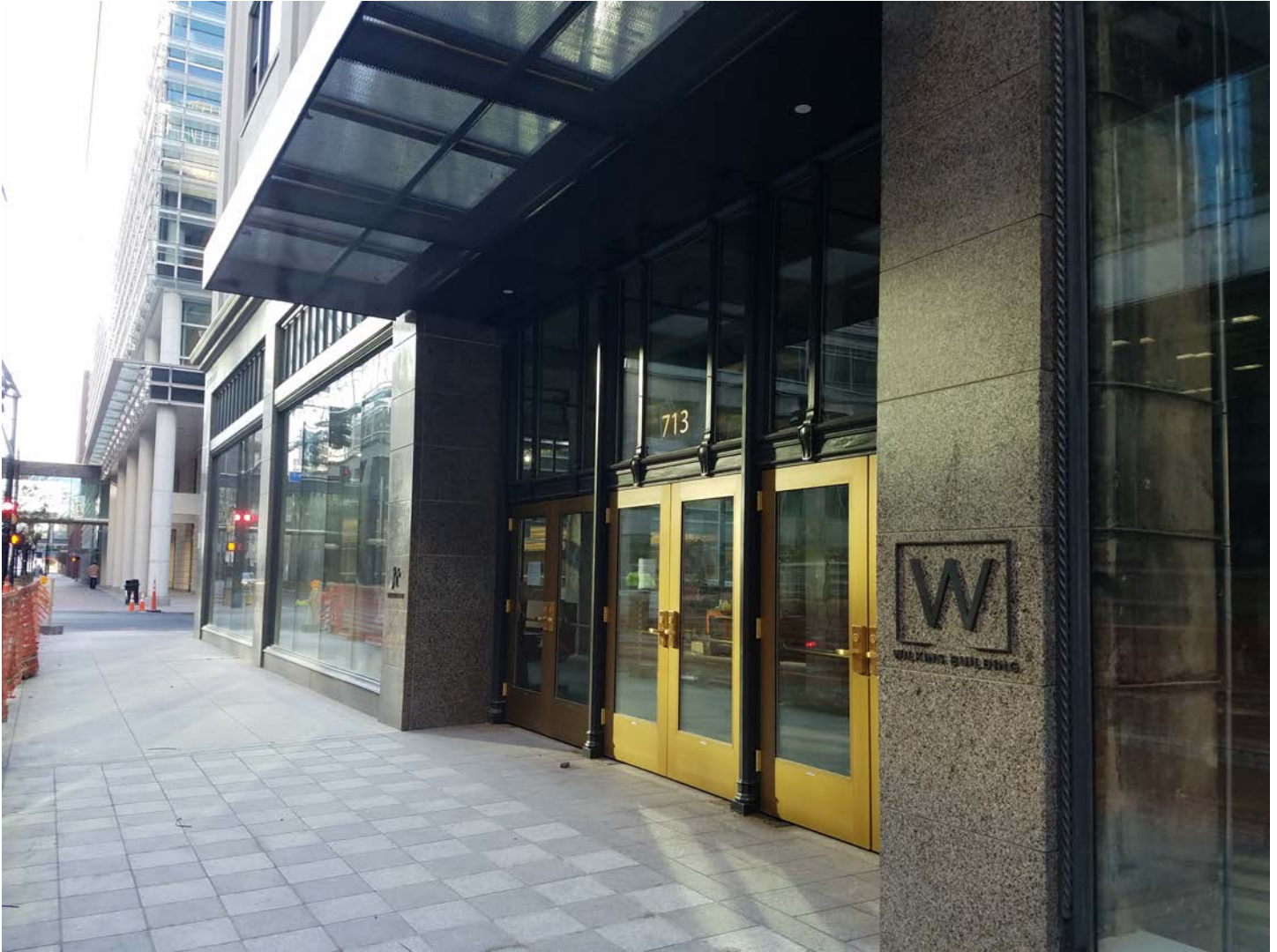
Photo 6 of _18_: EXTERIOR: Detail of storefronts and primary Walnut Street entrance
