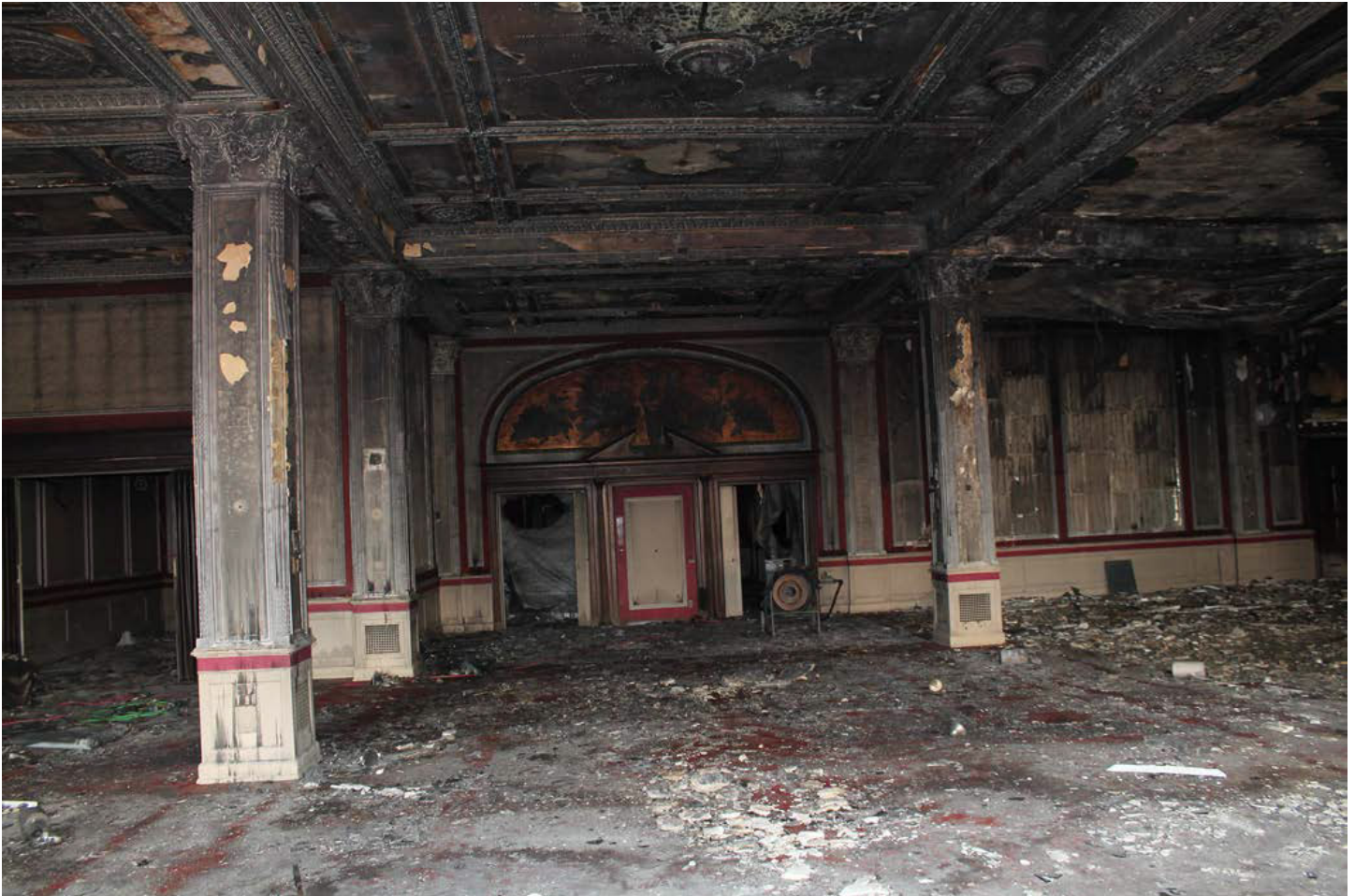
Photo 9 of 11: INTERIOR: Sixth floor – Yunkers Tea Room, looking north
