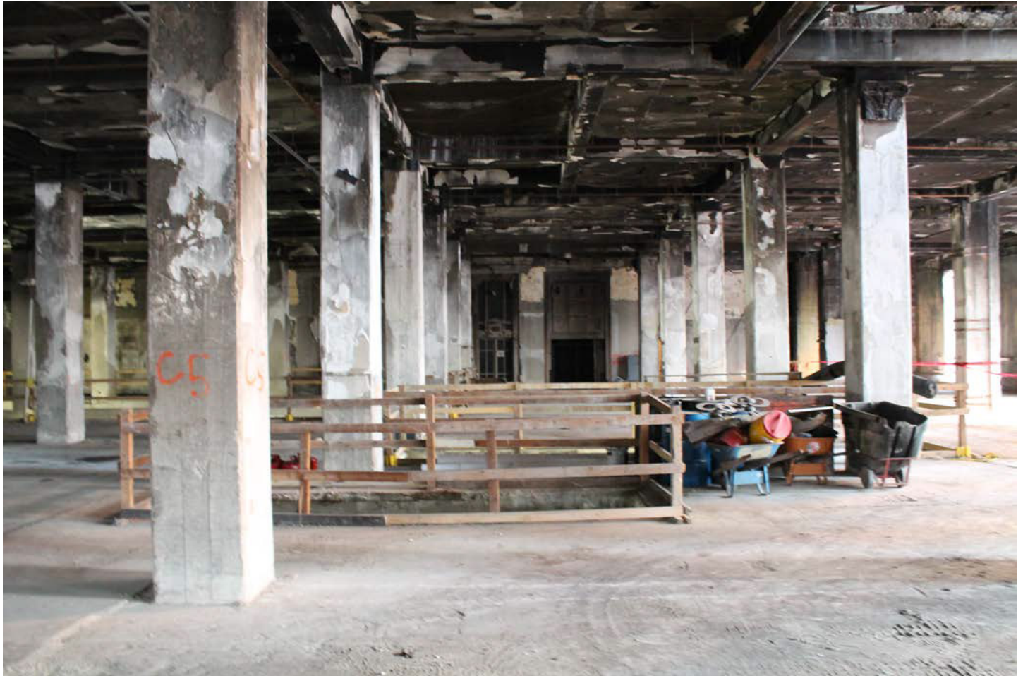
Photo 4 of 11: INTERIOR: First floor, looking north
