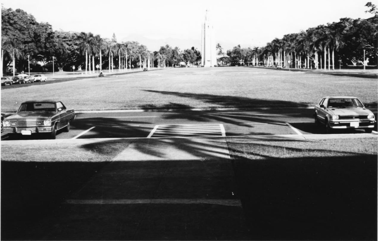
9. Hickam Field's water tower, a local landmark. Following the Japanese attack, the tower was covered with camouflage paint.
