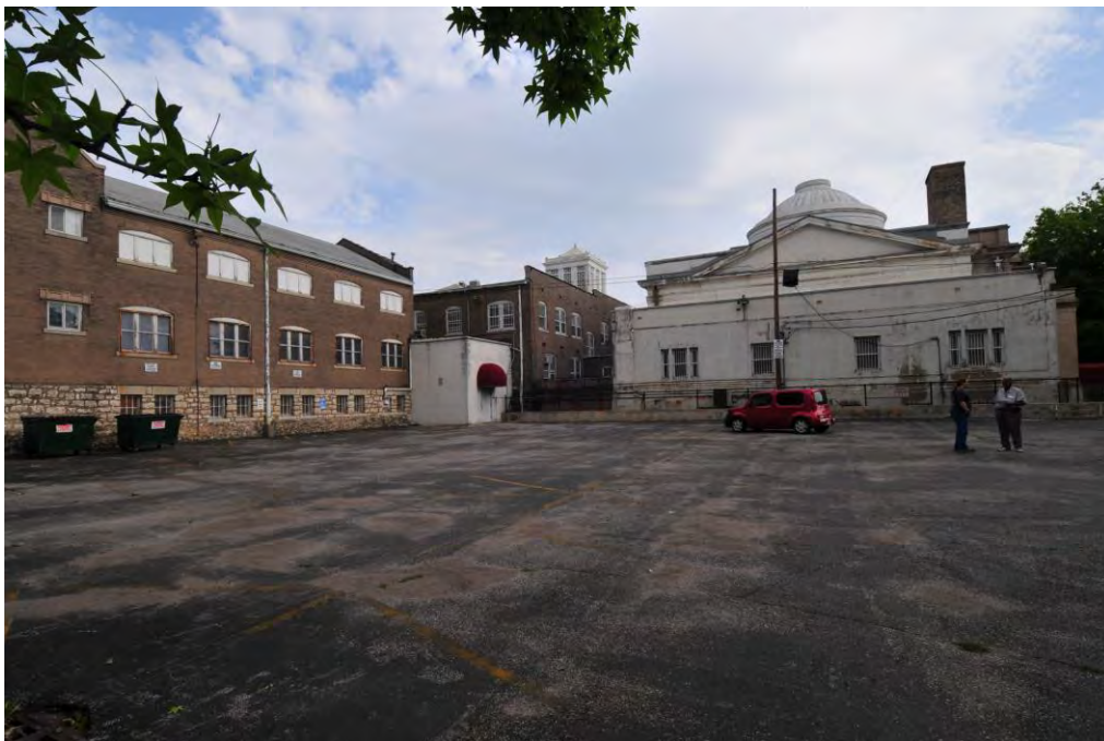
Photograph 4. South church elevation, east gymnasium elevation
