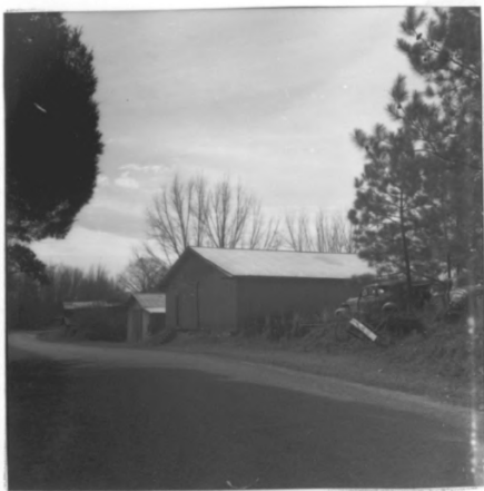
Shed (#21); Storage Building (#20)
