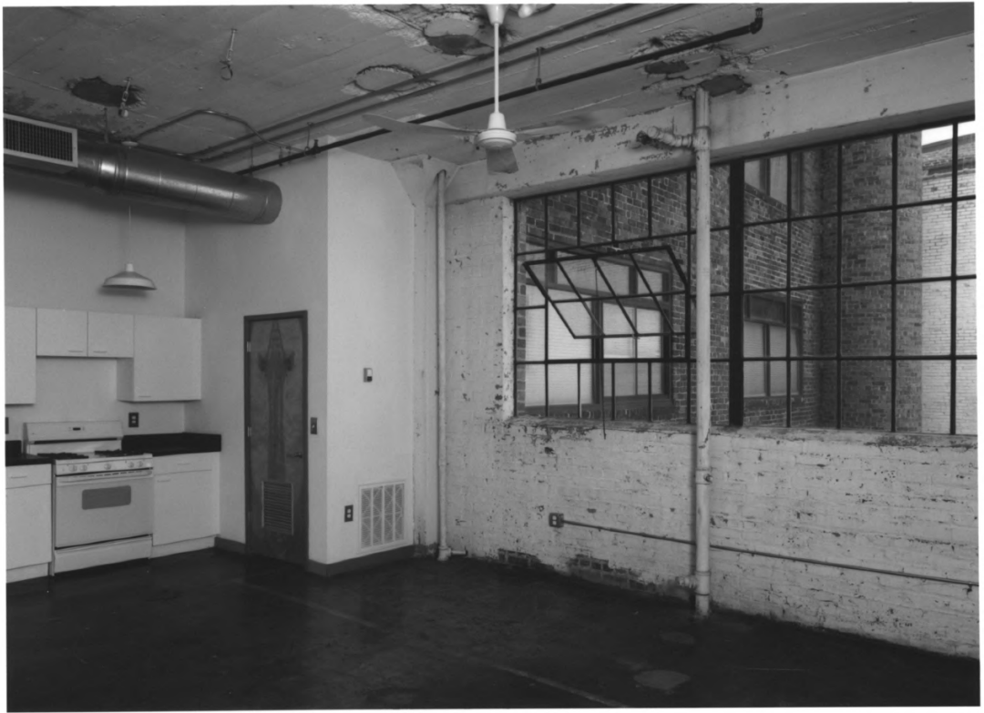
WESTINGHOUSE ELECTRIC COMPANY BUILDING ATLANTA, FULTON COUNTY, GEORGIA PHOTOGRAPHY 13 OF 15
