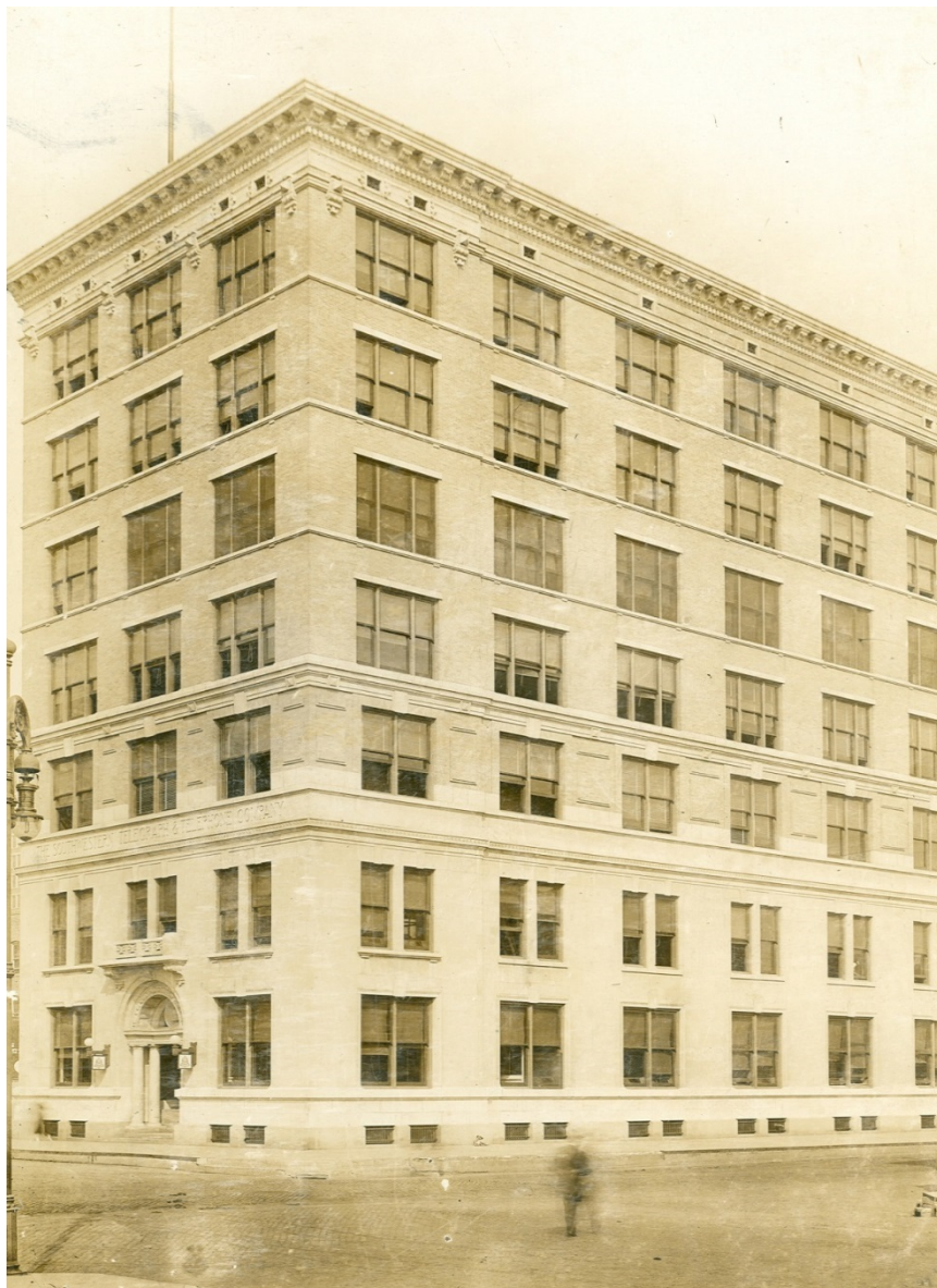
The Preston (now Capitol) Main Office and Exchange Building, circa 1912. View from southeast.
