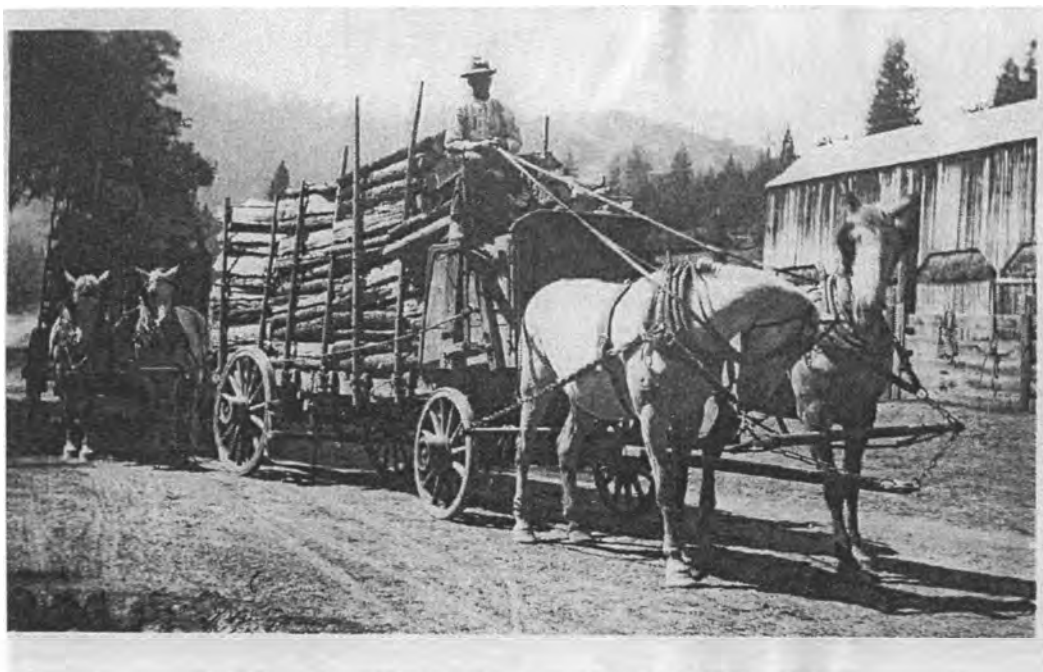
Figure 8. "Hauling Cordwood," 1918 (Note Barn) Burton Collection
