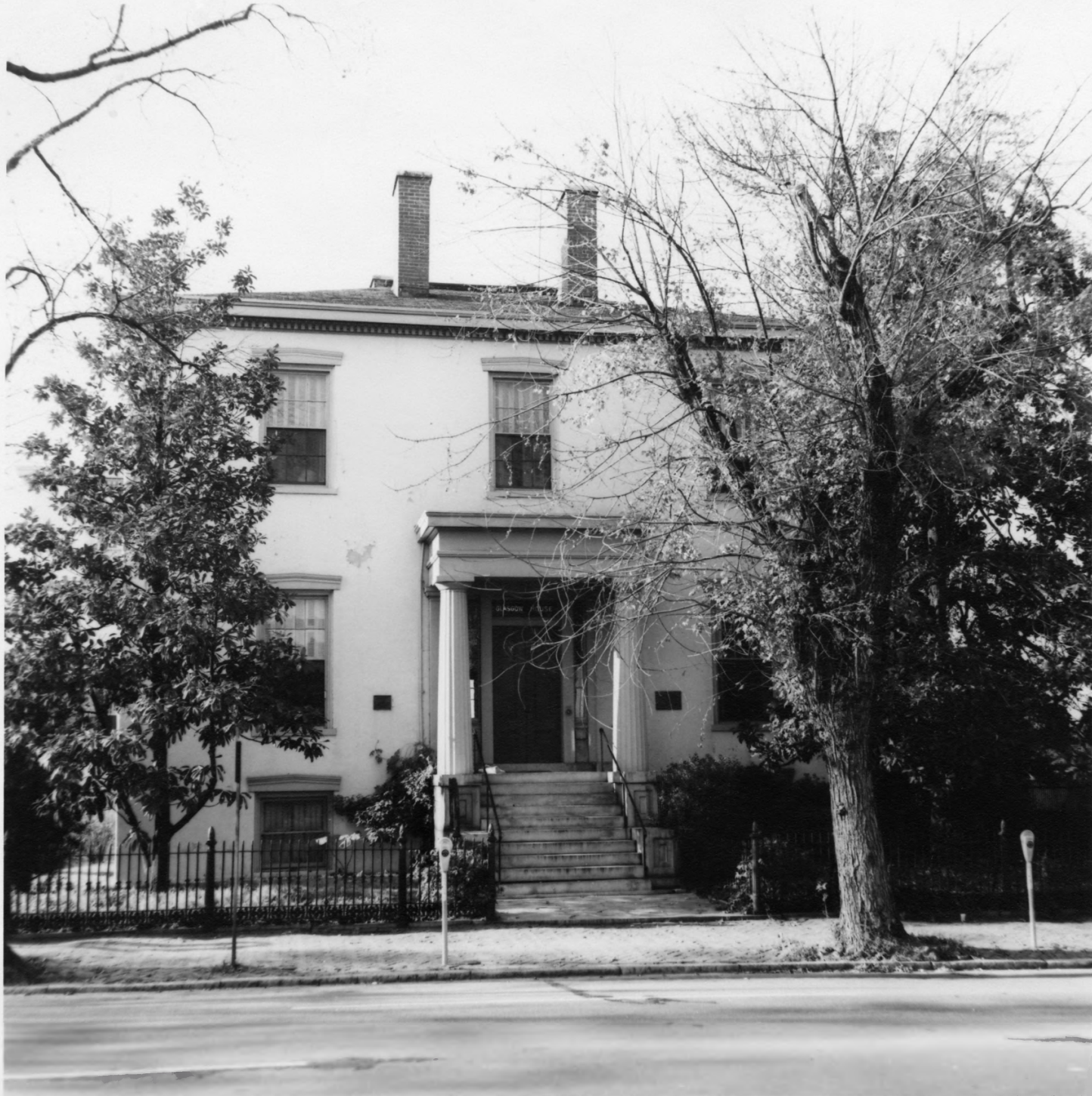
Ellen Glasgow House, Richmond, Virginia, North Elevation
