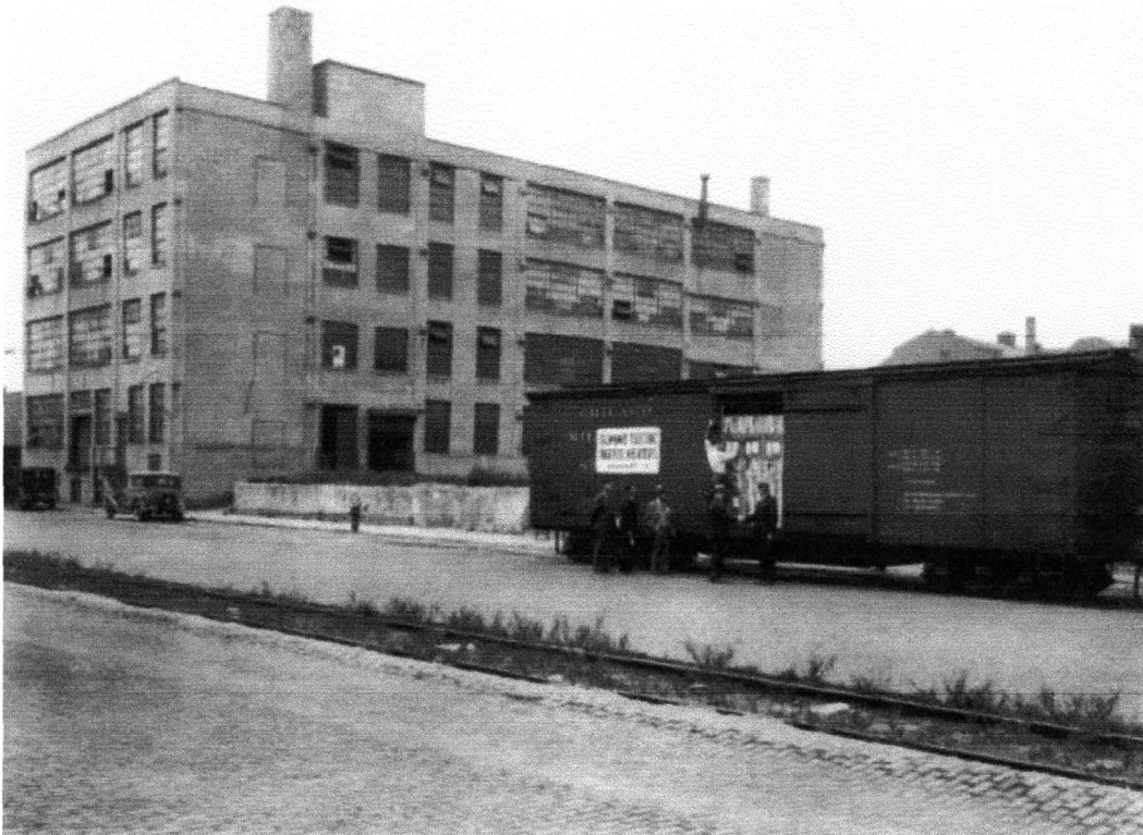
Judging from the cars in front of the building, this image of The Linograph Company Building dates to ca. 1933, which is several years prior to the 1949 construction of the addition. From this perspective, the large overhead door that provided access to the freight elevator is apparent. The image also documents the railroad line that ran along West River Drive (historically known as Front Street.)
