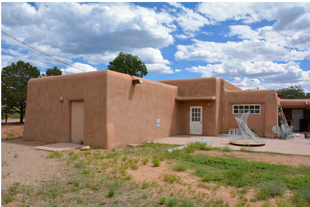
10. North elevation, east end, Darkroom in foreground, photographer facing southeast.
