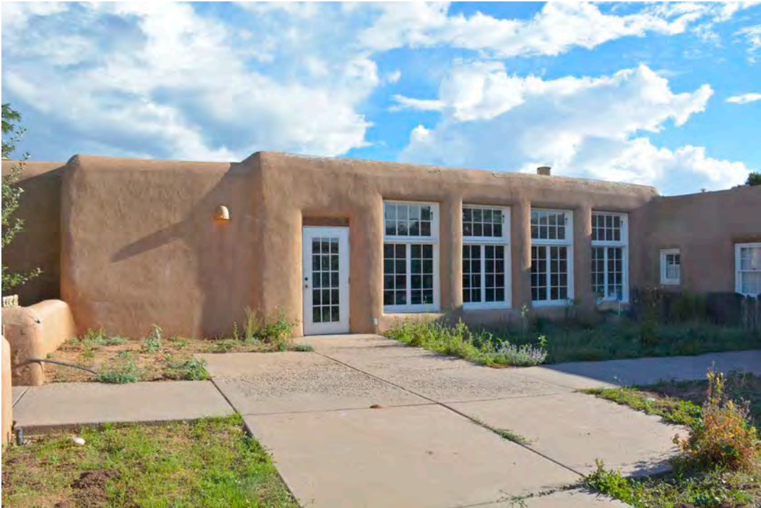
13. Courtyard, north elevation, Drafting Room, photographer facing southwest.
