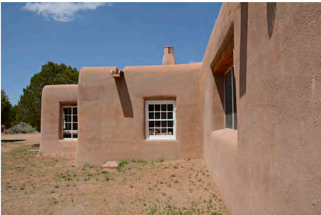
6. South elevation, west end, photographer facing north.
