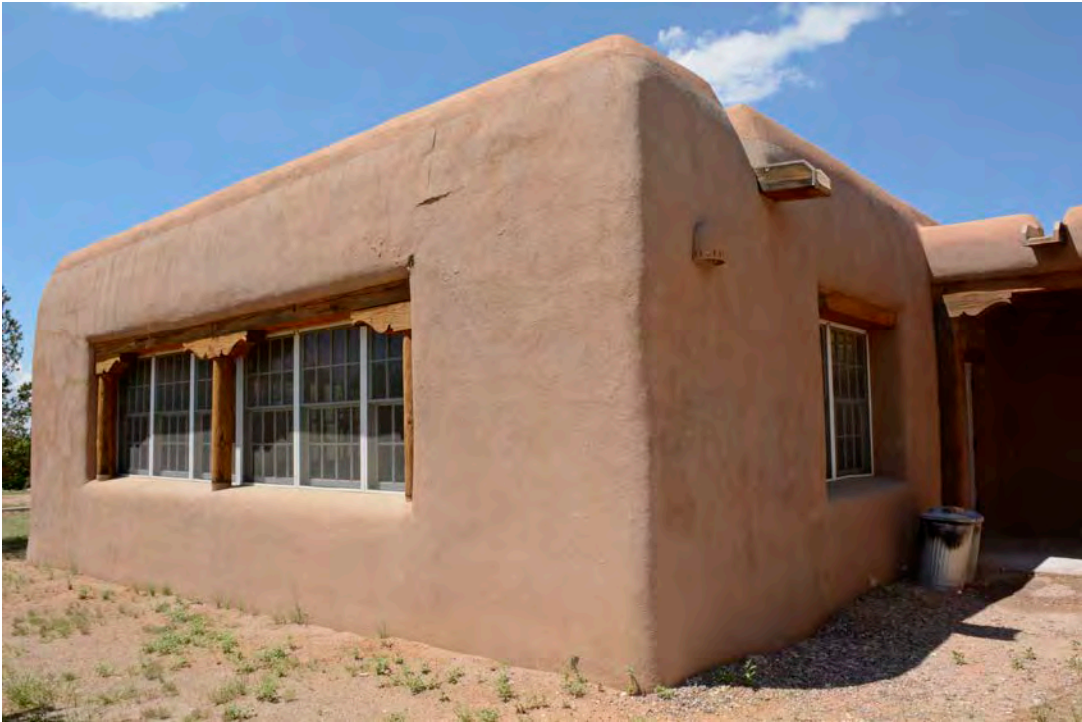
7. South elevation, 1996 Ceramics Studio addition, photographer facing northwest.
