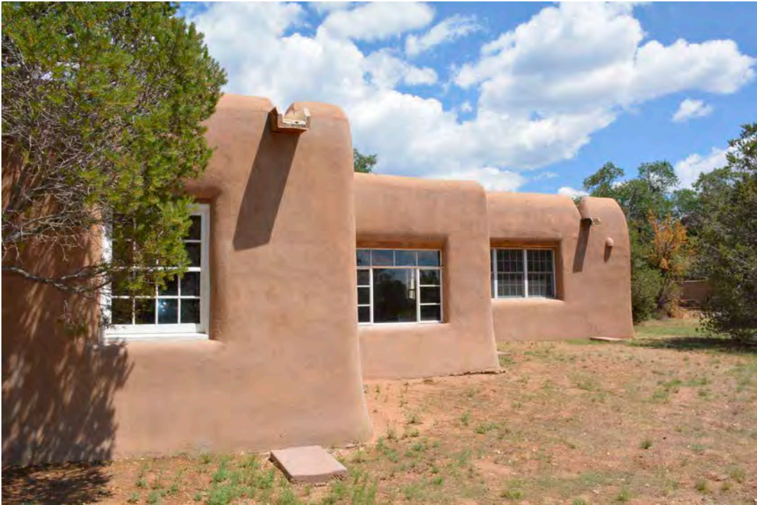
5. West façade, south end, photographer facing southeast.
