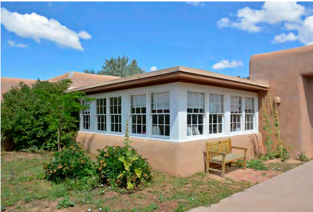
14. Courtyard, south elevation, circa 1950 New Office addition, photographer facing northwest.
