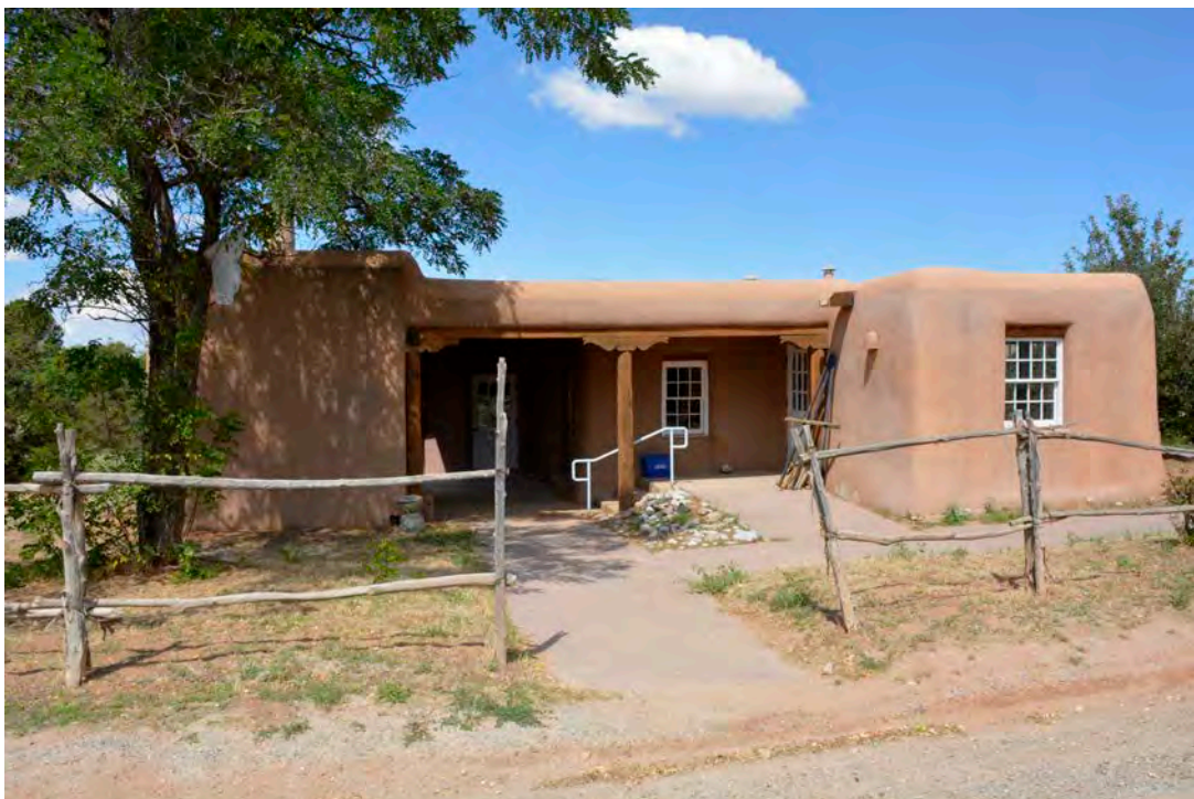
8. East elevation, south end, Garage #1 at right, photographer facing northwest.
