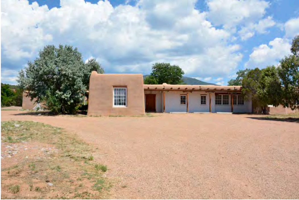
1. Setting and west (main) facade, photographer facing east.
