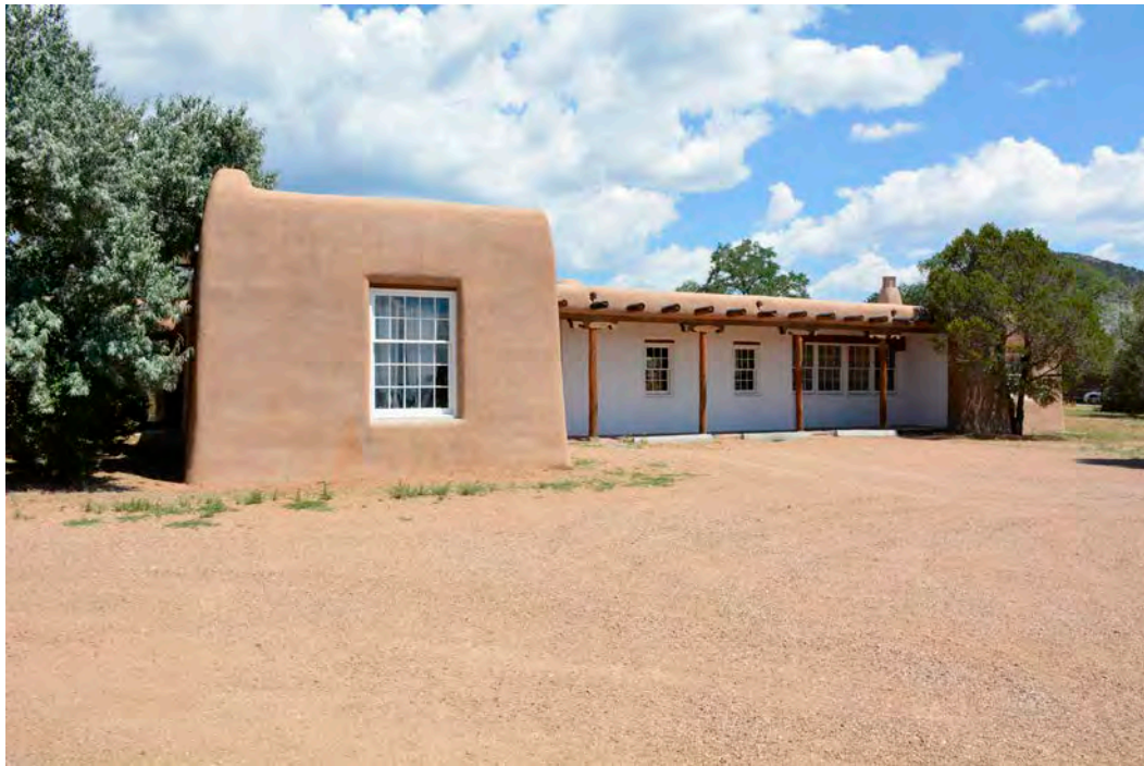
2. West (main) façade, photographer facing southeast.
