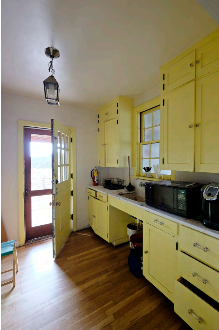
23. Kitchen, photographer facing northeast.
