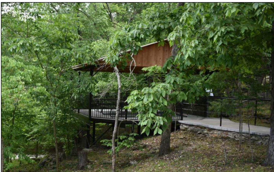
Figure 33: Overlook Platform (2015) Non-Contributing Structure. Image taken by Michelle Diedrich, Spring 2017.
