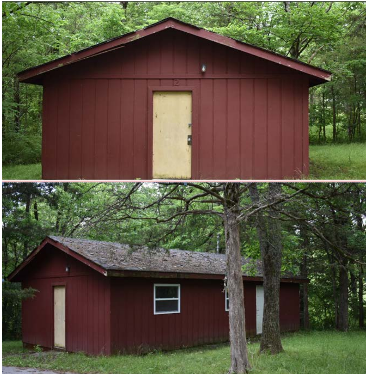
Figure 20: Front and Side View of c. 1980 Church Cabin #2, Non-Contributing Building. Image taken by Michelle Diedrich, Spring of 2017.
