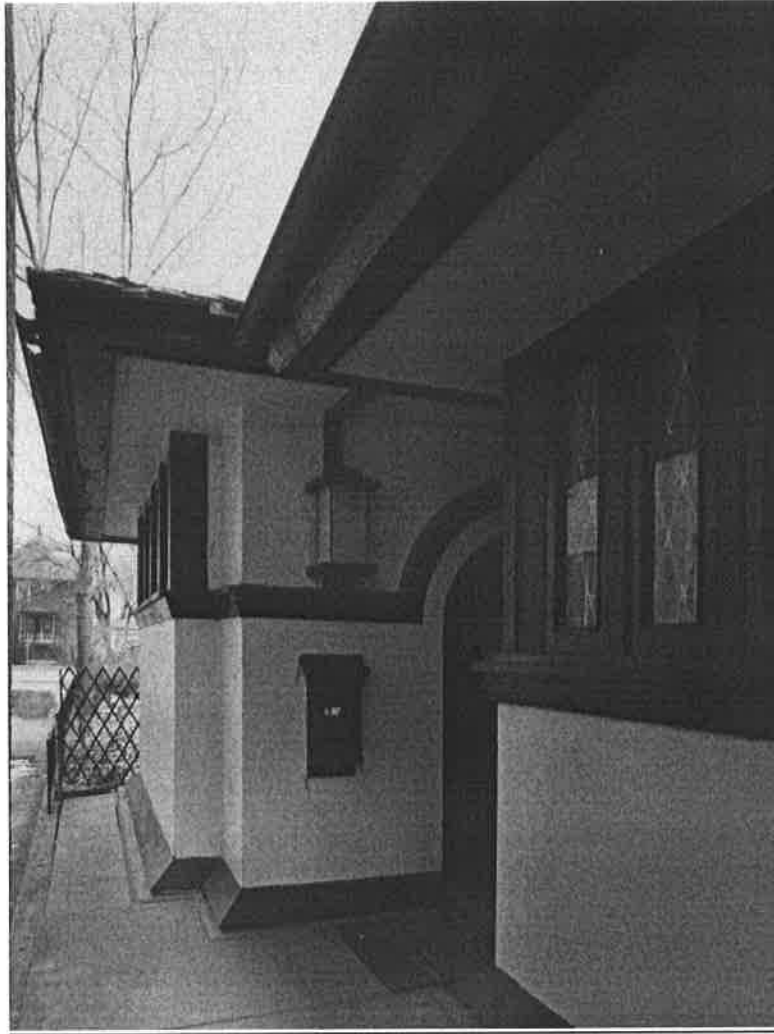
Figure 22 View of Walser House, looking west toward entrance, 1981. Source: Commission on Chicago Landmarks, 33 N. LaSalle Street, Suite 1600, Chicago, IL 60602
