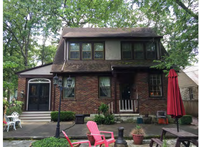
North (back) side
