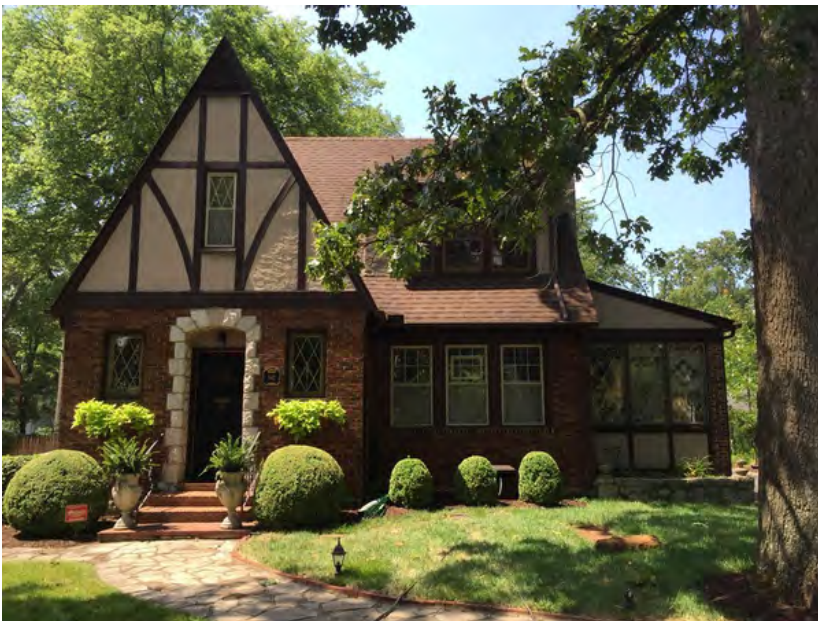
Front (South) side
