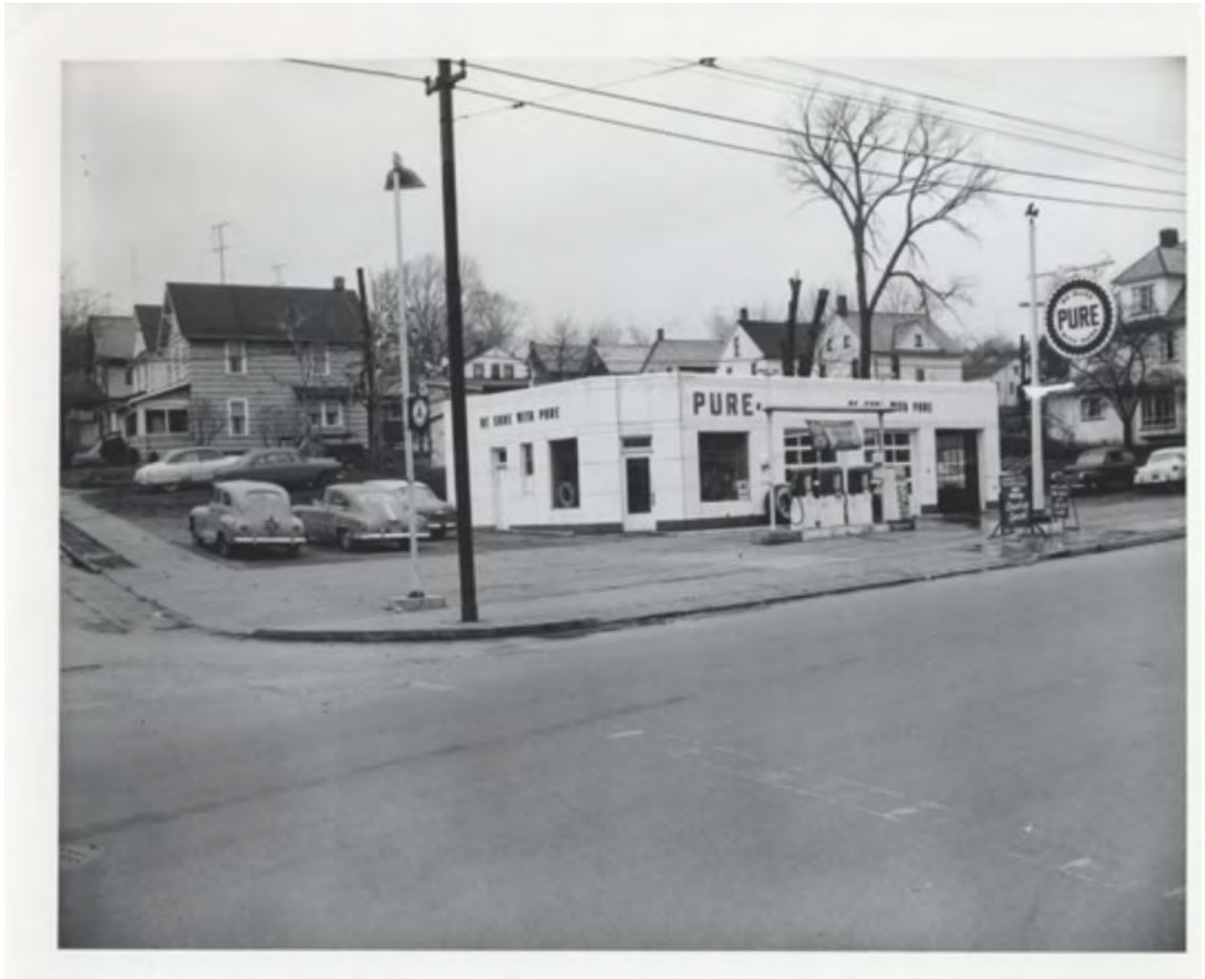
Figure 25. Photo showing 933 Kenmore Blvd. Photo taken aprx. 1950s.
