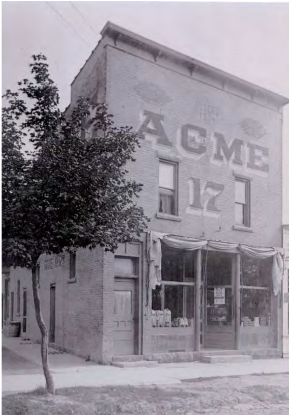
Figure 29. Photo showing 964 Kenmore Blvd. Photo taken aprx. 1905.
