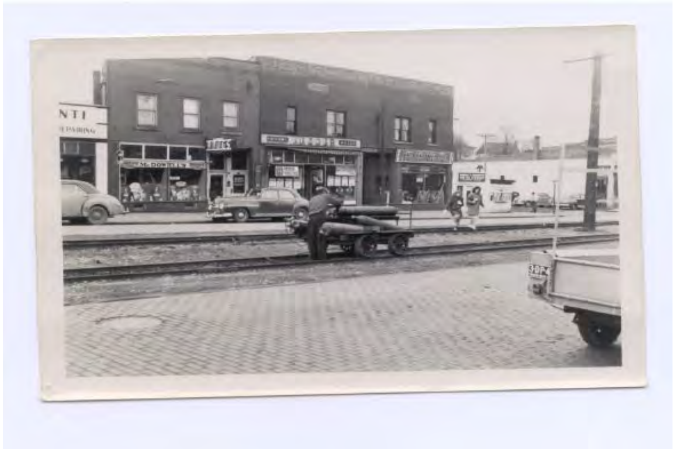
Figure 31. Photo showing 980-984 Kenmore Blvd. Photo taken aprx. 1940s.
