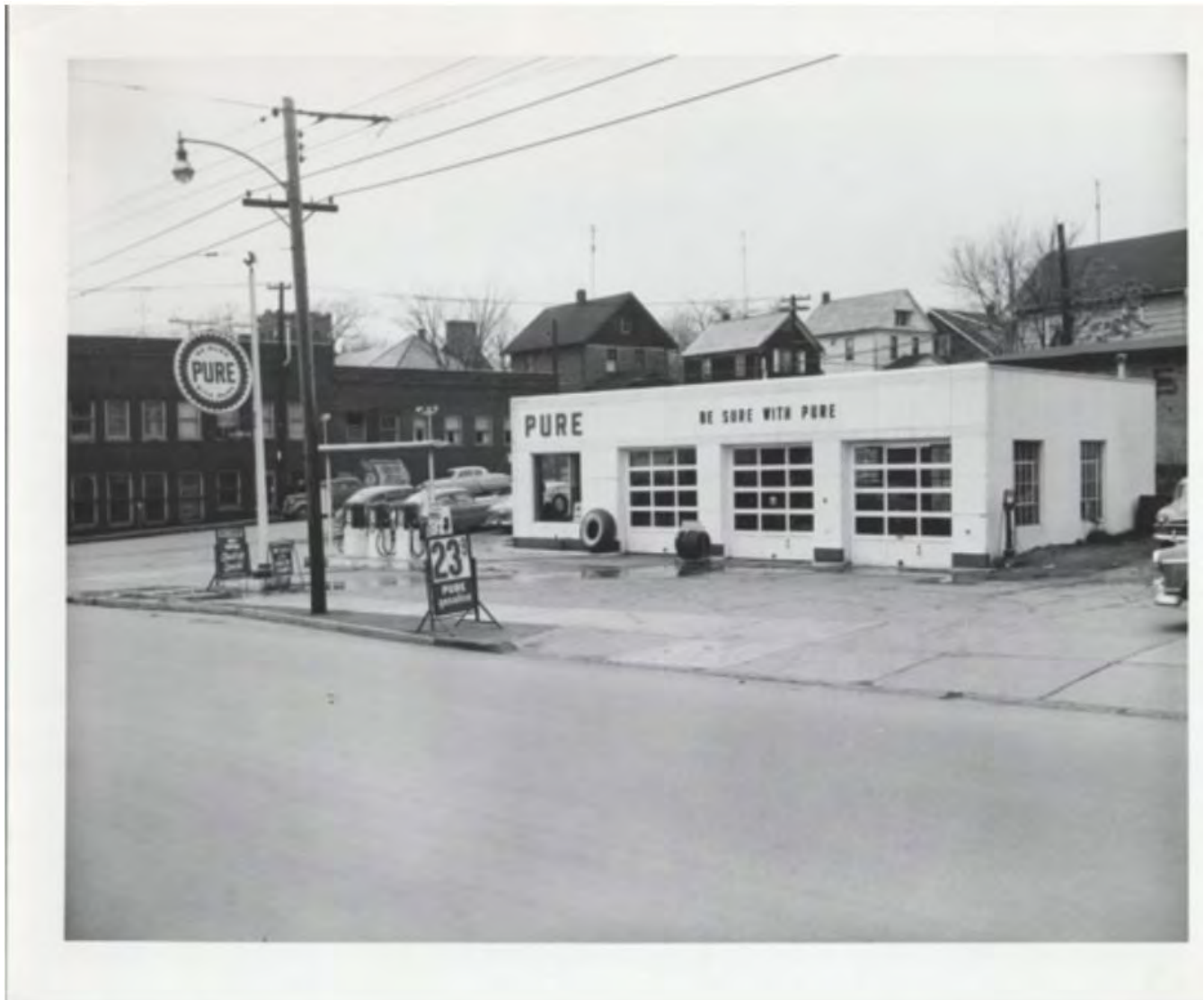
Figure 24. Photo showing 933 Kenmore Blvd. Photo taken aprx. 1950s.
