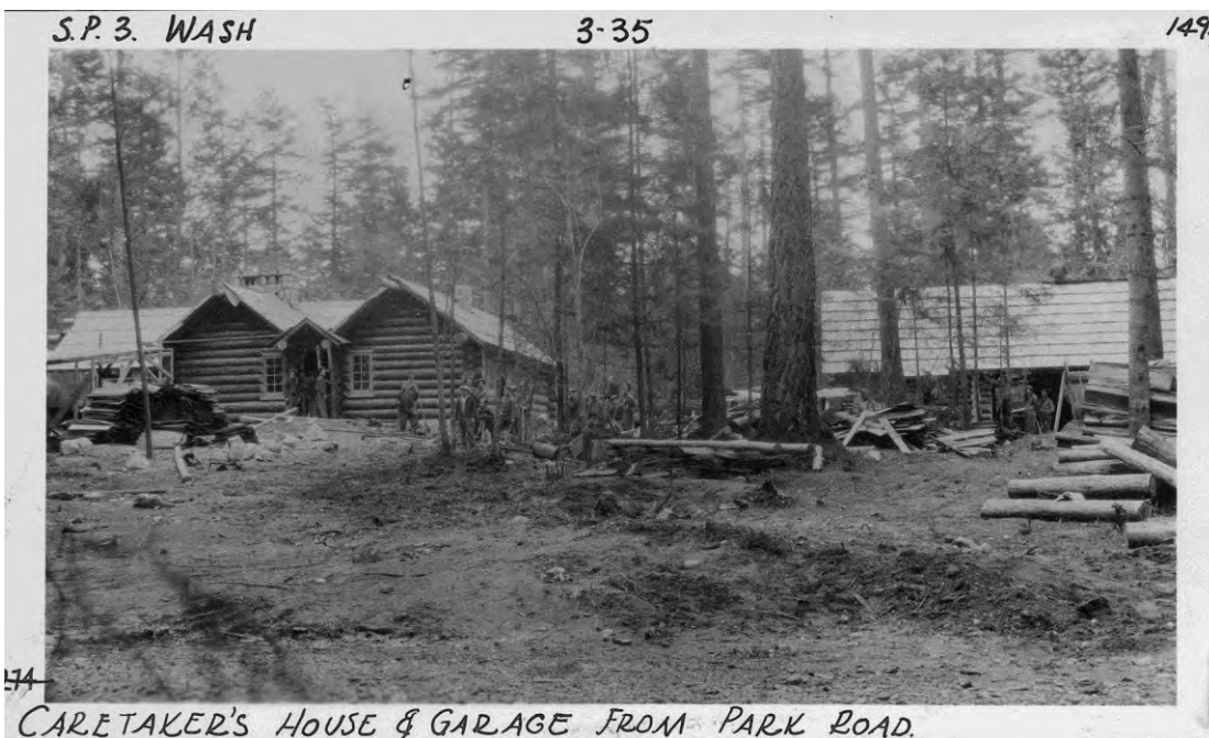
Caretaker's Residence (ID#1) and Garage (ID#2) nearly complete, view to east.
