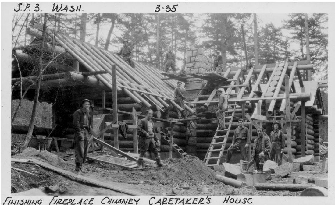
240 PLACING RAFTERS CARETAKER'S HOUSE Placing rafters on Caretaker's Residence (ID#1), view to southeast.
