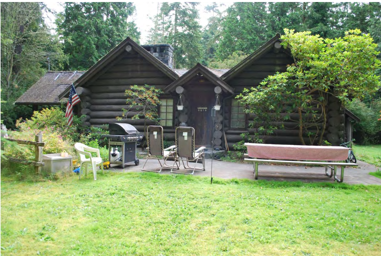
Photo 1 of 8: Cranberry Lake Caretaker's Residence (ID#1), view to east taken 8/1/2012.
