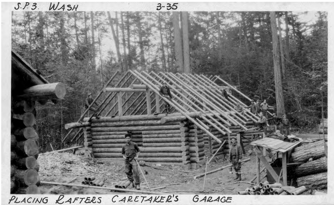
Placing rafters on Caretaker's Shop and Garage (ID#2), view to southeast.
