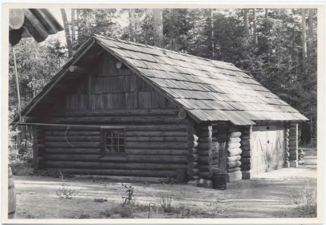
Caretaker's Shop and Garage (ID#2) completed, view to southeast.
