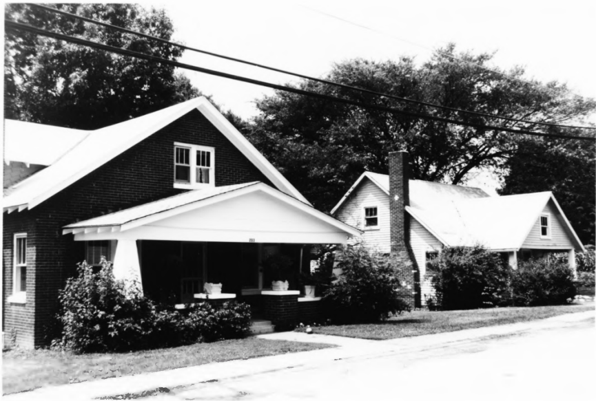
Old Town Historic District; Hartford, Ohio Co., KY Photo 9
