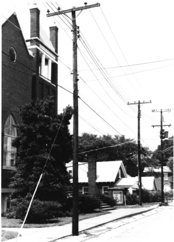
Old Town Historic District; Hartford, Ohio, 1944 Photo 8
