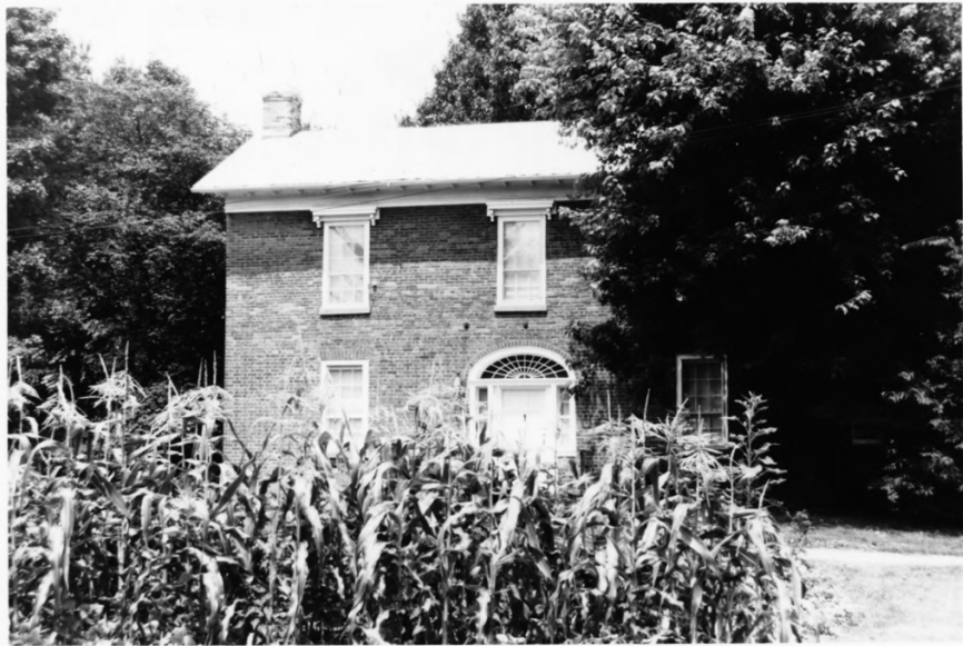
Old Town Historic District, Hartford, Ohio Co., KY Photo 10
