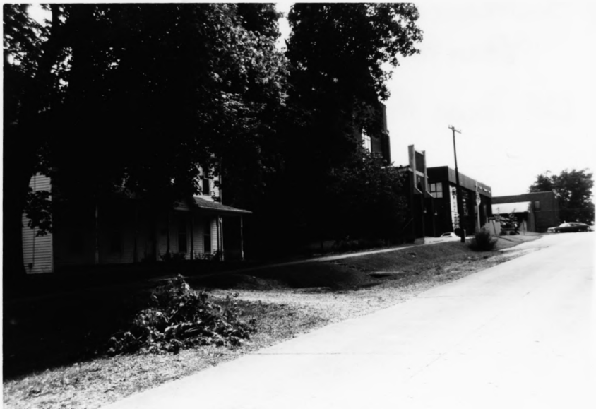
Old Town Historic District Hartford, Ohio Co., Ky Photo 3
