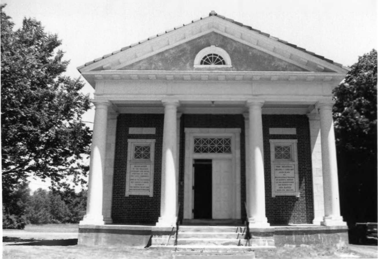
ASA BATES MEMORIAL CHAPEL; SOMERSET CO., MAINE
