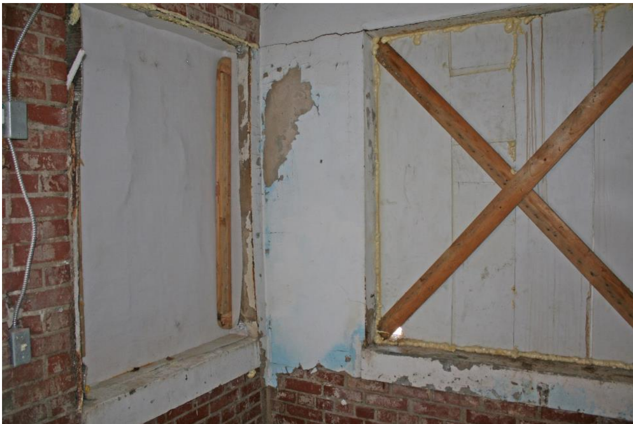
15 of 19. Section C (office); camera looking northwest.
