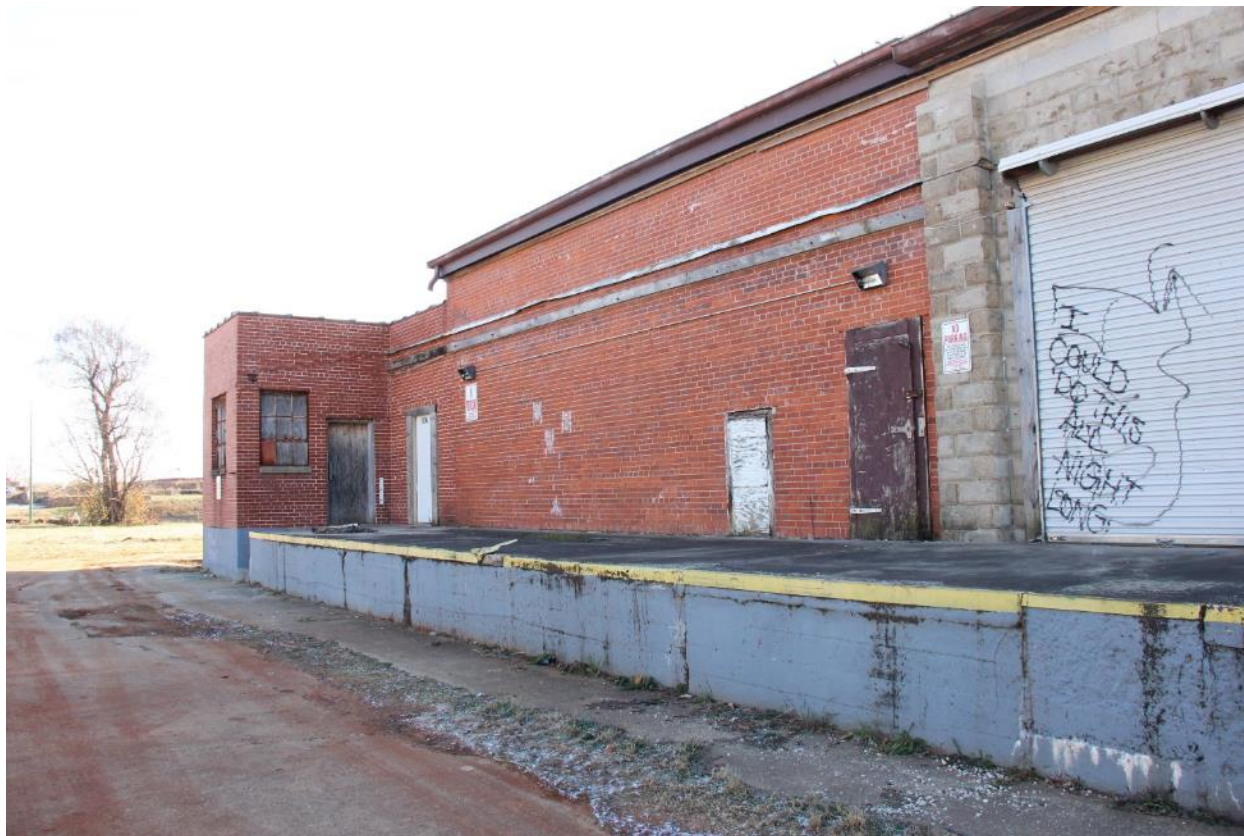
4 of 19. Front, north wall and loading dock; camera looking east-southeast.
