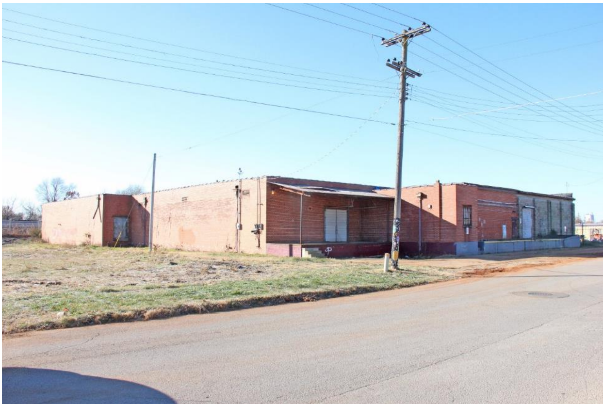
1 of 19. Front, northeast corner; camera looking southwest.
