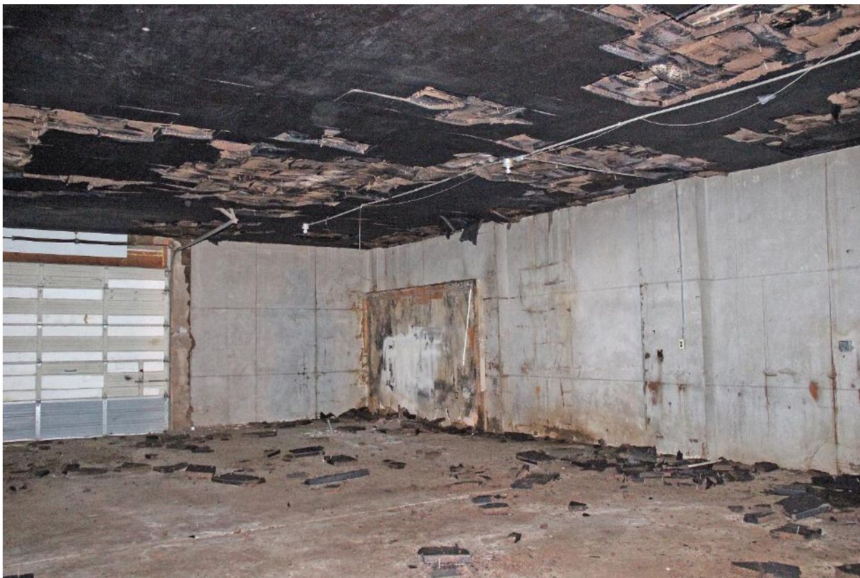
17 of 19. Section D; camera looking west.
