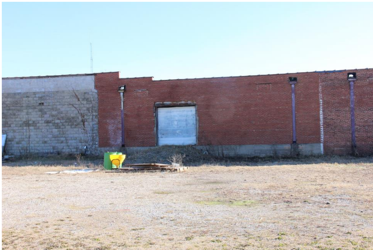
8 of 19. Center of west wall; camera looking east.
