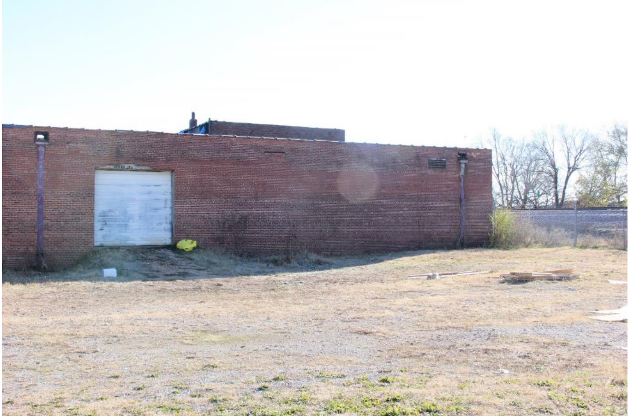
9 of 19. South end of west side wall; camera looking east.
