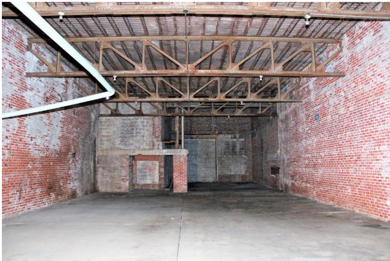
13 of 19. Section B; camera looking south.
