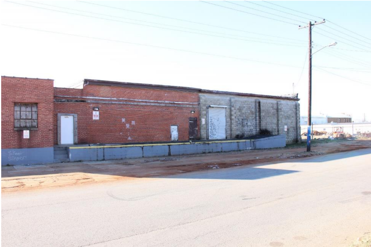
5 of 19. West end of front (north) wall; camera looking south.
