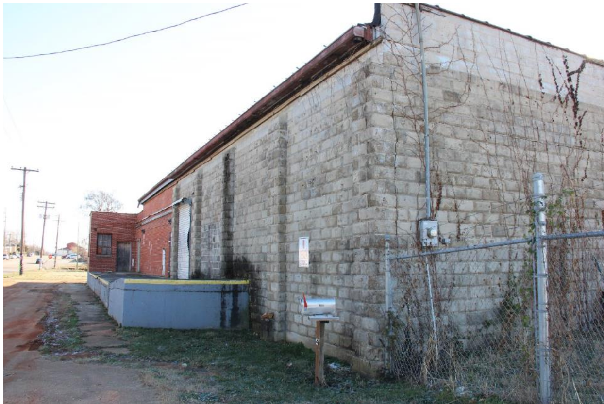
6 of 19. Northwest corner; camera looking southeast.
