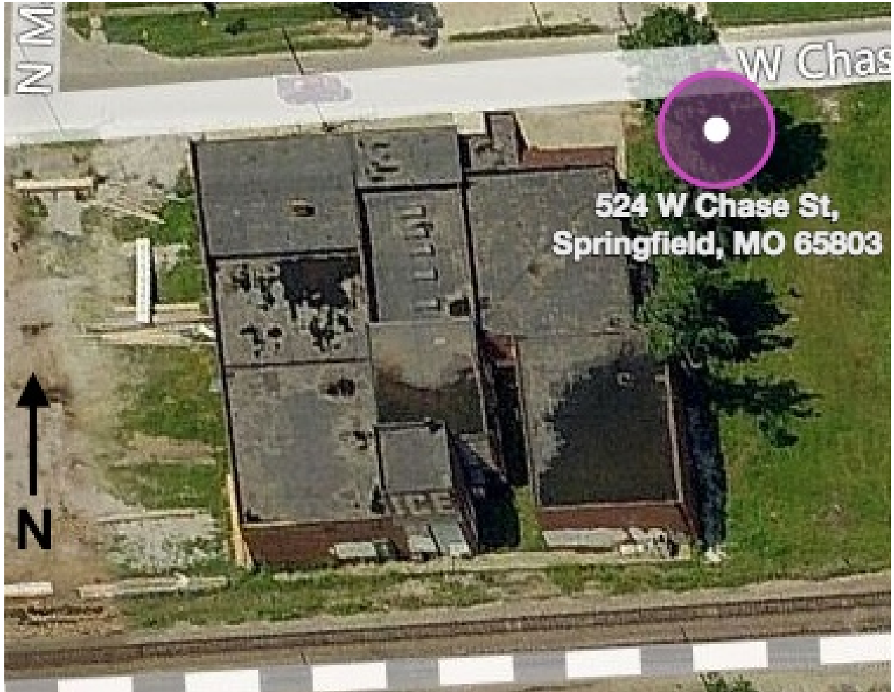
Figure 5. Aerial view of rear of building from https://www.bing.com/maps . Accessed 5 July 2017.
