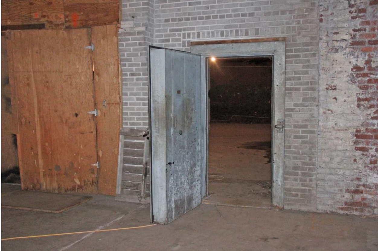
12 of 19. Section B; camera looking northeast to original door.
