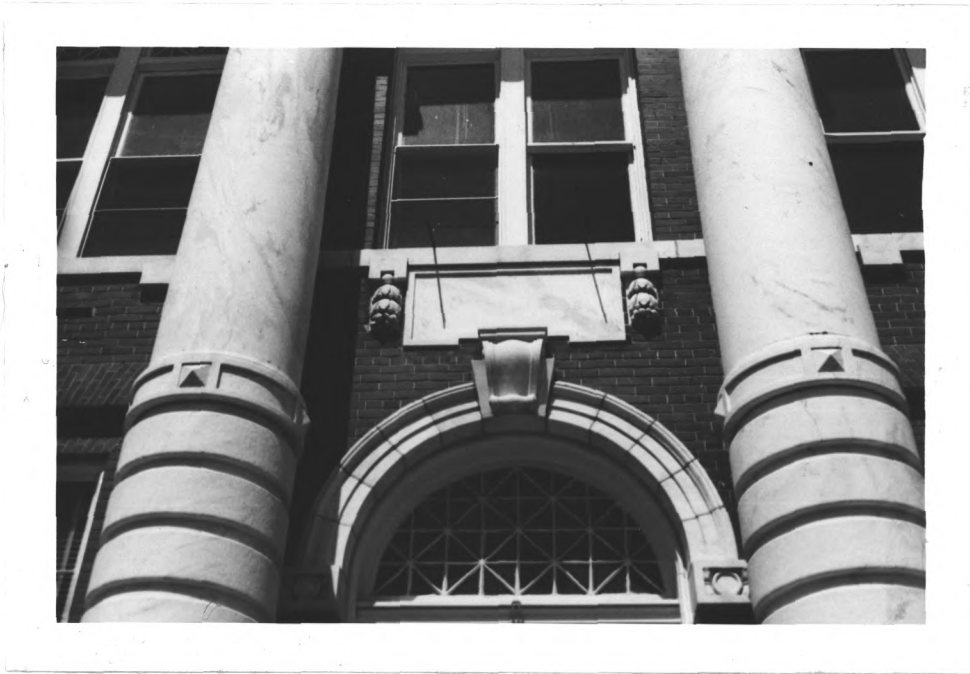
DETAIL - BANDED COLUMNS
