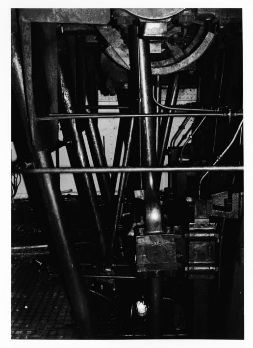
TUGBOAT HERCULES, SAN FRANCISCO, CA VIEW OF HER TRIPLE - EXPANSION STEAM ENGINE , SHOWING CRANKSHAFT, PISTON RODS, AND CAMSHAFTS FEBUARY 1985 N. P. S. PHOTO BY STEPHEN A HALLER NEGATIVE ON FILE AT GOLDEN GATE N.R.A.
