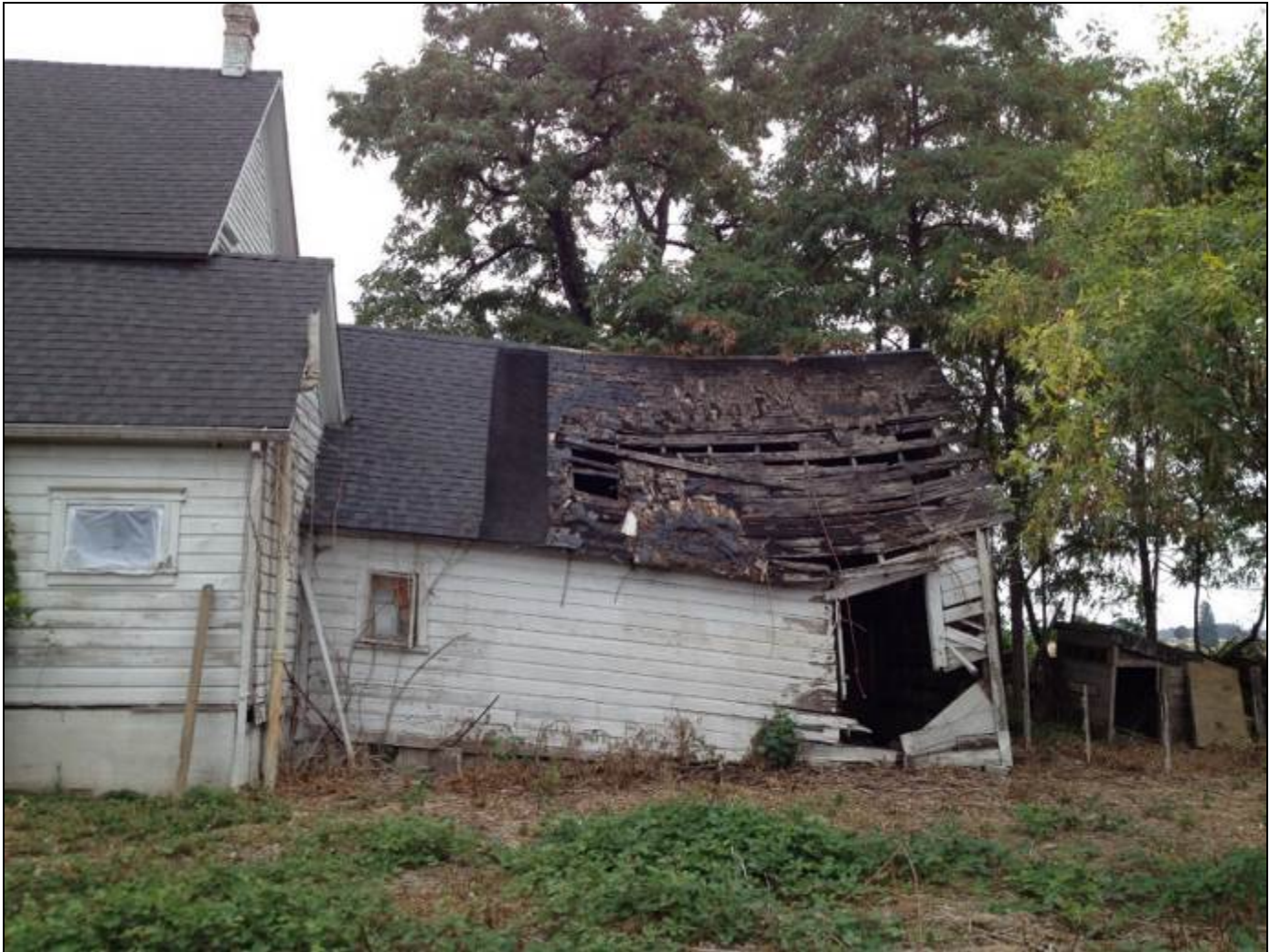
Figure 22: Woodshed addition replaced in 2016 (see Photo 4)
