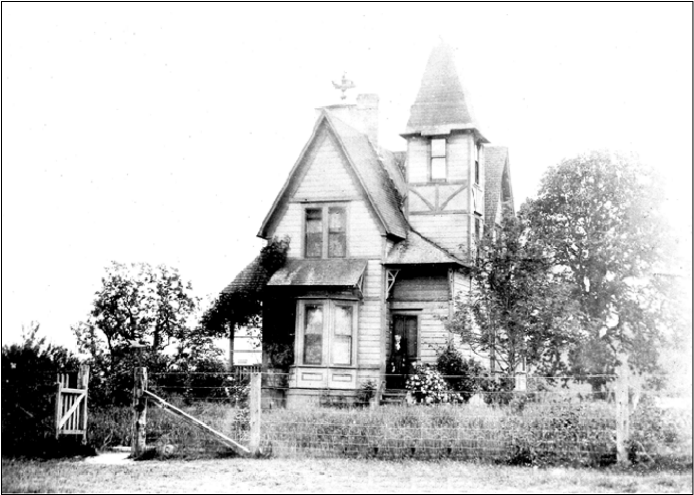
Figure 10: Historical photo of the farmhouse taken sometime between 1892-1911, looking south
