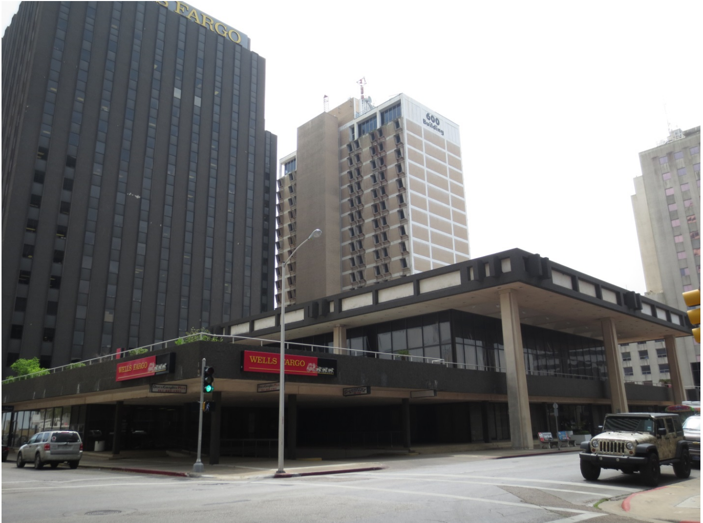
Photo 6 Oblique northwest corner
