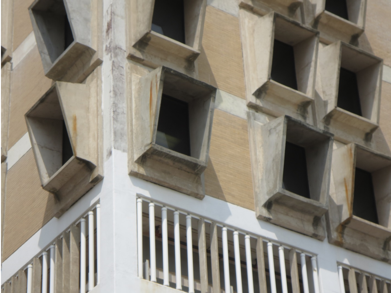
Photo 12 Close-up oblique, southeast corner
