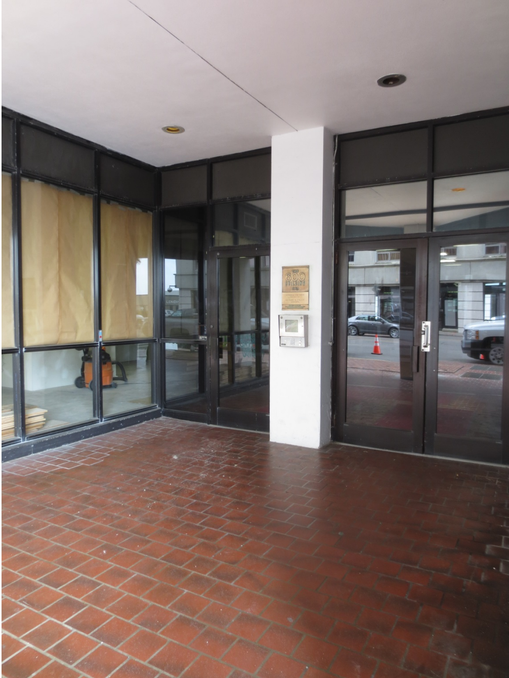
Photo 9 Entryway south elevation
