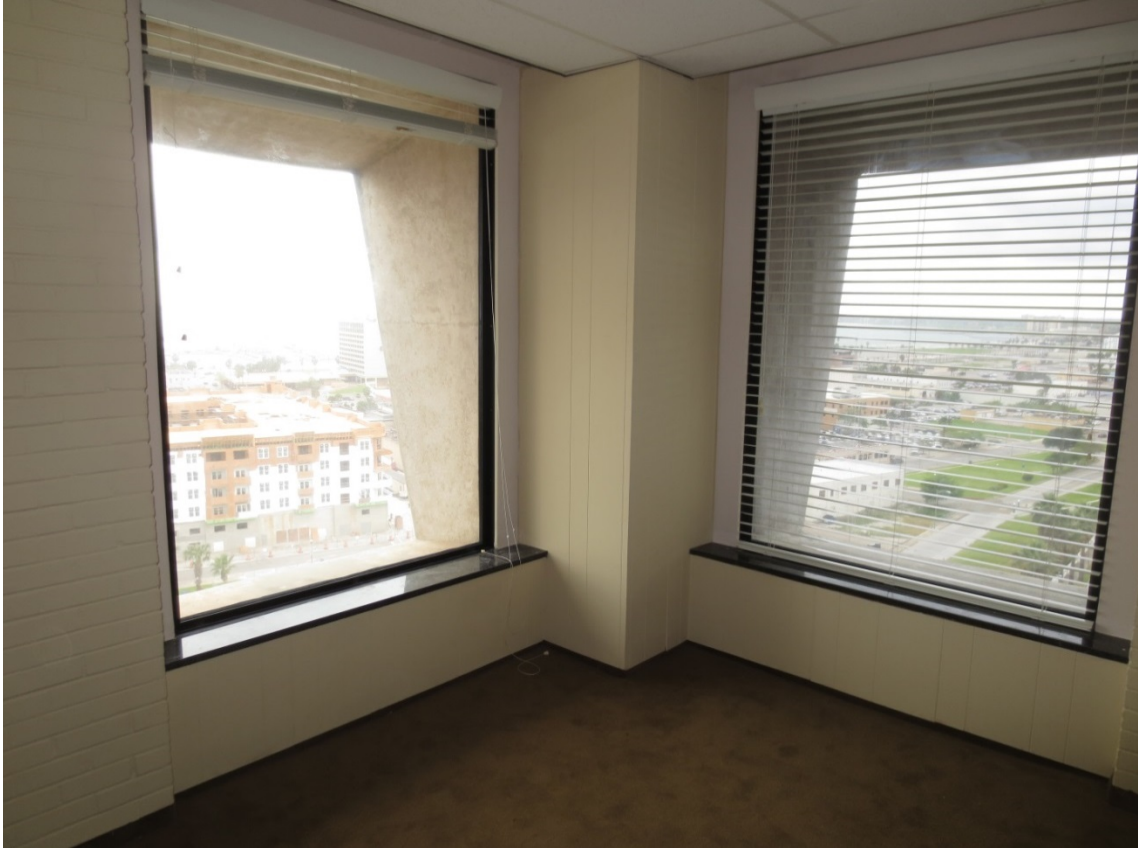
Photo 22 Typical interior window
