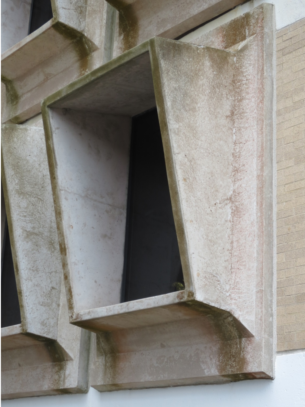
Photo 10 Close-up precast concrete sunshade
