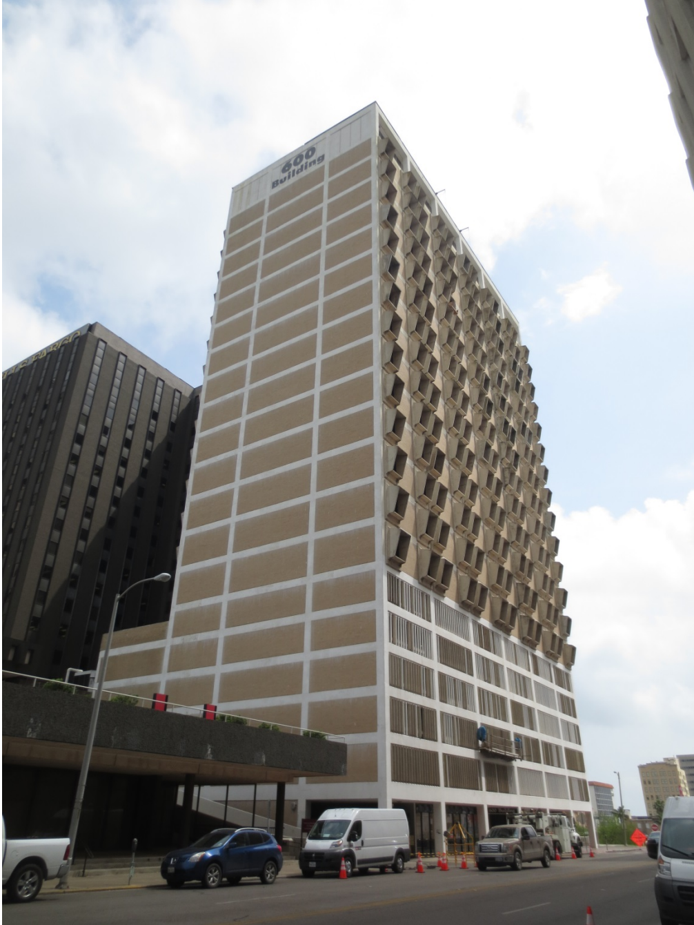
Photo 4 Oblique southwest corner
