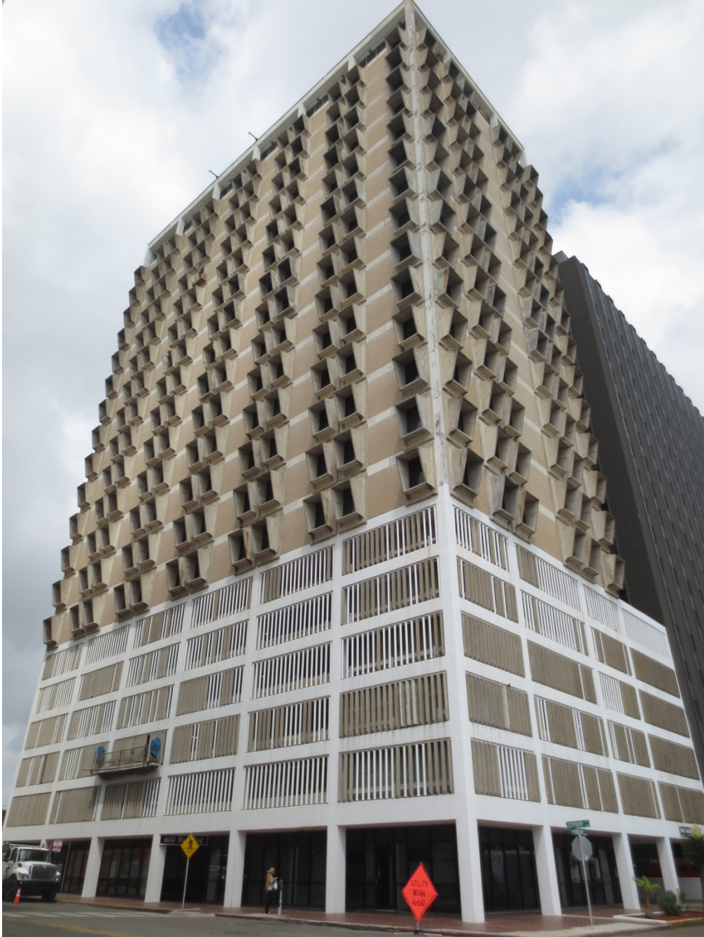
Photo 3 Oblique southeast corner
