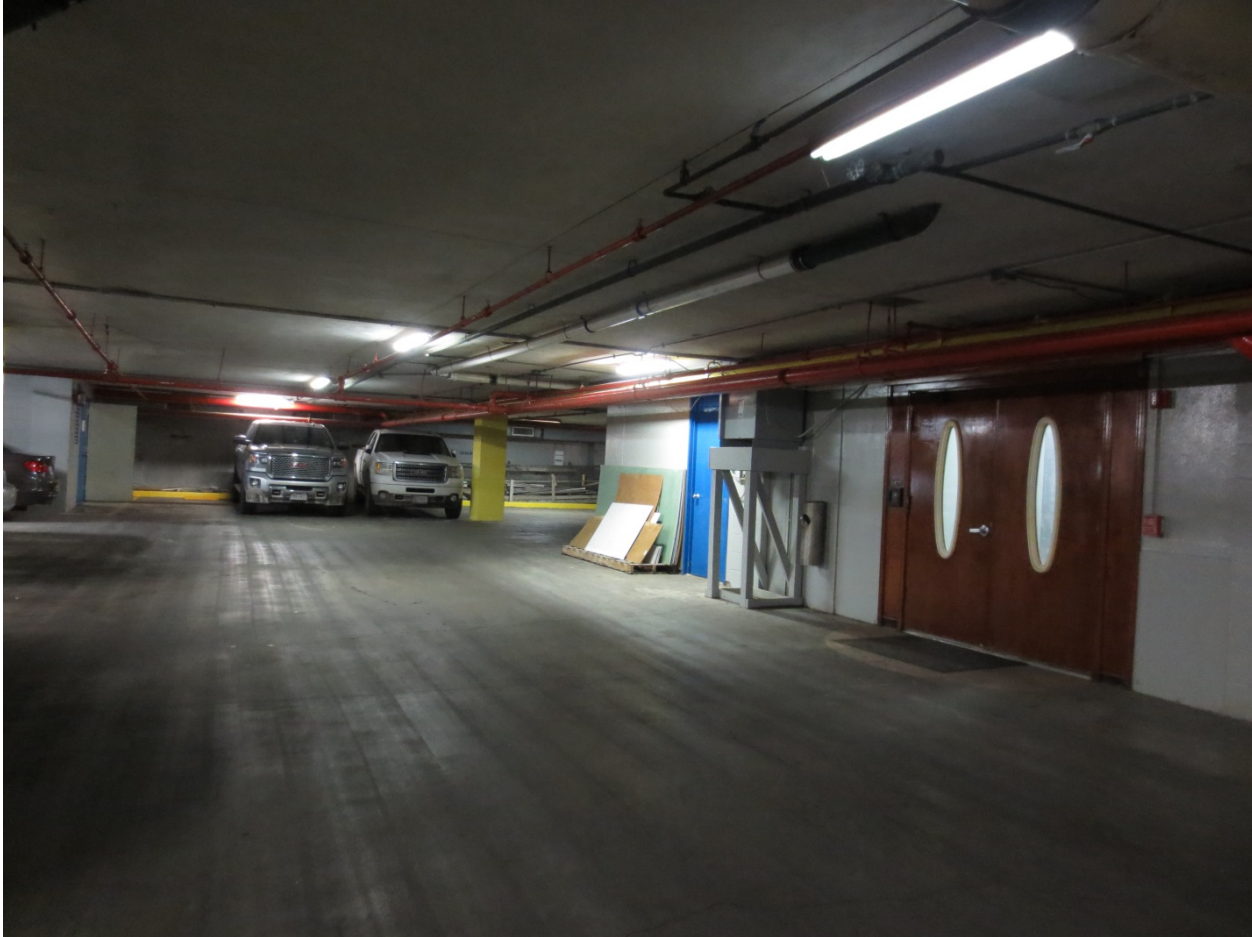
Photo 15 Typical parking garage floor
