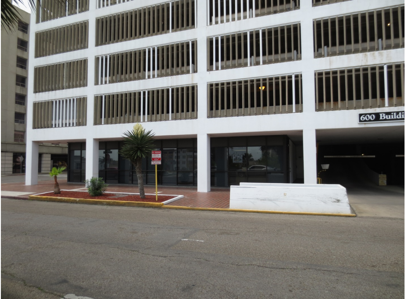
Photo 8 Ground floor of east elevation
