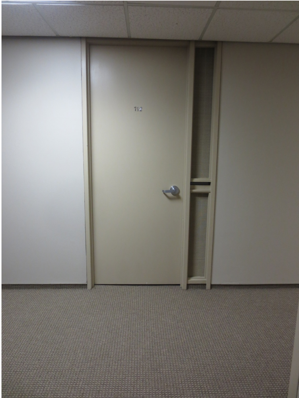
Photo 20 Typical office entry door from corridor
