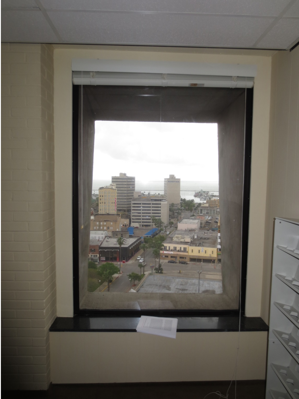
Photo 21 Typical interior window
