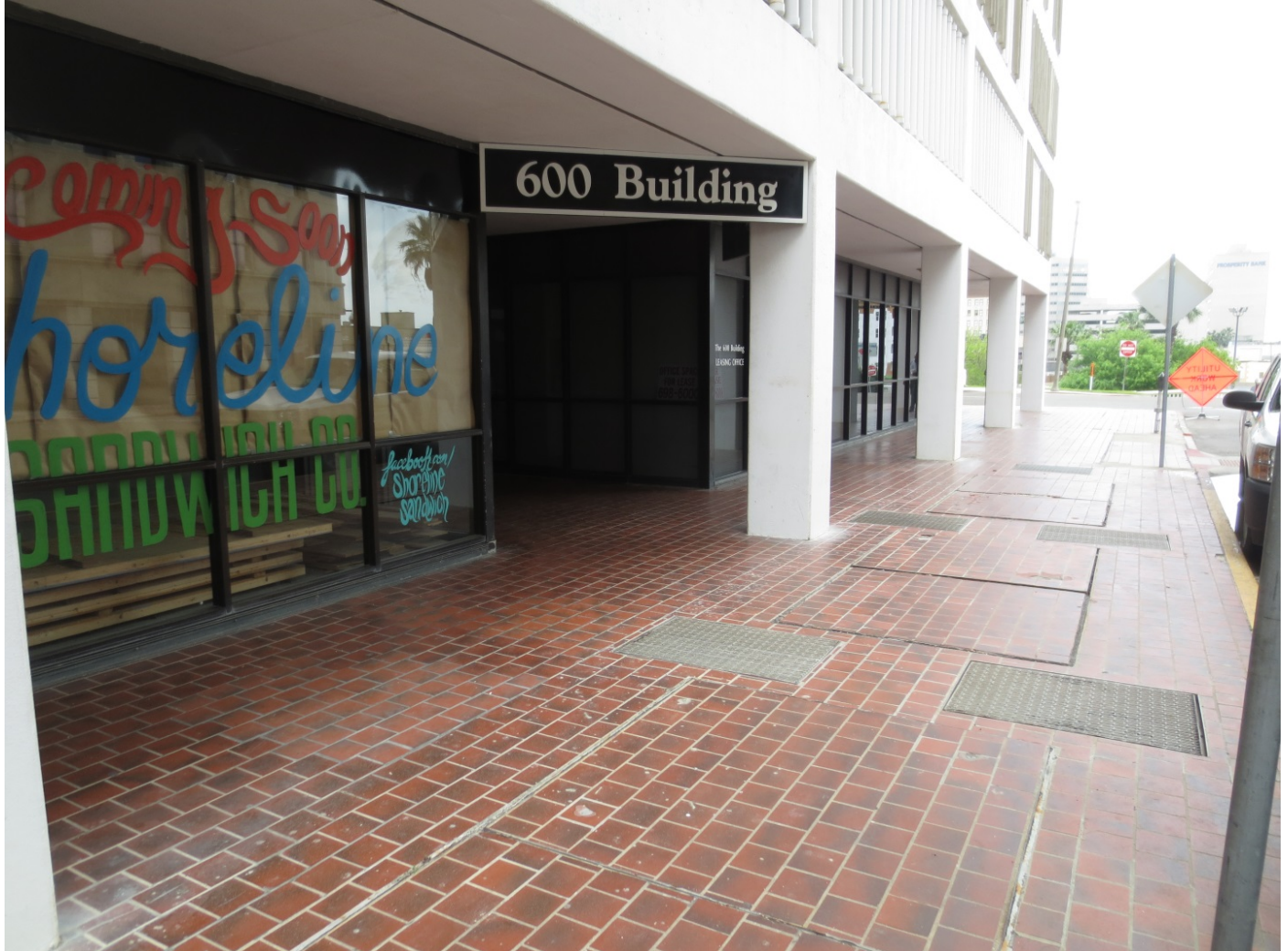
Photo 7 Ground floor of south façade and entryway
