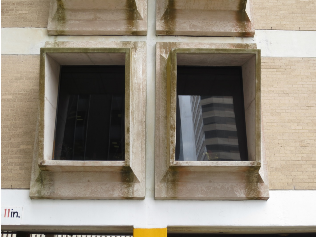
Photo 11 Close-up pair of precast concrete sunshades
