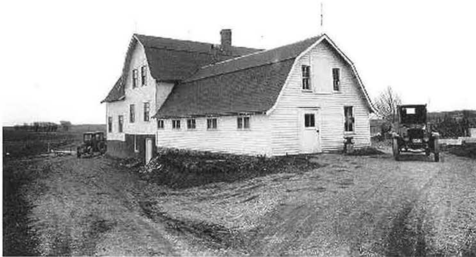
Figure 15: 1924 looking southeast. The new Honey House that incorporated and expanded the old hog barn structure (foreground).
