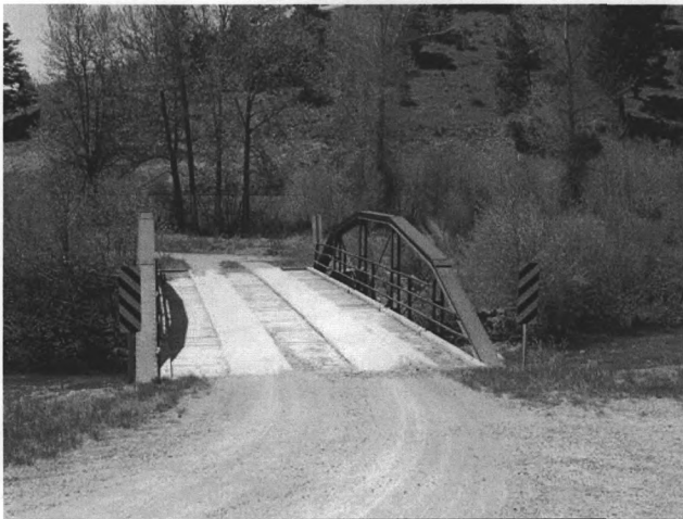
Photograph 0002. Little Blackfoot River Bridge. East portal. View to west.
