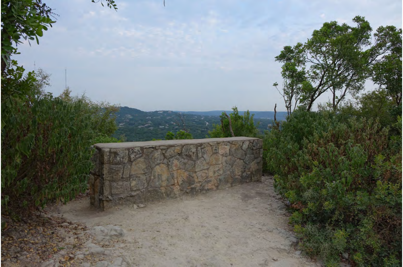
Photo 14 Stone wall on north trail Camera facing west
