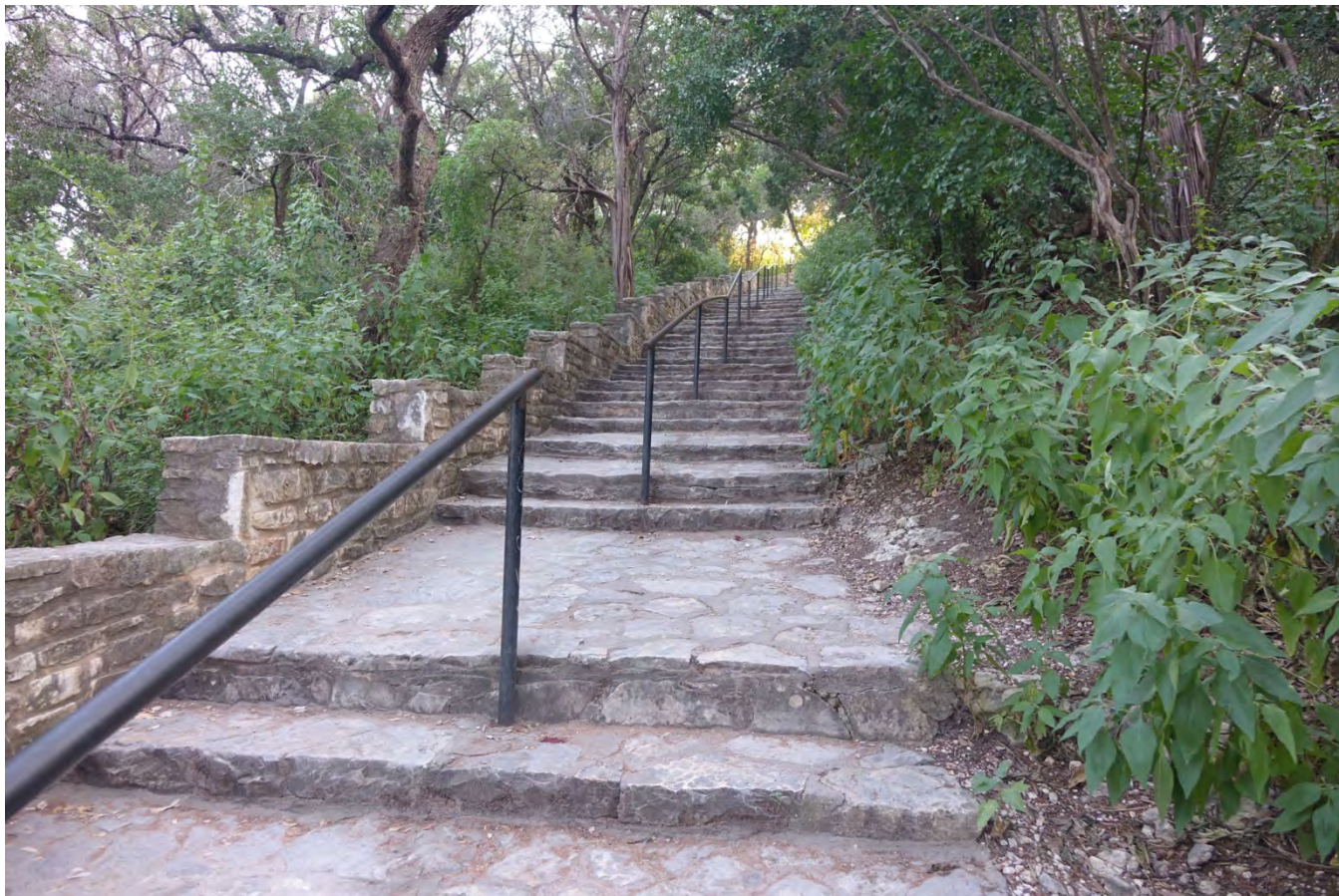
Photo 3 Staircase, looking up from street level Camera facing west
