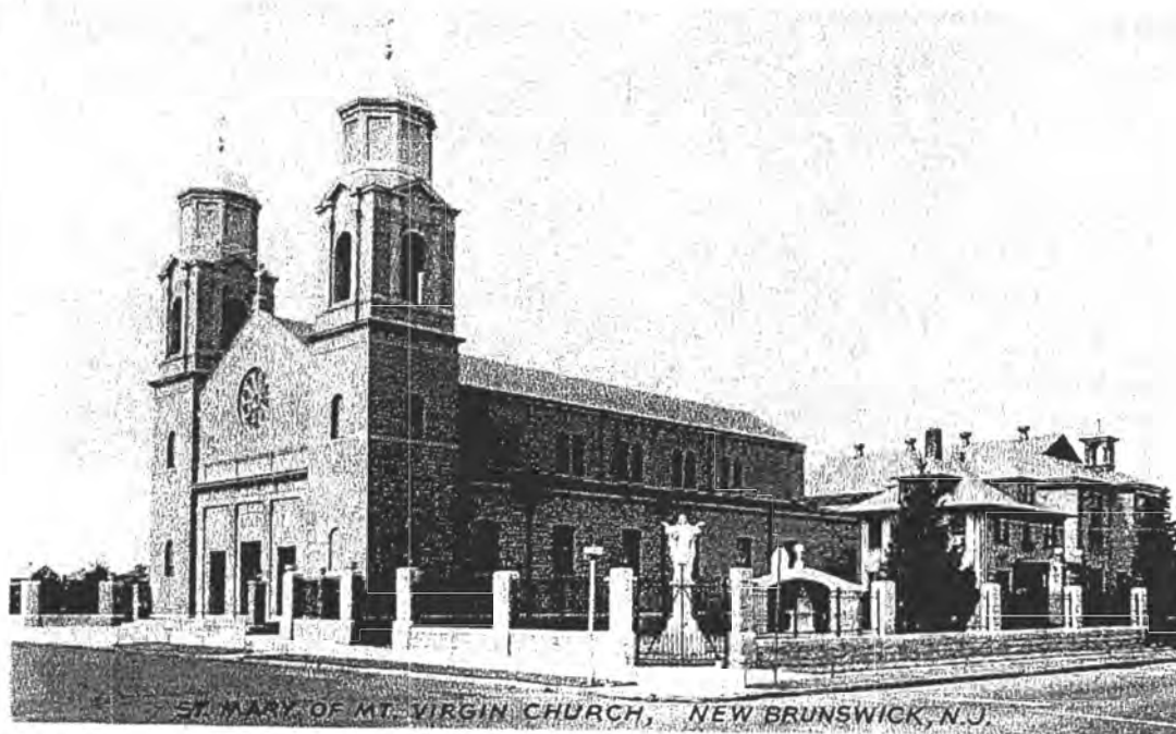
Historic Photograph 3 of 5. Exterior view of St. Mary of Mount Virgin Church, taken in the late 1950s after the parish obtained title to the two corner lots fronting on Remsen Avenue, fenced the grounds, and created outdoor sculpture gardens on either side of the church. Courtesy of the New Brunswick Free Public Library, New Brunswick, NJ.
