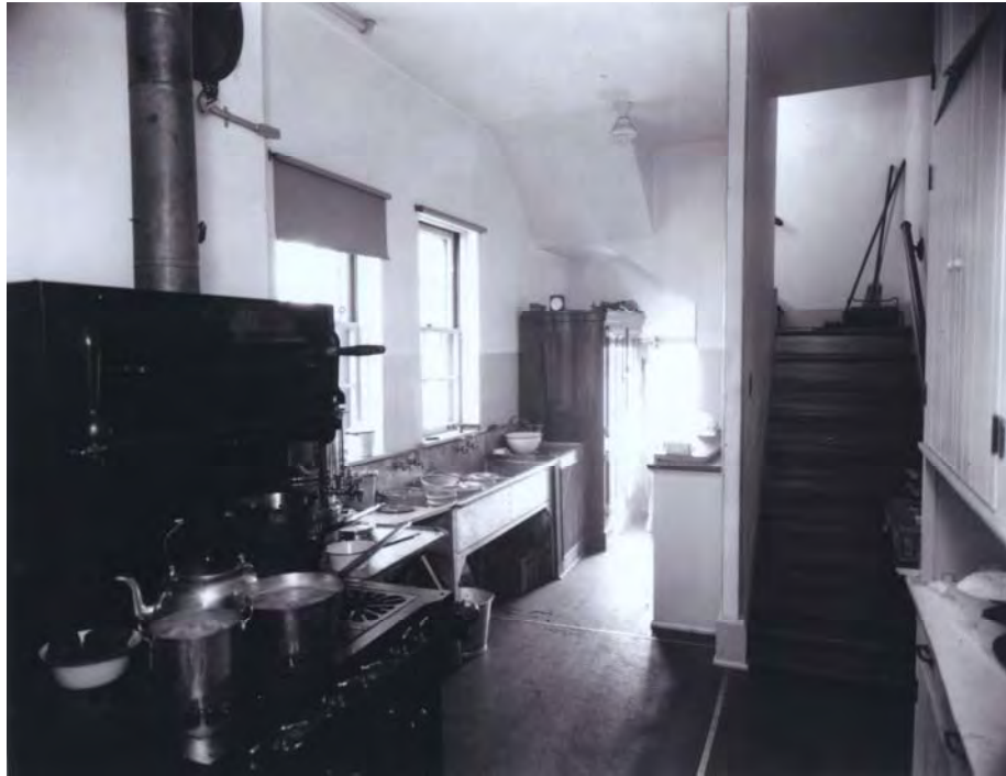
Figure 10: Interior, Kitchen, 1925, camera facing northeast.
