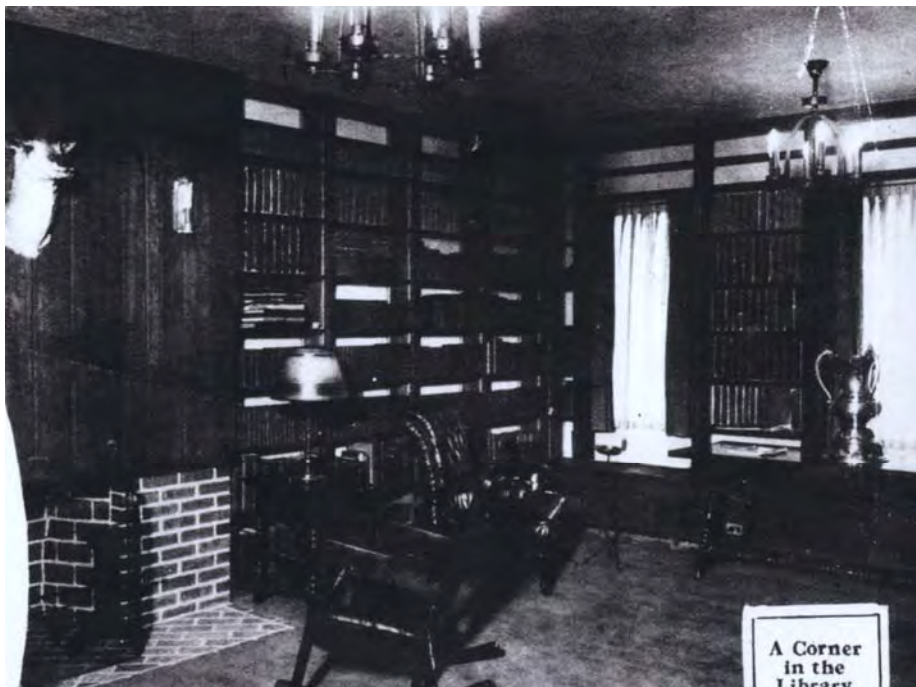
Figure 11: Interior, Library, 1925, camera facing southwest.
