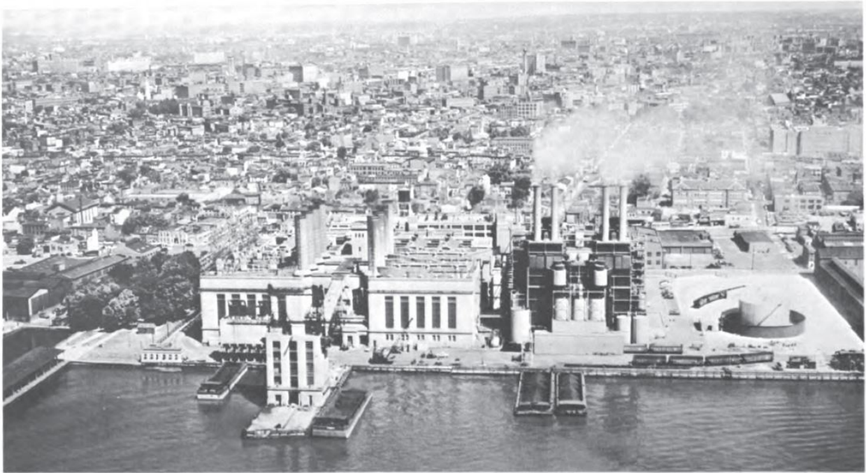
Figure 20 – Aerial view, 1957 (From Wainwright, History of the Philadelphia Electric Company )
