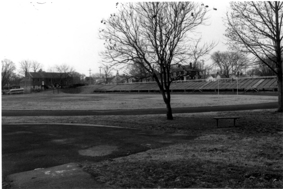
Cameron School Davidson County TN
