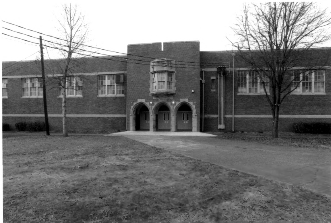
Cameron School Davidson County TN
