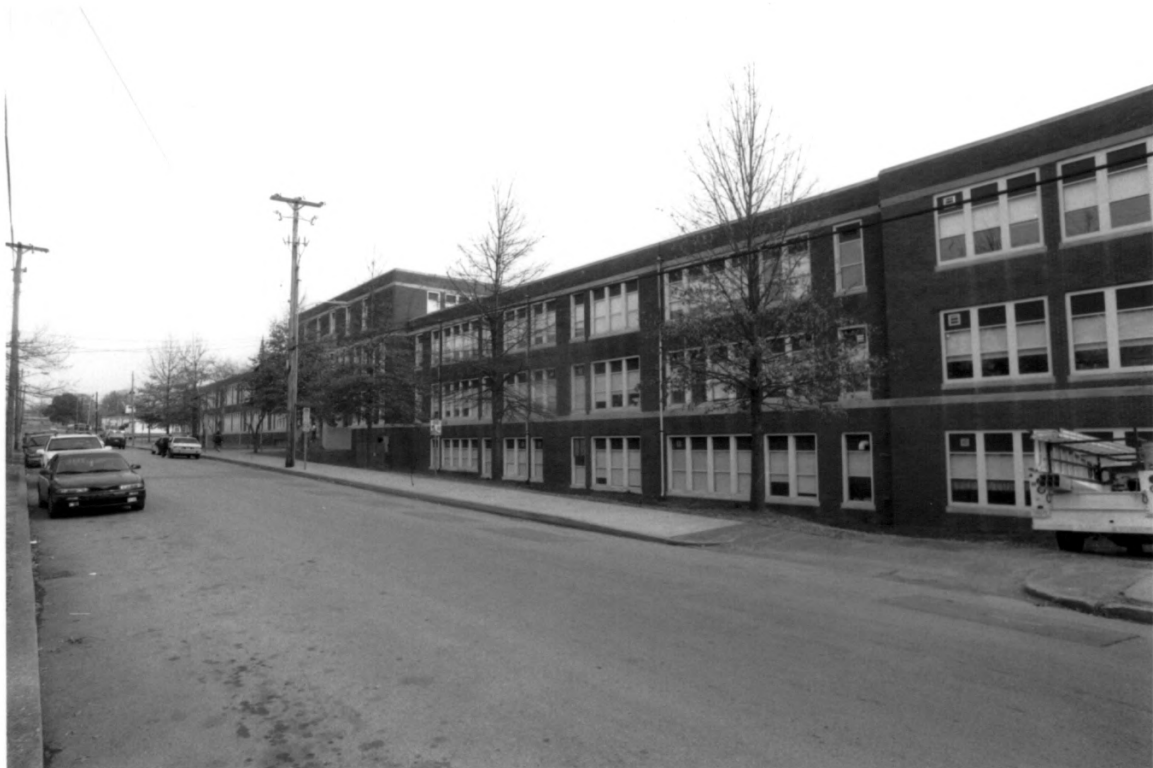
Cameron School Davidson County TN
