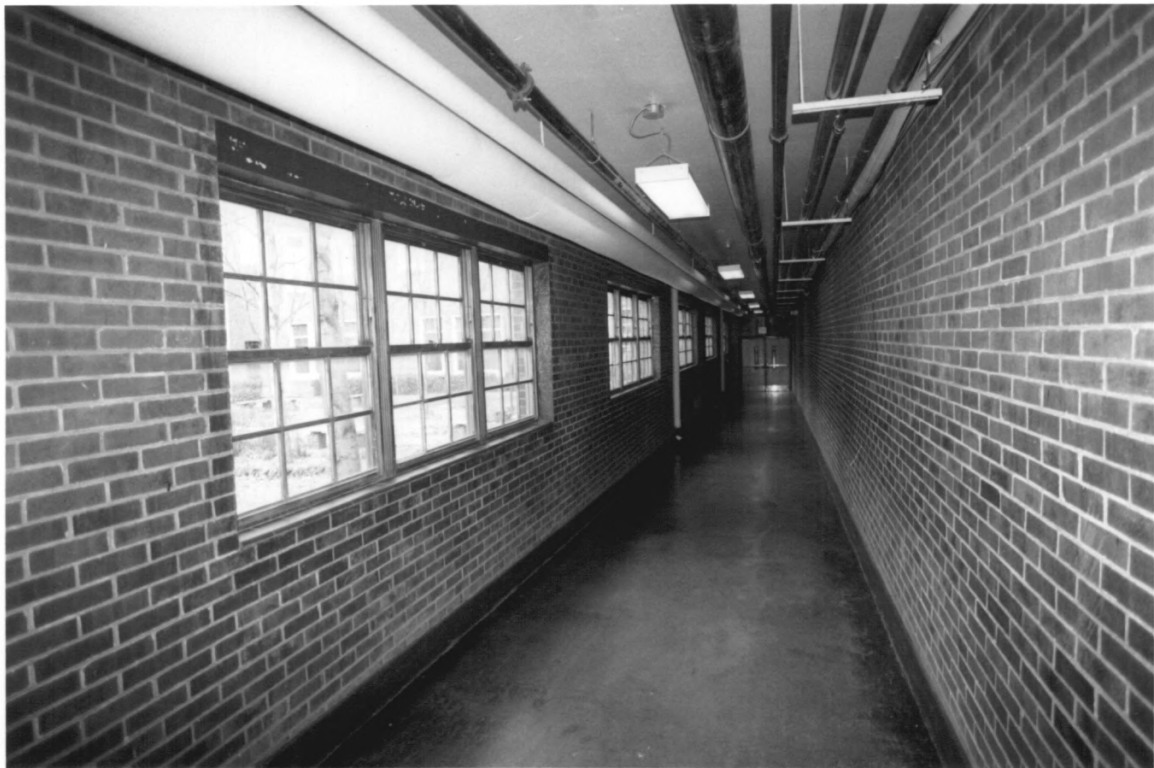
Cameron School Davidson County TN
