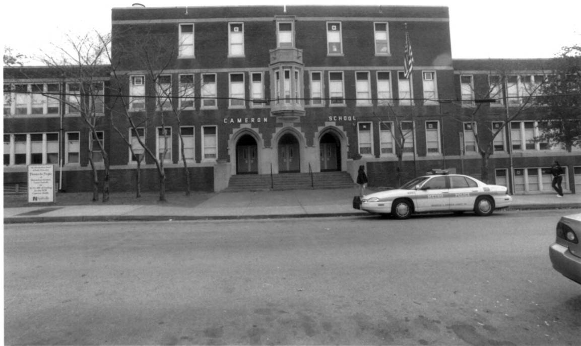
Cameron School Davidson County TN
