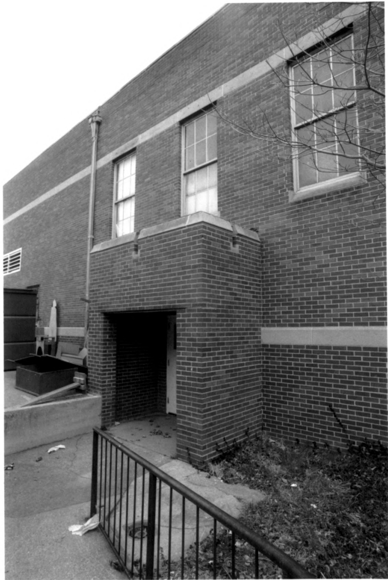
Cameron School Davidson County TN
