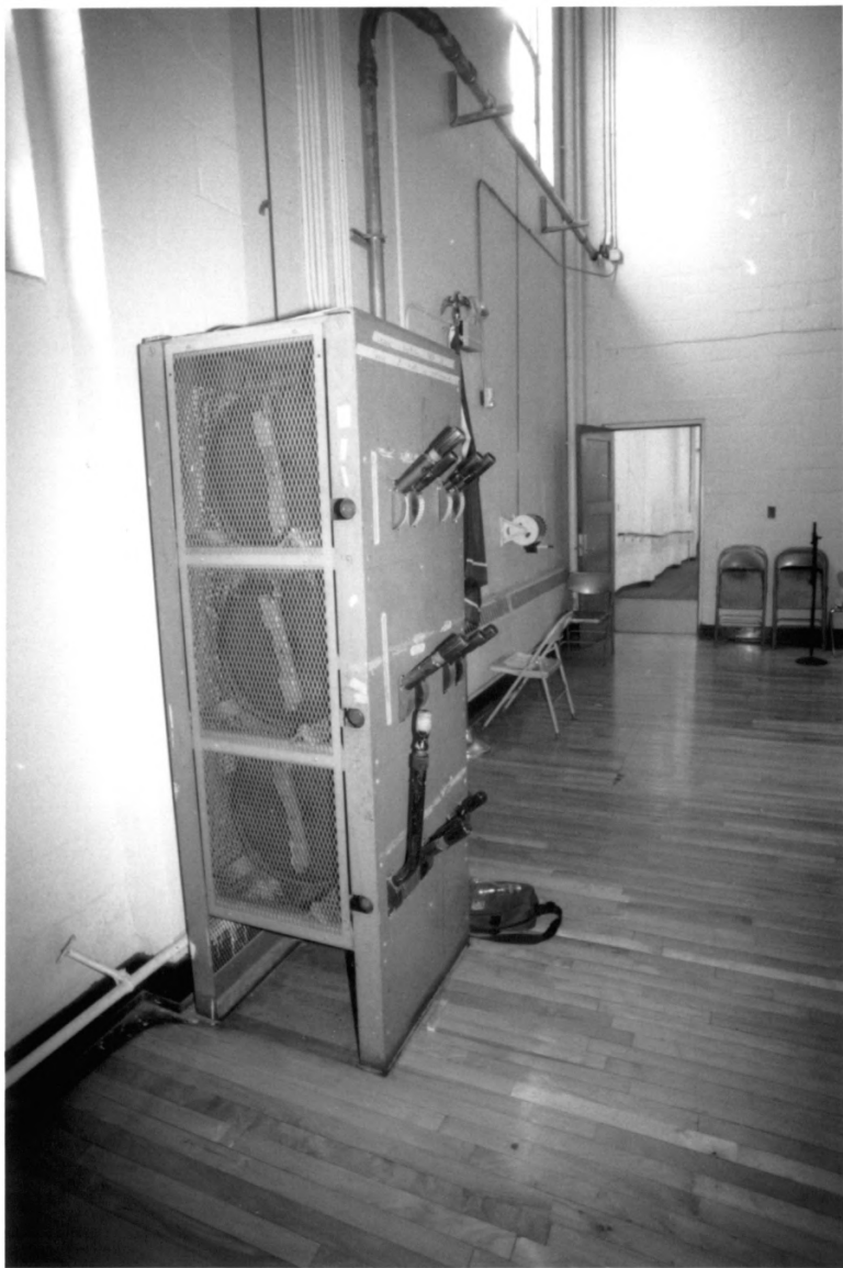
Cameron School Davidson County TN
