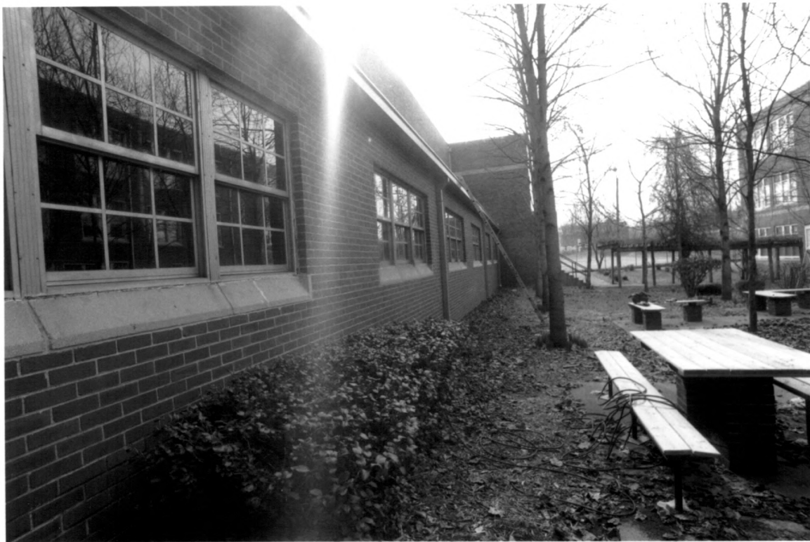
Cameron School Davidson County TN
