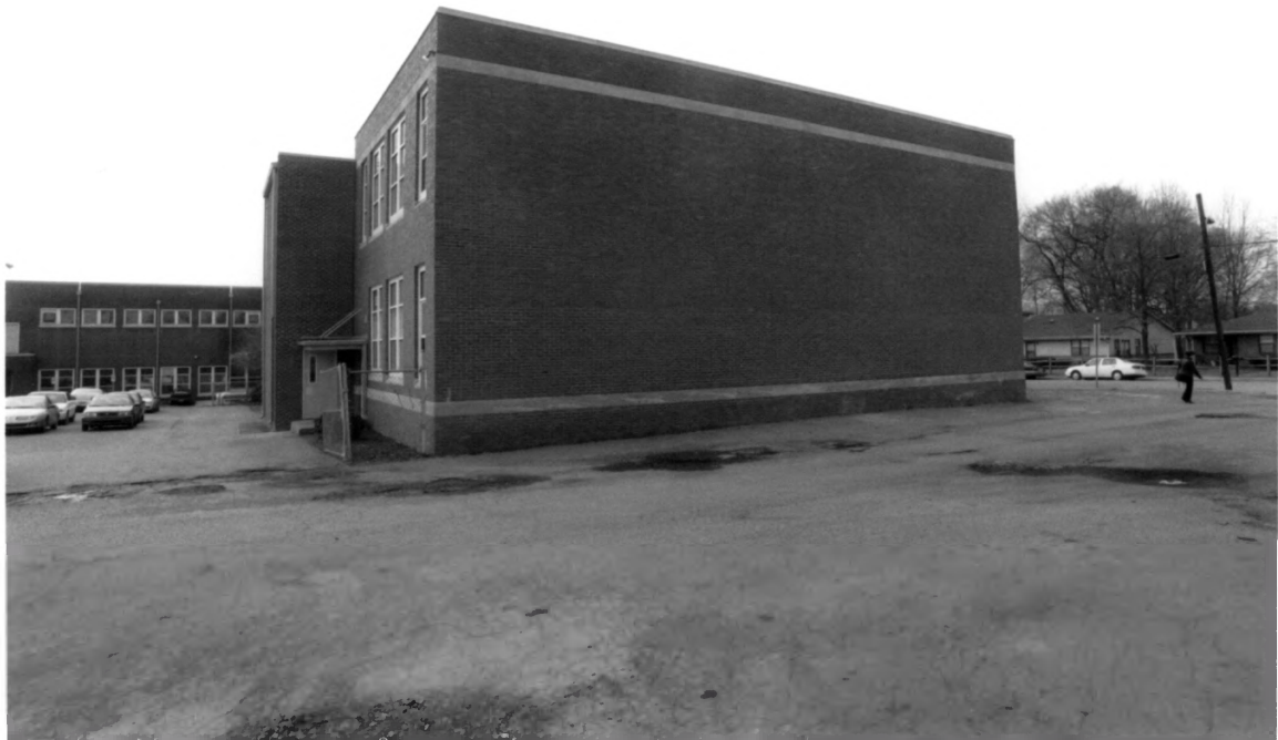
Cameron School Davidson County TN
