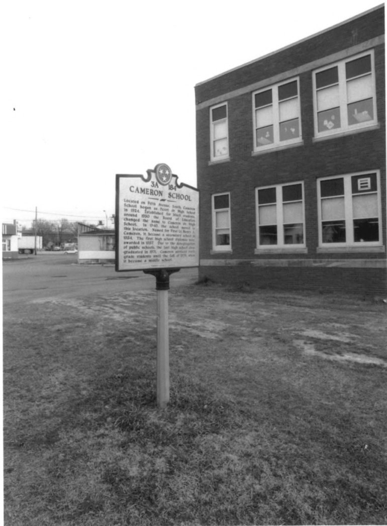
Cameron School Davidson County TN
