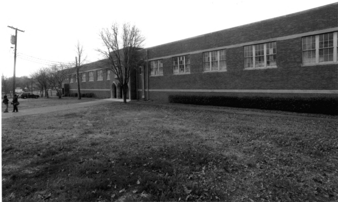
Cameron School Davidson County TN
