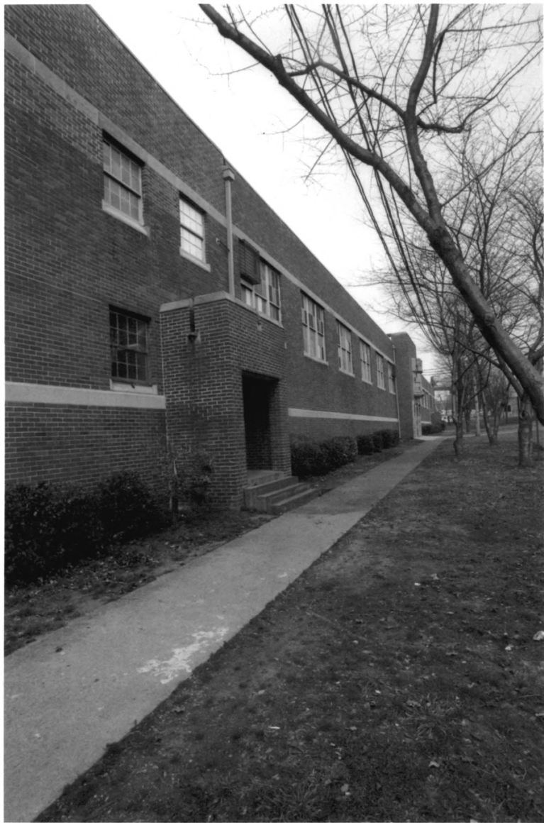
Cameron School Davidson County TN
