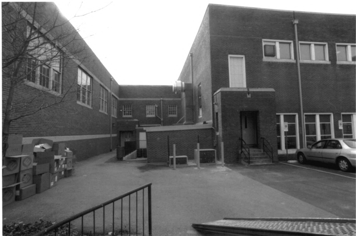
Cameron School Davidson County TN
