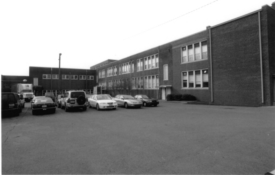
Cameron School 1 Davidson County TN
