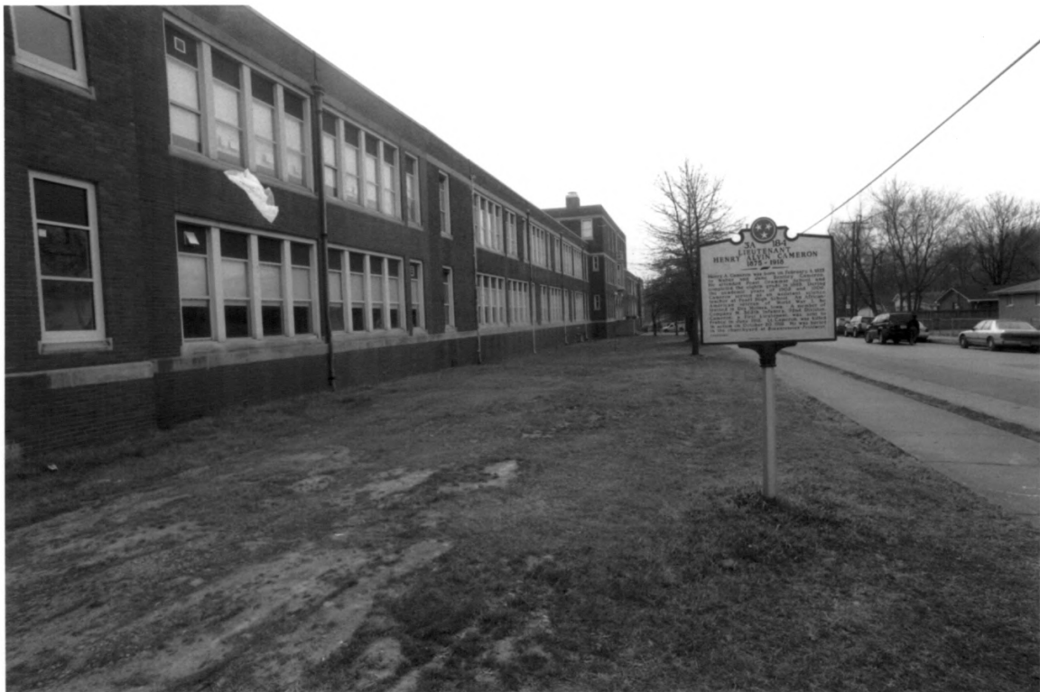
Cameron School Davidson County TN
