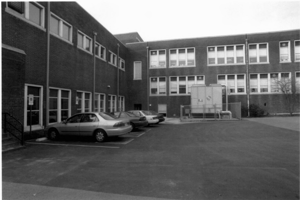
Cameron School Davidson County TN
