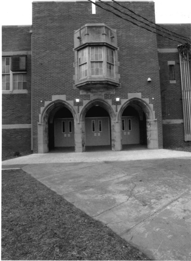
Cameron School Davidson County TN
