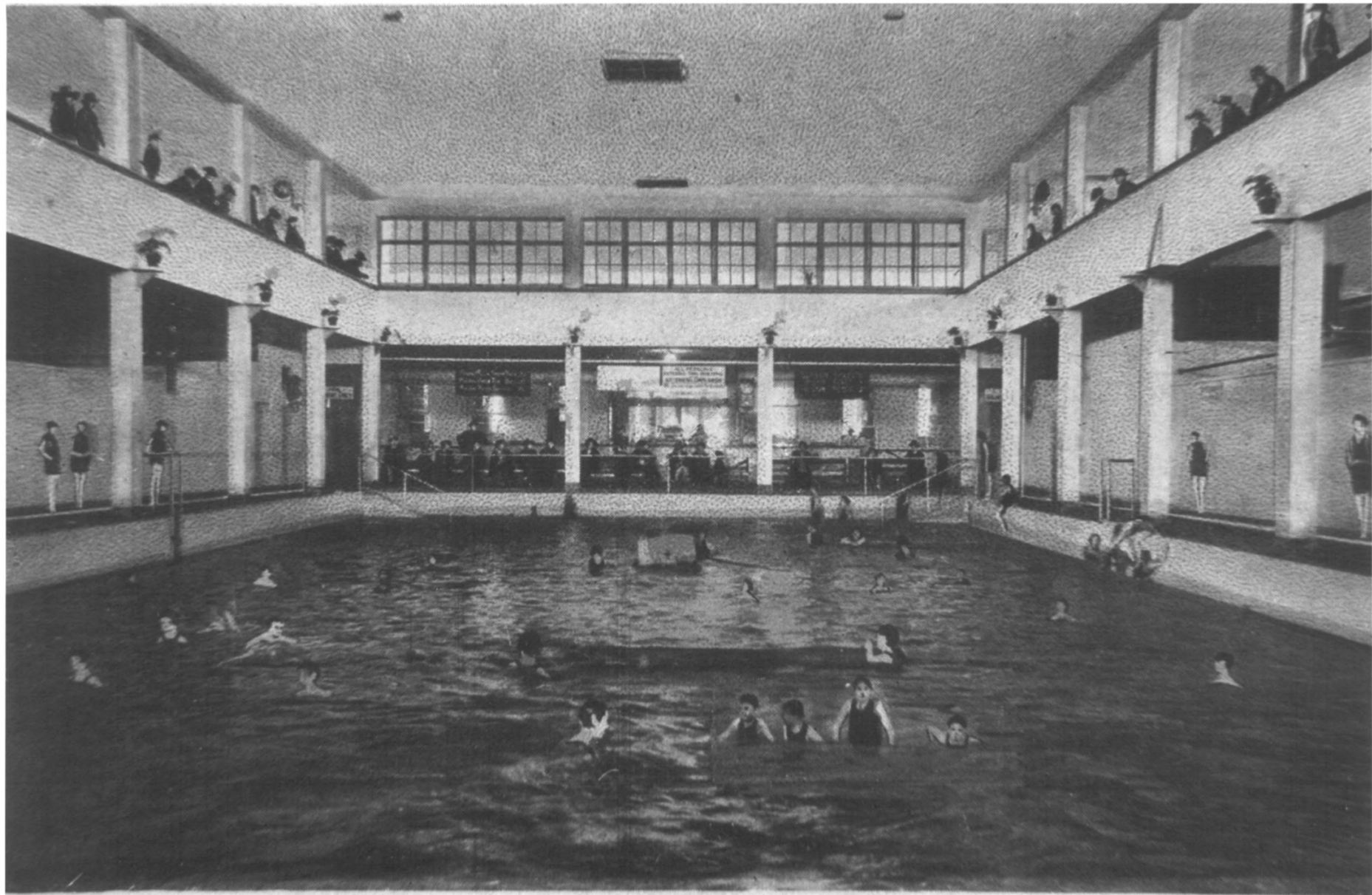
INTERIOR, MUNICIPAL NATATORIUM, BAKER, OREGON. "ON THE OLD OREGON TRAIL."
