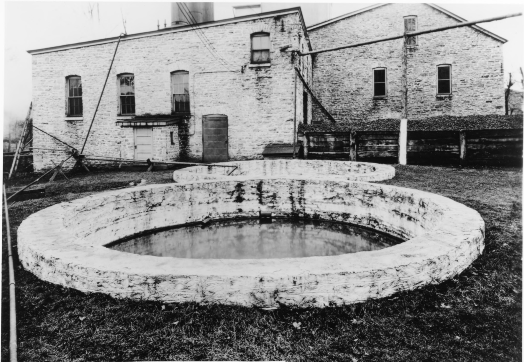
Photo 11. LABROT & GRAHAM'S OLD OSCAR PEPPER DISTILLERY Woodford County, Kentucky North elevation of renovated distillery building, coal-fired boiler, reservoirs Cusick Studio, photographer, 1935.
