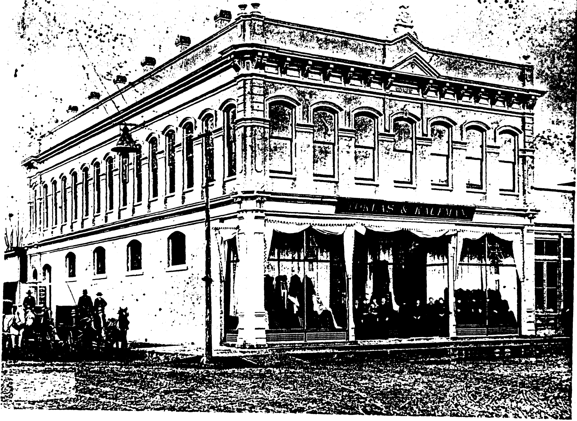
MOTTMAN BUILDING: THURSDAY COUNTY, WASHINGTON ORIGINAL (1888) OLYMPIC BLOCK / THOMAS & KAUFMAN BLDG. PRIOR TO 1911 MOTTMAN EXPANSION.
