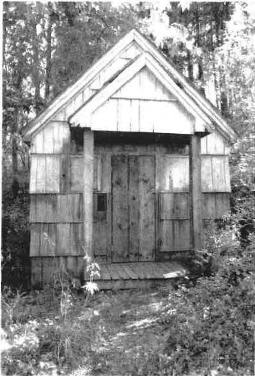
Photograph 7 of 9: Men's Restroom, front (northeast) facade.
