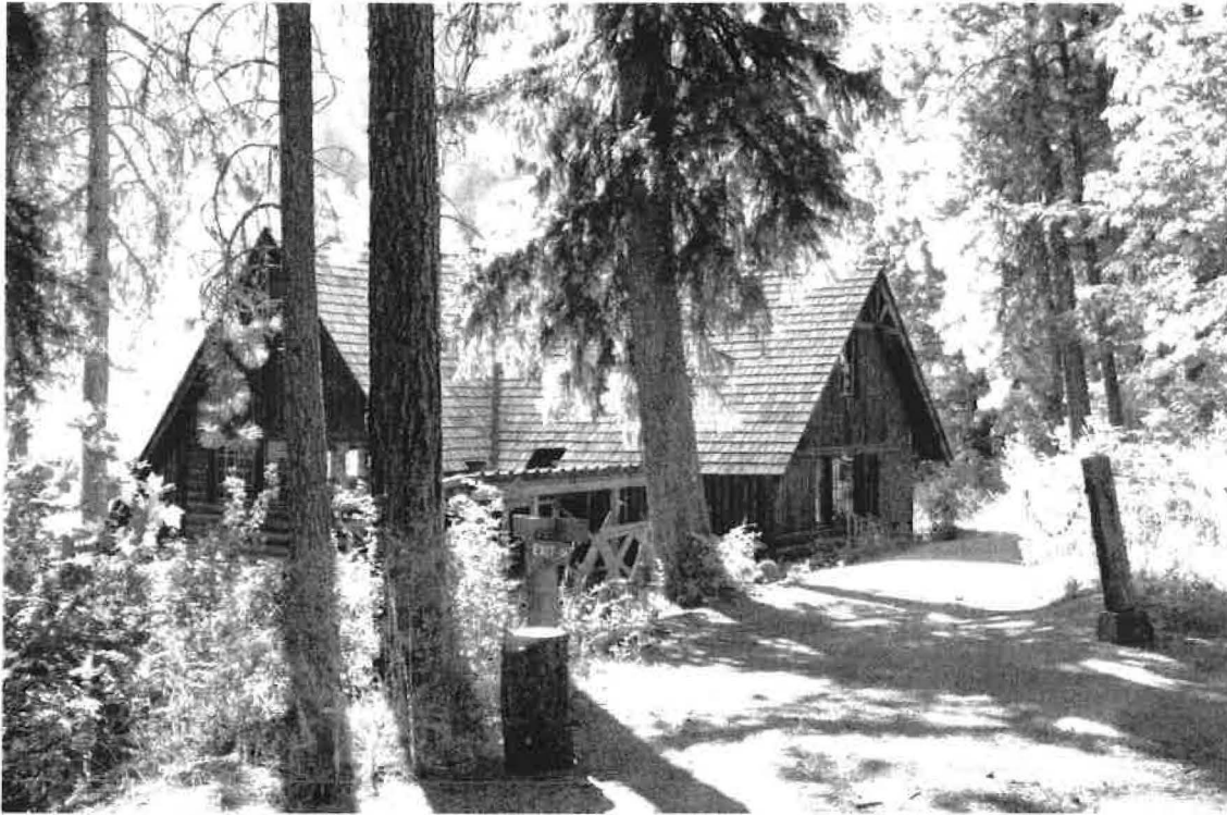
Photograph 3 of 9: East and north facades of Lodge.
