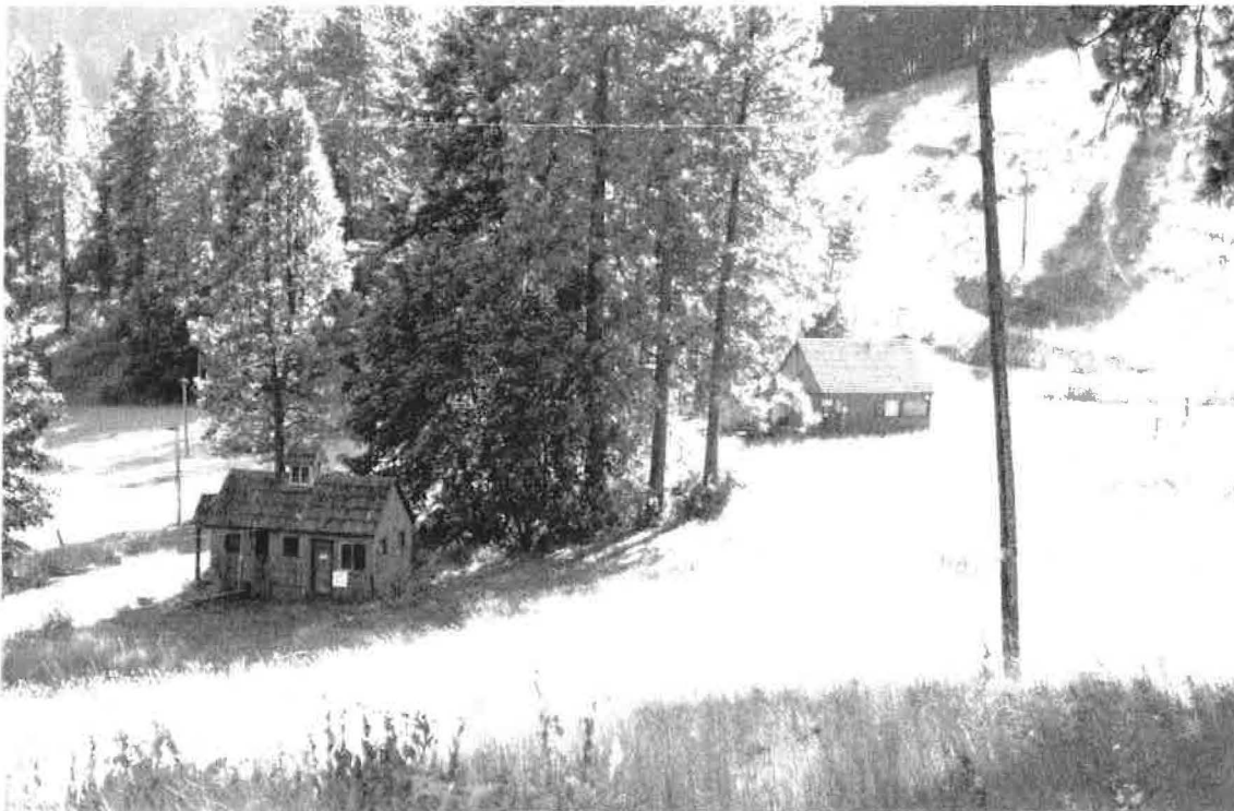
Photograph 8 of 9: Looking southwest across the site, with Women's Restroom/Rope Tow House (left) and Garage/Ticket Booth (right).
