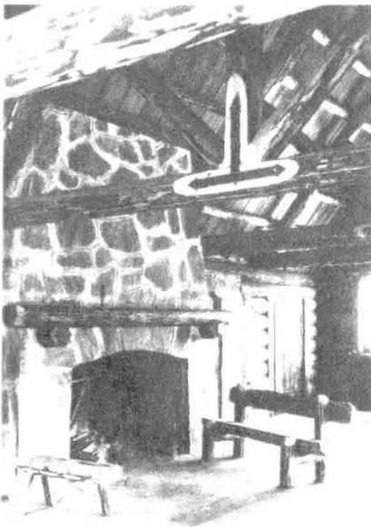
Circa 1936 view of lodge interior, looking northeast in Warming Room. Note light colored areas on logs, indicating fresh peeling and shaping work. Source: Wenatchee National Forest.
