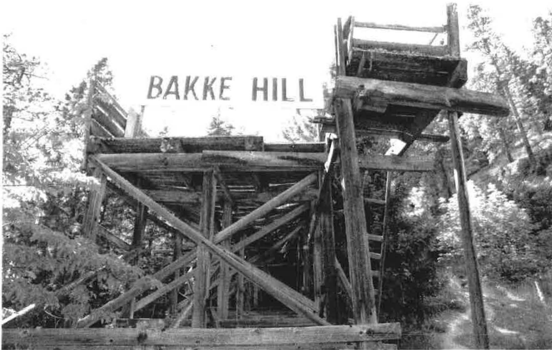
Photograph 9 of 9: Take off ramp of 90 meter ski jump, looking uphill (west).
