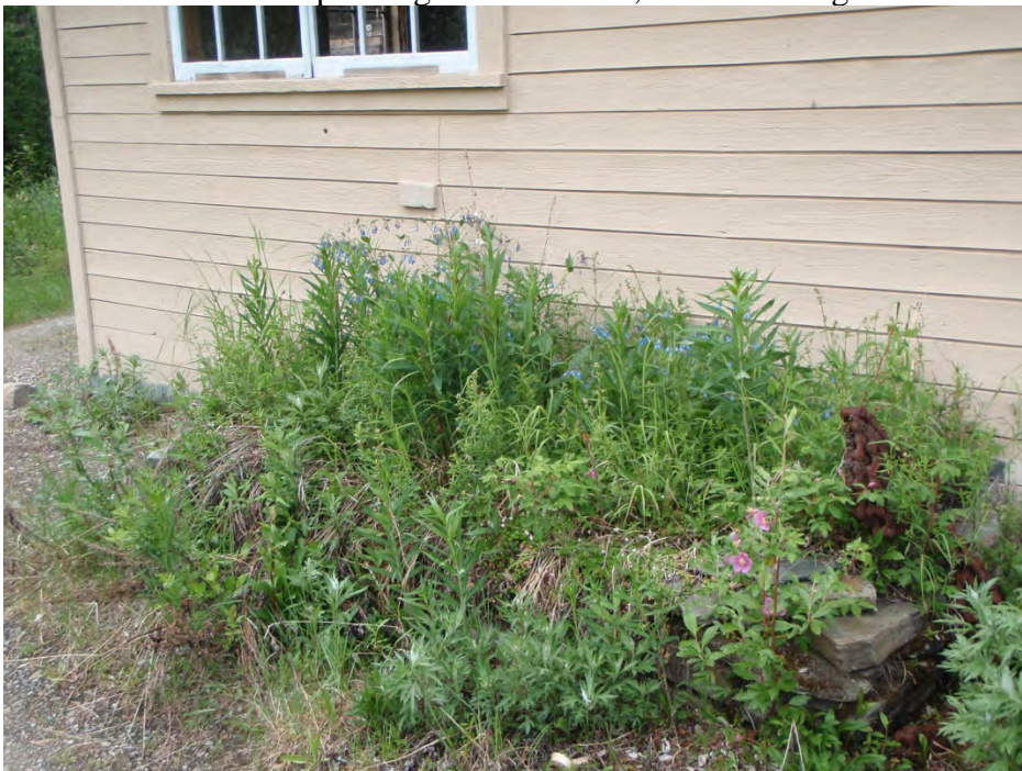
Photo #28 of 29 . (AK_Denali Borough_ Fannie Quigley Residence _0028)
