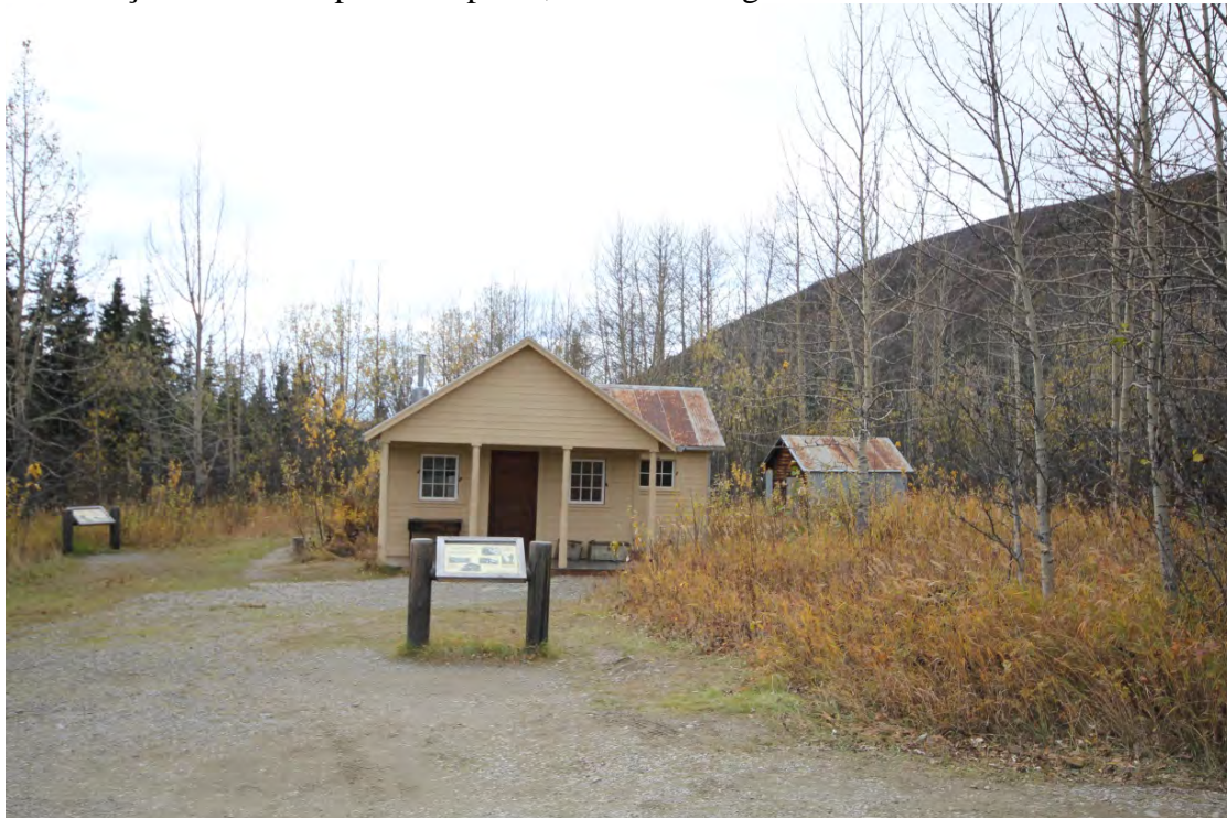
Photo #26 of 29 . (AK_Denali Borough_ Fannie Quigley Residence _0026)
