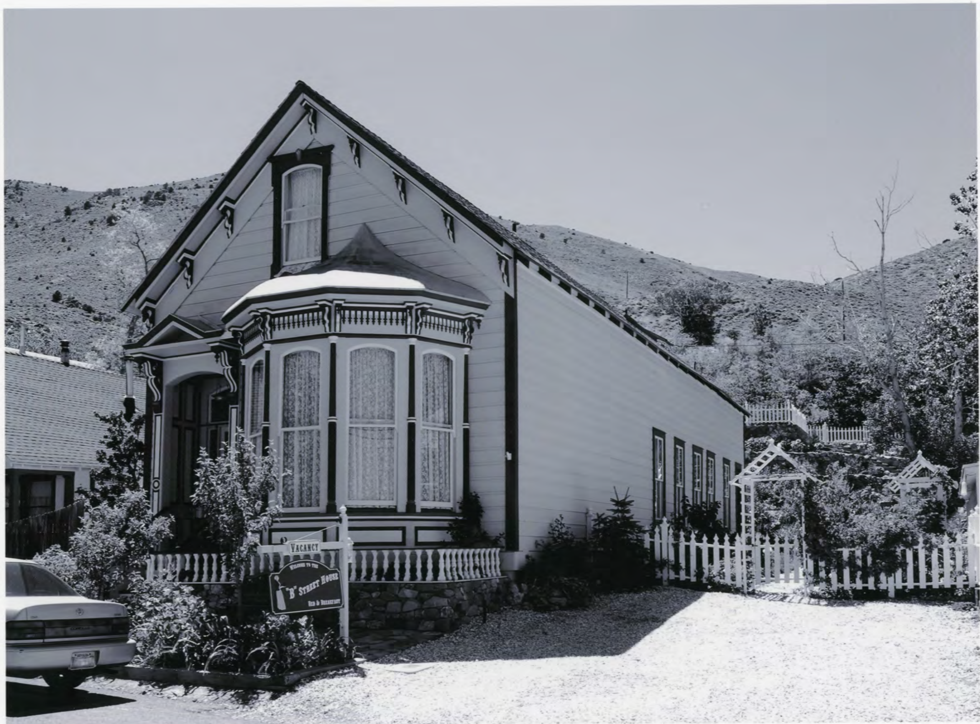
HENRY PIPER HOUSE STOREY, NV PHOTO 12
