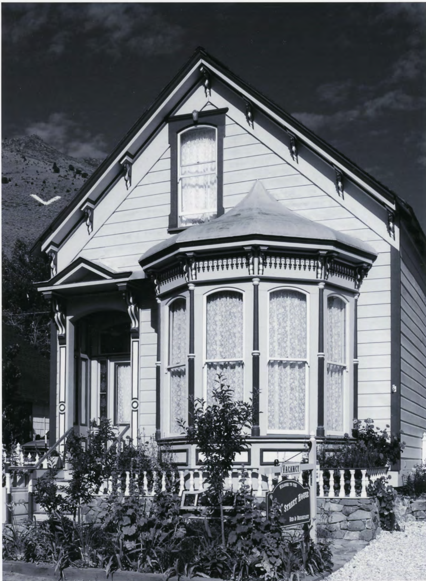
HENRY PIPER HOUSE STOREY, NV PHOTO 10
