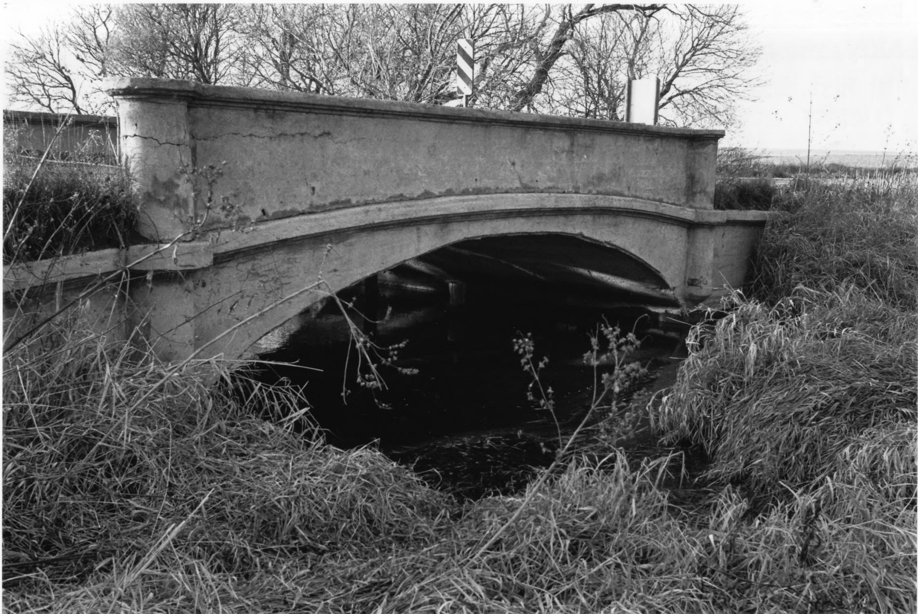
BRIDGE NO. L-2315 ROCK CO., MN PHOTO I.D. 09160#4
