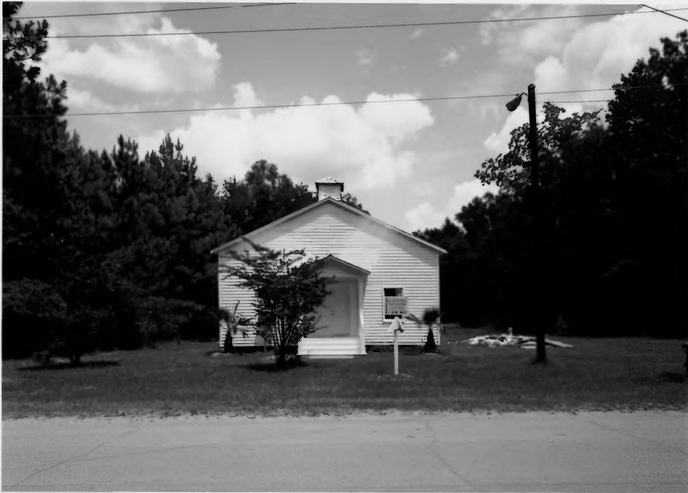
NEW OGEECHEE MISSIONARY BAPTIST CHURCH SAVANNAH, CHATHAM COUNTY, GEORGIA PHOTOGRAPH 2 OF 10
