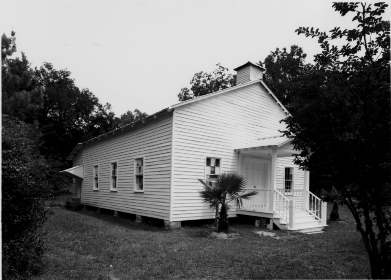
NEW OGEECHEE MISSIONARY BAPTIST CHURCH SAVANNAH, CHATHAM COUNTY, GEORGIA PHOTOGRAPH 1 OF 10
