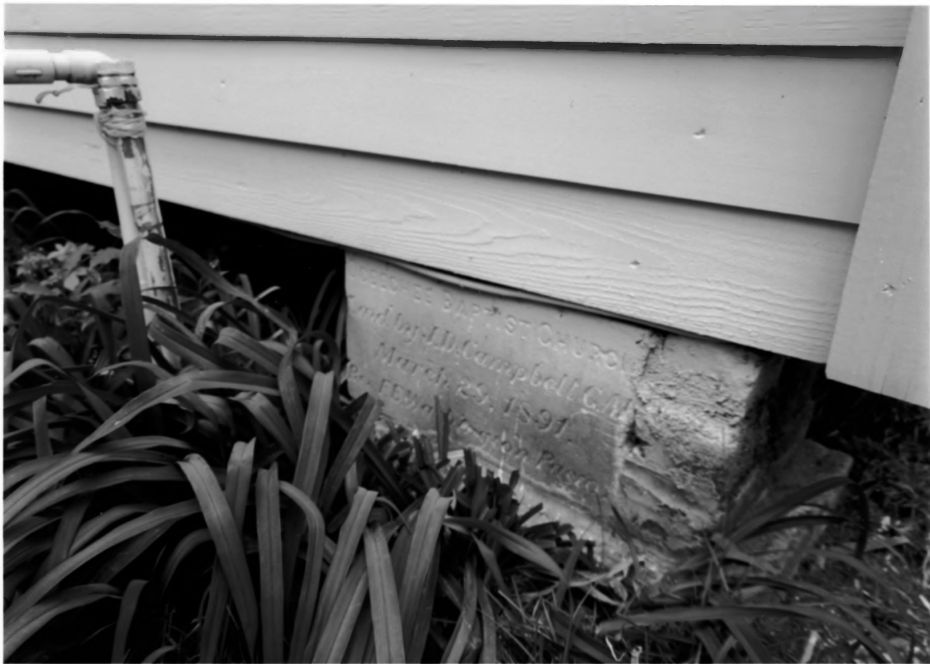
NEW OGEECHEE MISSIONARY BAPTIST CHURCH SAVANNAH, CHATHAM COUNTY, GEORGIA PHOTOGRAPH 4 OF 10
