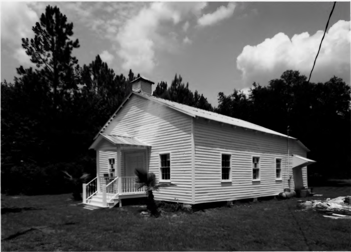
NEW OGEECHEE MISSIONARY BAPTIST CHURCH SAVANNAH, CHATHAM COUNTY, GEORGIA PHOTOGRAPH 3 OF 10
