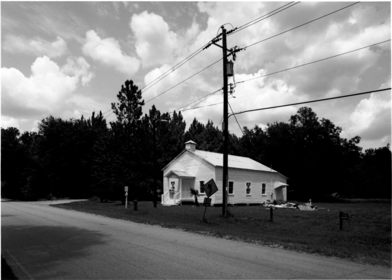
NEW OGEECHEE MISSIONARY BAPTIST CHURCH SAVANNAH, CHATHAM COUNTY, GEORGIA PHOTOGRAPH 10 OF 10
