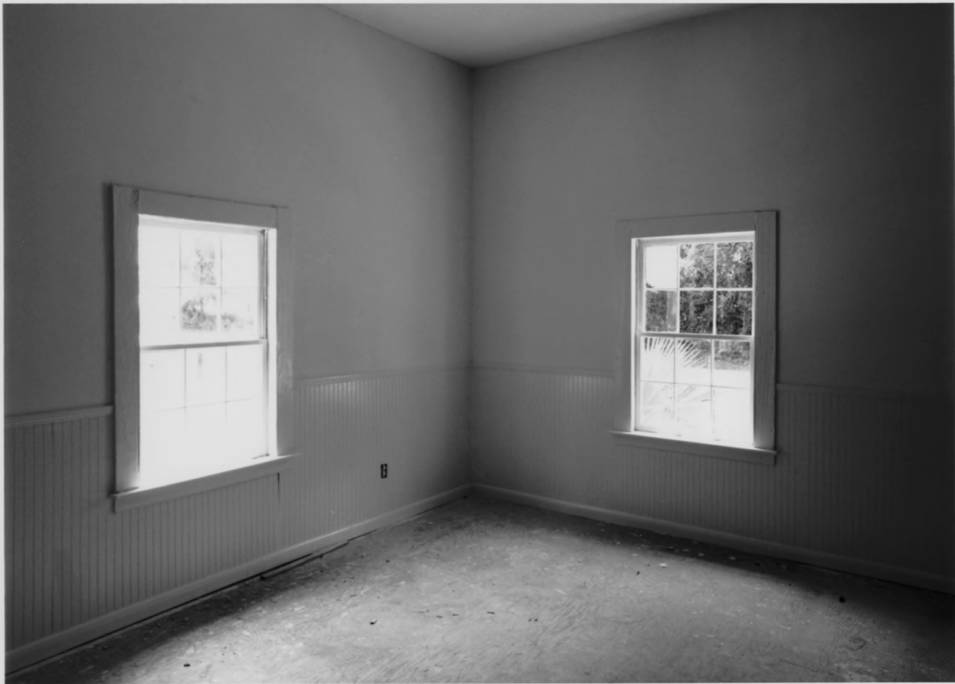
NEW OGEECHEE MISSIONARY BAPTIST CHURCH SAVANNAH, CHATHAM COUNTY, GEORGIA PHOTOGRAPH 7 OF 10
