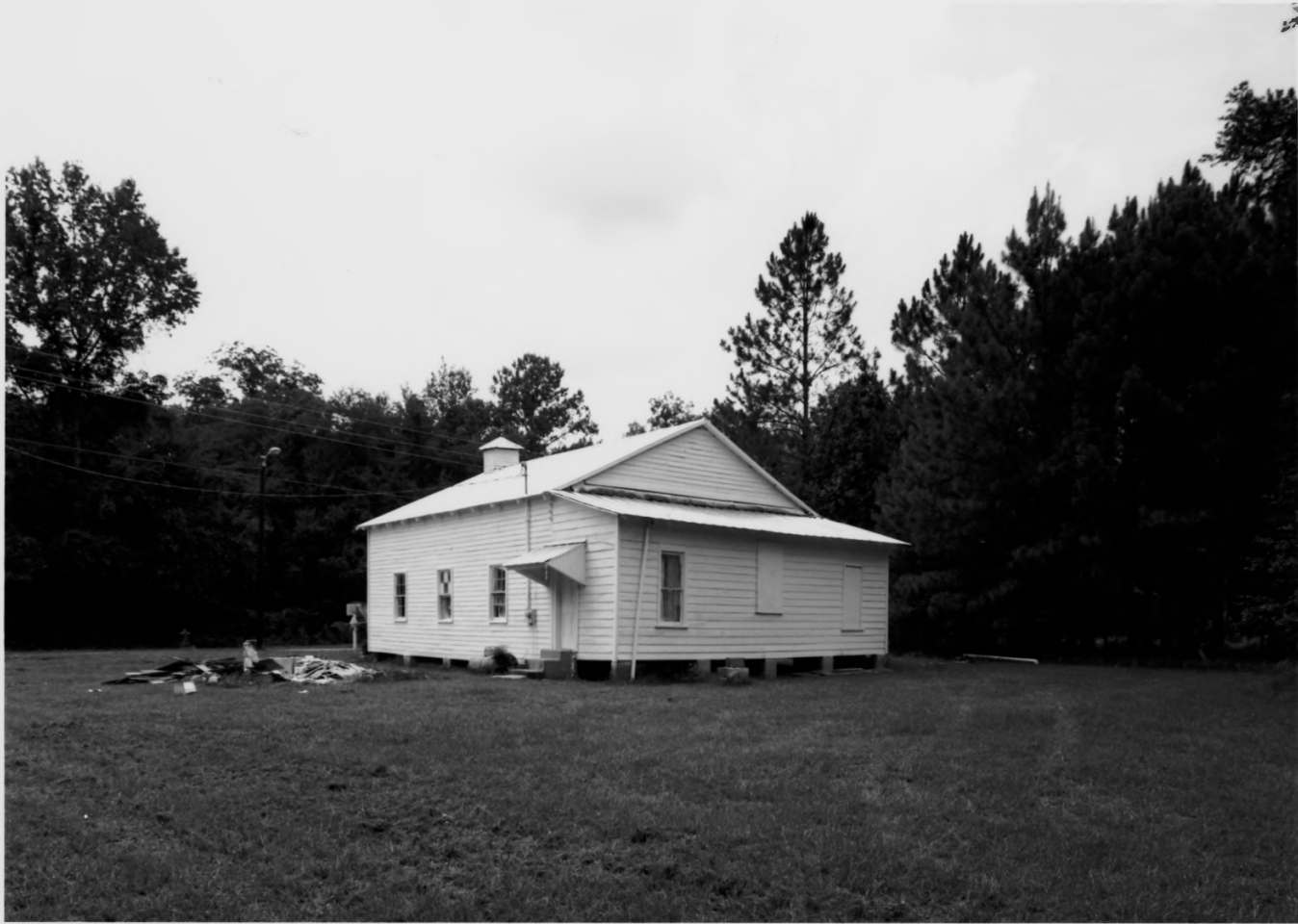
NEW OGEECHEE MISSIONARY BAPTIST CHURCH SAVANNAH, CHATHAM COUNTY, GEORGIA PHOTOGRAPH 5 OF 10
