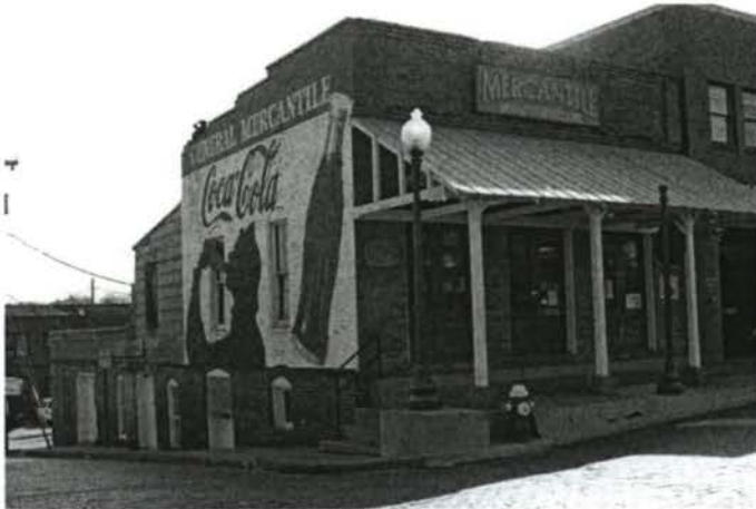
Roberts Building (1904) 216 E. Pilar Property #8 Contributing National Register (1992)
